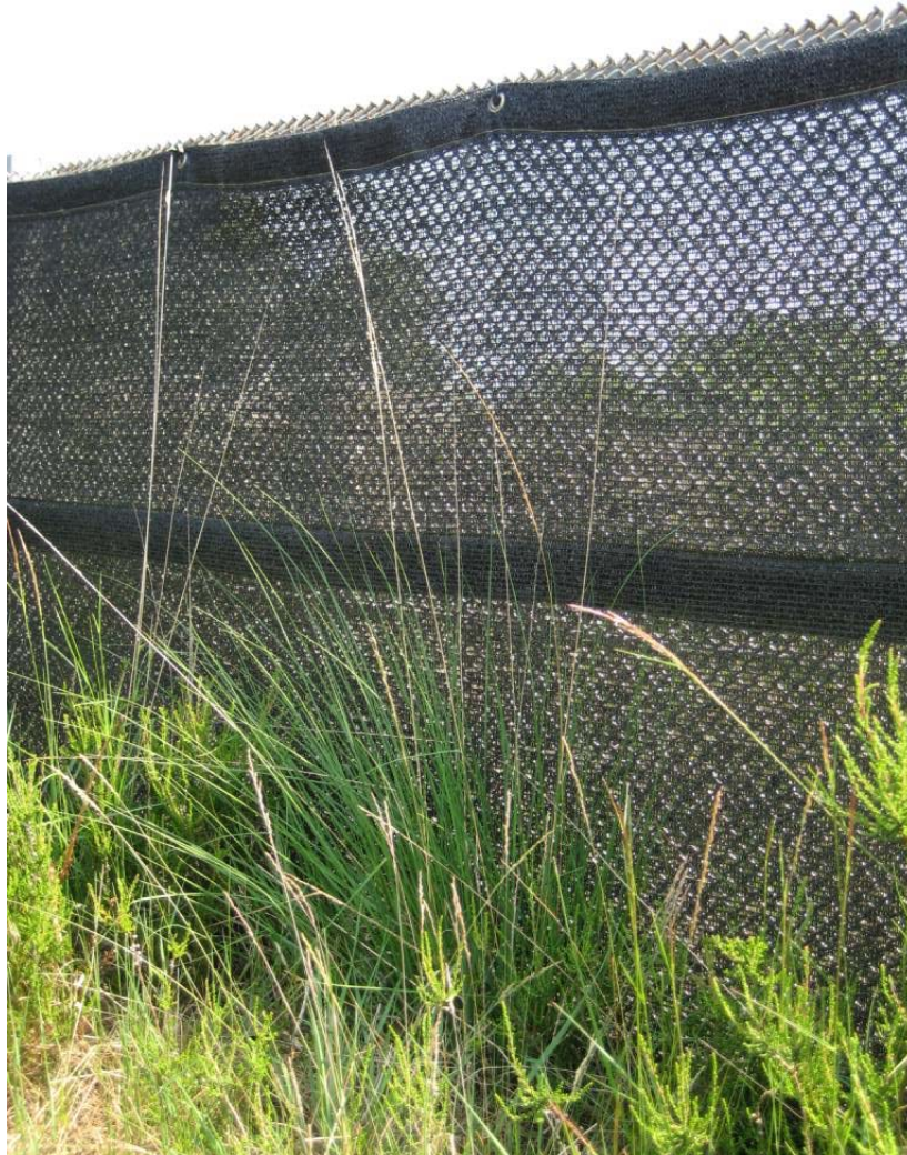
Figure 88. A row of tree stumps, grass-herb-shrub vegetation, and a road (overpass name: "Mauritskamp") on top of an overpass across the A28 motorway near the town Zeist, The Netherlands. The overpass was originally designed for a road only. Note the black screen attached to a chain link fence to reduce light disturbance from the A28 motorway (copyright: Marcel Huijser).
