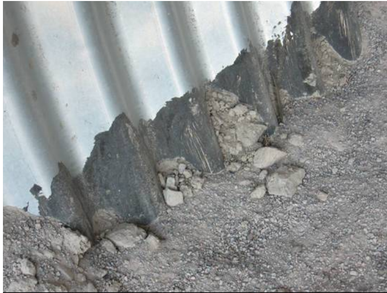
Figure 55. Soil in corrugated metal culvert makes it more suitable for use by wildlife (copyright: Marcel Huijser).
