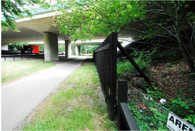
Figure 83. An underpass for a road (Hilversumsestraatweg) under the motorway A27 near the town "Hilversum", The Netherlands, that was modified with soil and tree stumps to encourage co-use by wildlife to the right of the fence. The purpose of the fence, which is painted black, is to reduce light and noise disturbance from traffic (copyright: Marcel Huijser).
