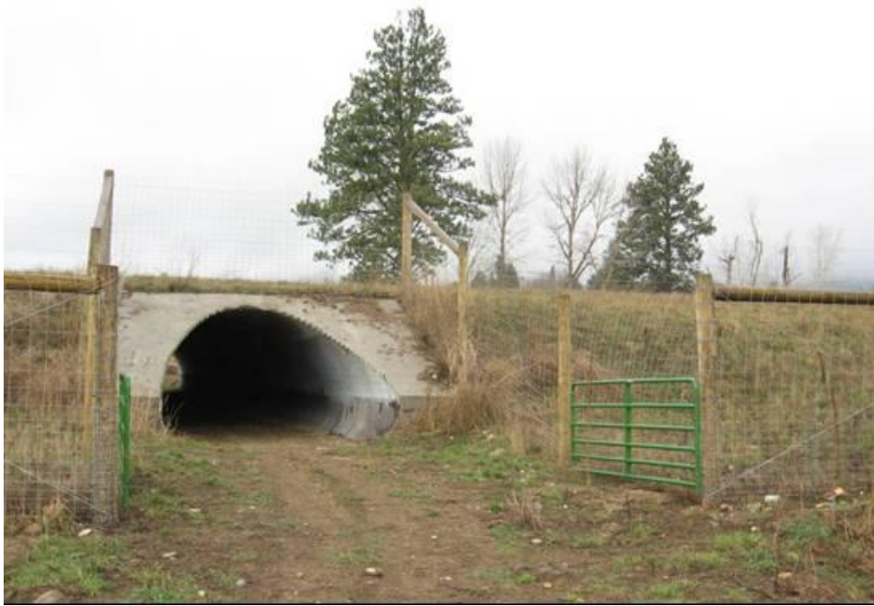
Figure 80. An underpass designed for wildlife and human access, farm machinery and livestock along U.S. Highway 93, south of Missoula, MT (copyright: Marcel Huijser).
