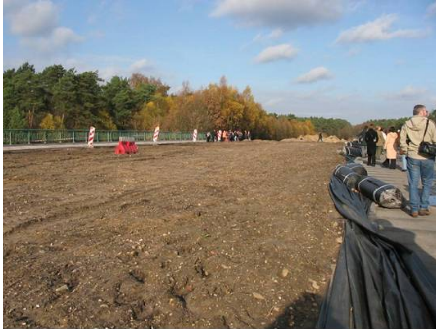
Figure 89. Road removed on bridge over motorway in Belgium and replaced with soil for vegetation and bike path (copyright: Bethanie Walder).
