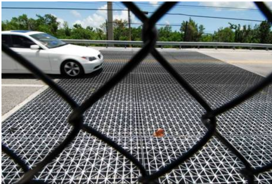
Figure 29. Wildlife guard at a fence end on the two-lane U.S. Highway 1 on Big Pine Key, FL (copyright: Marcel Huijser).
