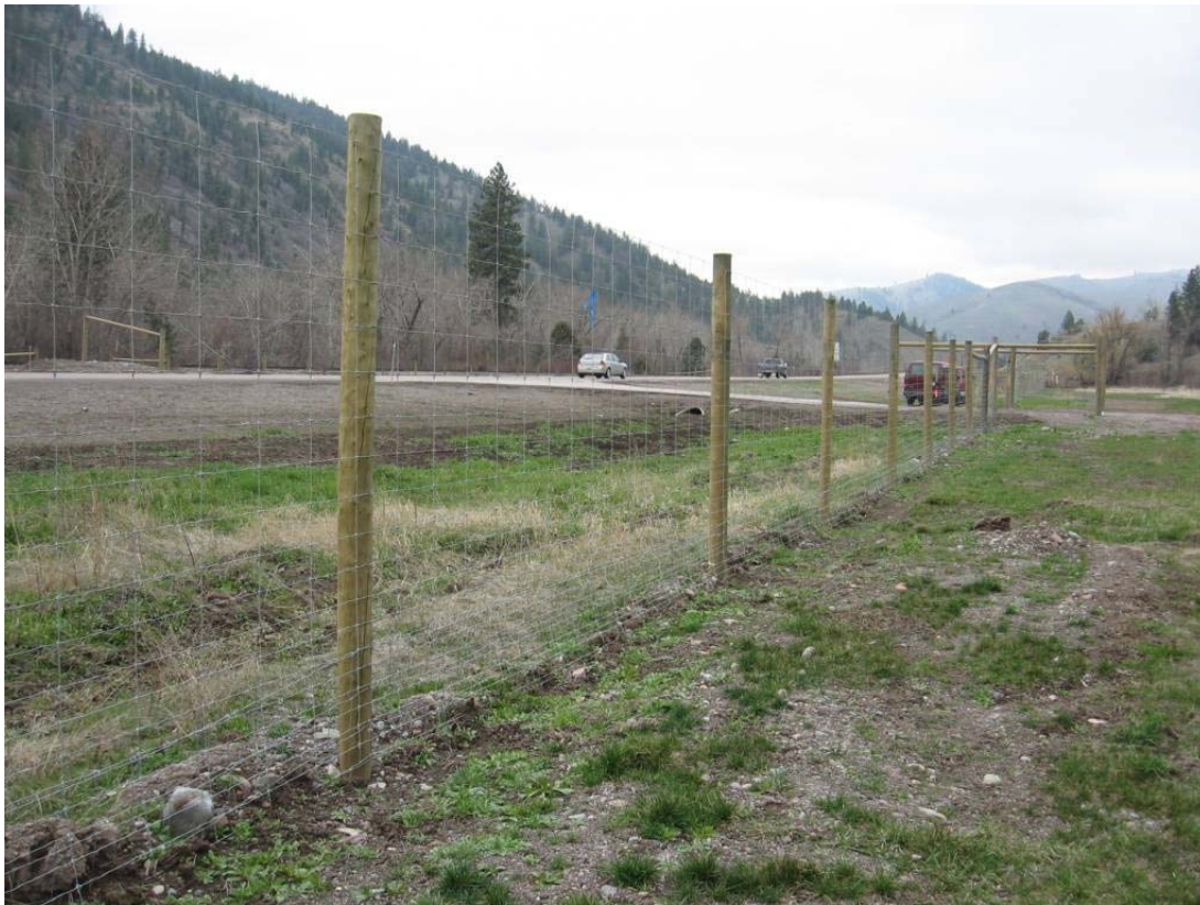
Figure 14. A 2.4-m-high (8-ft-high) large-mammal fence, with smaller mesh sizes toward the bottom, on U.S. Highway 93 on the Flathead Reservation in Montana (copyright: Marcel Huijser).
