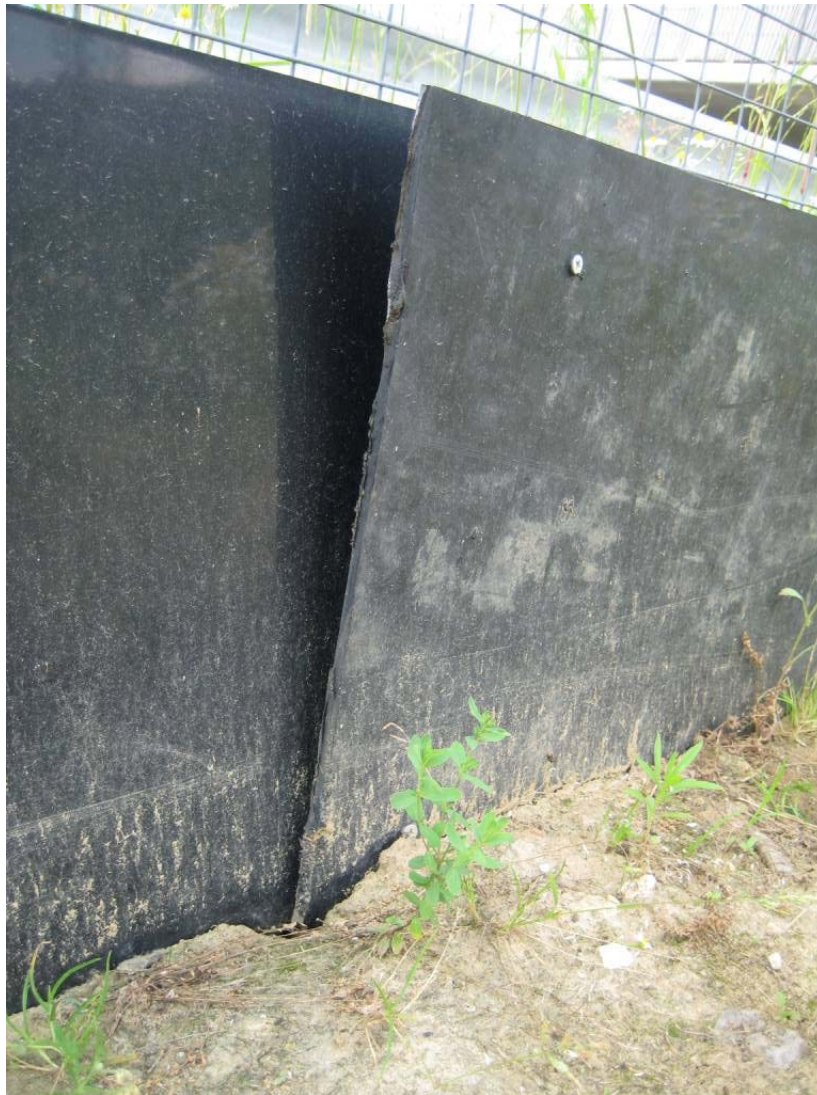
Figure 116. Plastic screens combined with a medium- and large-mammal fence guiding the animals toward an overpass (Waterloo) along the A73 motorway near the town Roermond, The Netherlands. Note that the screw that holds the two plastic sheets together is broken, allowing for a gap and potential intrusions of amphibians and other small species into the road corridor (copyright: Marcel Huijser).
