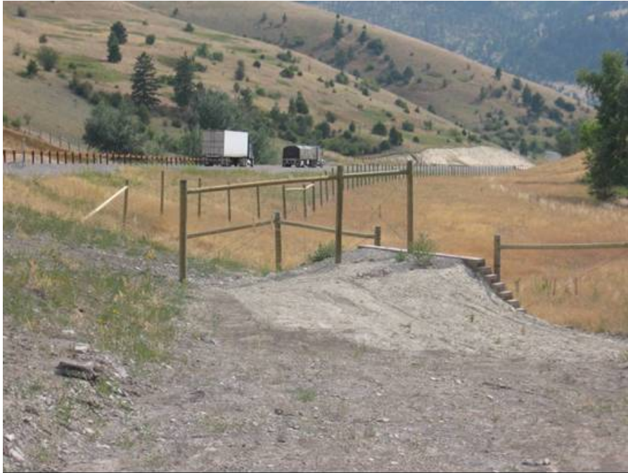
Figure 30. A short section of perpendicular fence to guide animals on top of a jump-out along a 2.4-meter-high (8-ft-high) fence along U.S. Highway 93 in Montana (copyright: Marcel Huijser).
