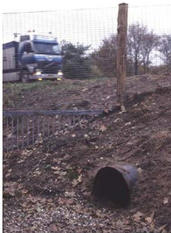
Figure 50. A small- to medium-mammal pipe (badger pipe) in The Netherlands (copyright: Marcel Huijser).
