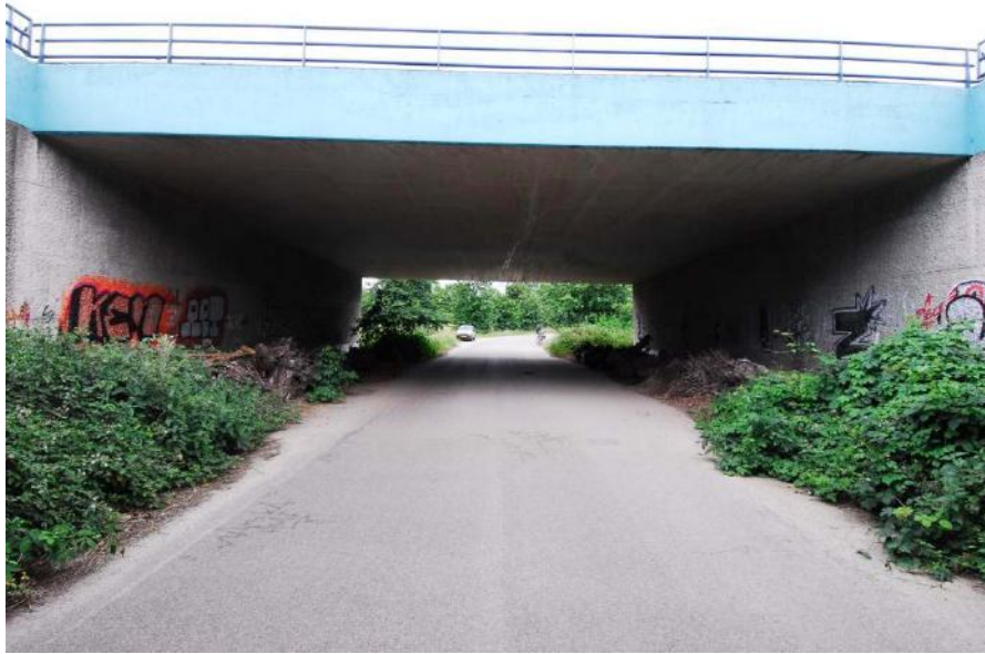
Figure 81. An underpass for a road (Lage Vuurscheweg) under the motorway A27 near the town "Hilversum", The Netherlands, that was modified with soil and tree stumps to encourage co-use by wildlife (target species included invertebrates, amphibians, reptiles, and small- and medium-sized mammals). Note that light and moisture allow for shrubs in the gap in the median (foreground) and that tree stumps provide cover under the bridge for northbound traffic (background) (copyright: Marcel Huijser).
