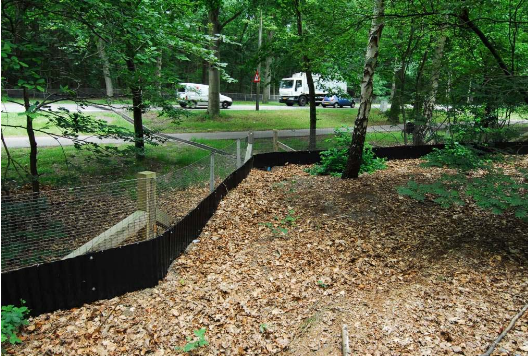
Figure 114. Plastic screens combined with a badger fence guiding the animals towards an underpass for amphibians under the road "Hilversumsestraatweg" near the town Hilversum, The Netherlands (copyright: Marcel Huijser).
