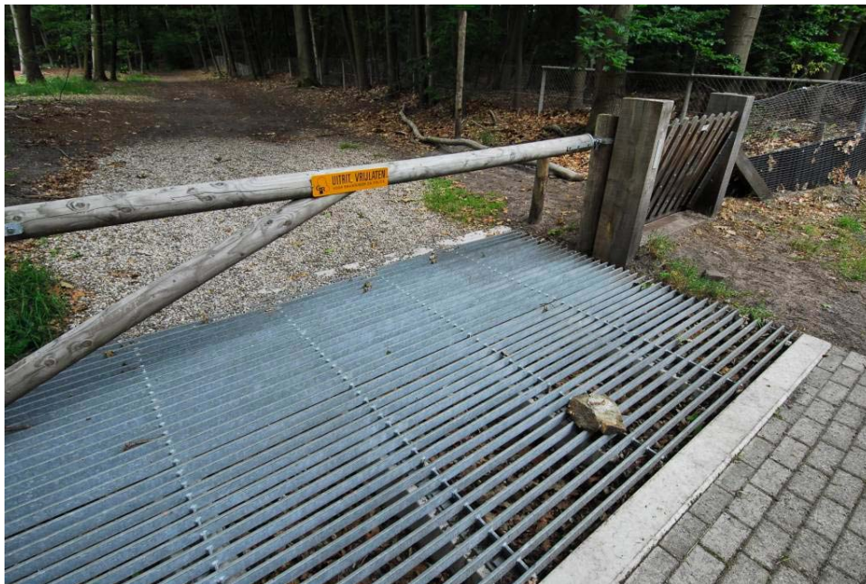
Figure 38. A wildlife guard, similar to a standard cattle guard, at a forest access road connecting to the road "Hilversumsestraatweg", near Hilversum, The Netherlands (copyright: Marcel Huijser).
