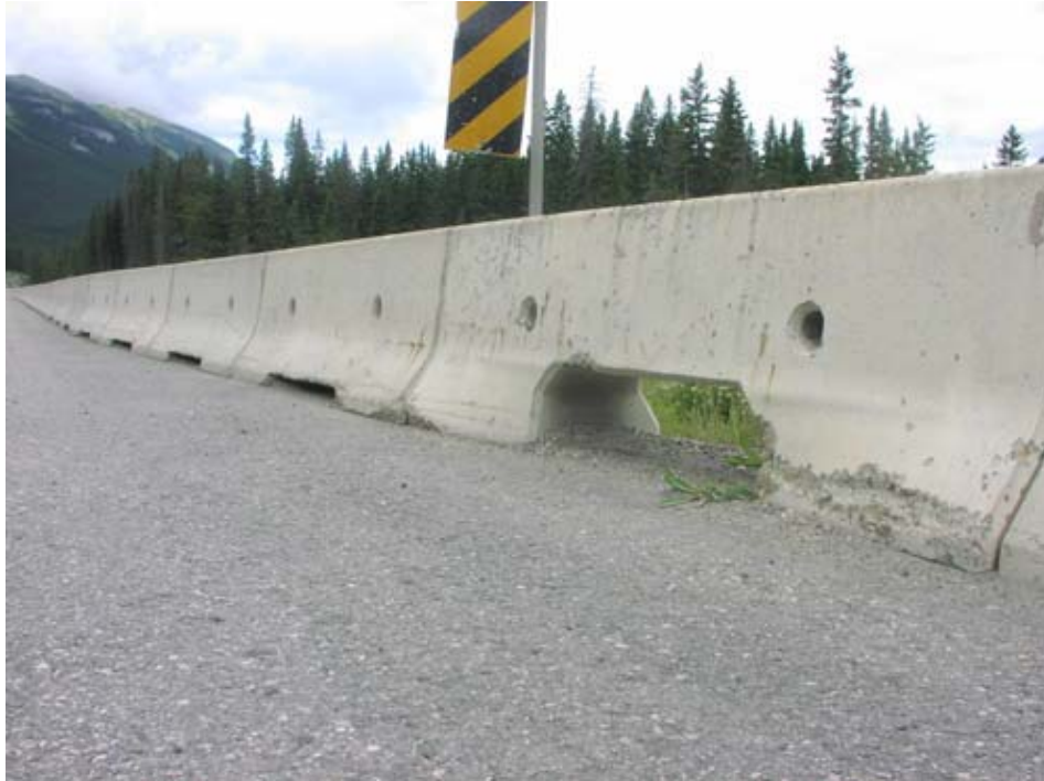
Figure 9. Concrete barriers with scuppers that allow small and mid-sized species to cross under the median barriers (copyright: A.P. Clevenger).
