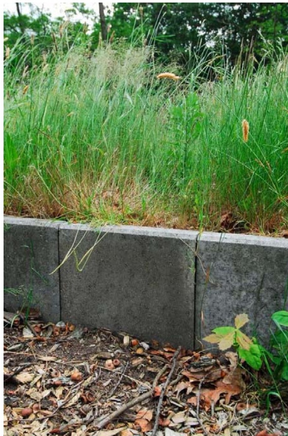
Figure 111. Concrete barrier leads amphibians toward an underpass along the road "Hilversumsestraatweg" near the town Hilversum, The Netherlands (copyright: Marcel Huijser).
