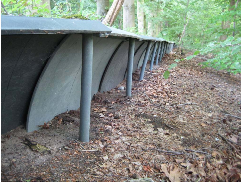
Figure 112. Plastic sheets that guide amphibians to an underpass, near the town Hilversum, The Netherlands (copyright: Marcel Huijser).
