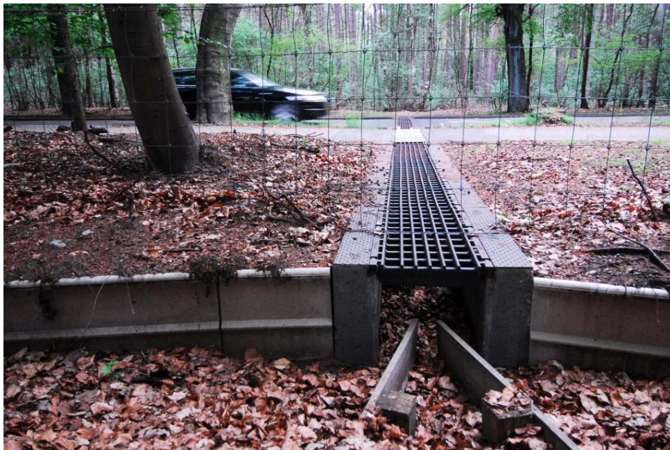
Figure 115. Concrete barrier and planks guiding amphibians toward an underpass under the road "Bussumergrindweg", near the town Hilversum, The Netherlands (copyright: Marcel Huijser).
