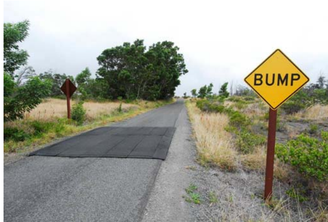
Figure 134. Speed bump, specifically installed to reduce vehicle speed for nearby breeding, roosting and feeding area for the Hawaiian goose in Volcanoes National Park, HI (copyright: Marcel Huijser).
