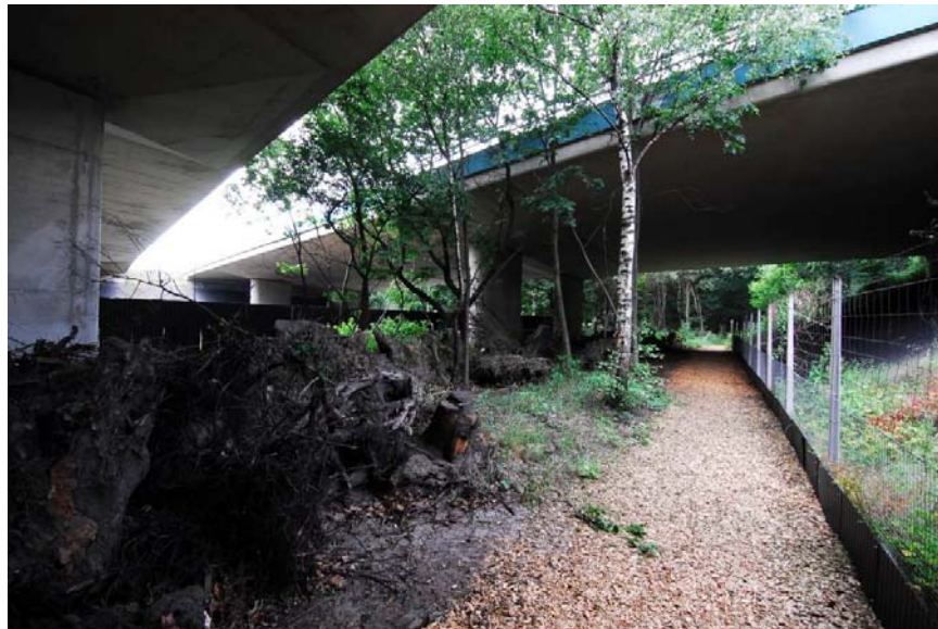
Figure 82. An underpass for a road (Hilversumsestraatweg) under the motorway A27 near the town "Hilversum", The Netherlands, that was modified with soil and tree stumps to encourage co-use by wildlife. Note that light and moisture allow for shrubs and trees in the gap in the median (background) and that tree stumps provide cover under the bridge for northbound traffic (foreground) (copyright: Marcel Huijser).
