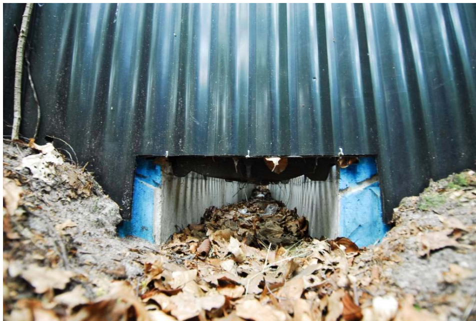
Figure 123. Close-up of an underpass for amphibians along the road "Hilversumsestraatweg" near the town Hilversum, The Netherlands. Note that the open roof allows light, air, and moisture to enter the underpass (copyright: Marcel Huijser).
