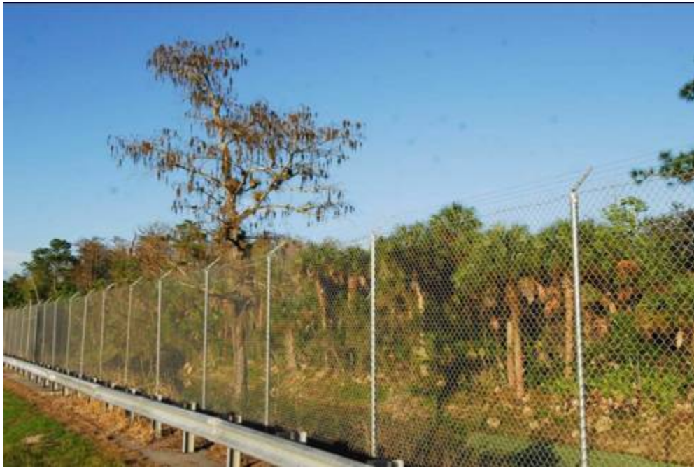
Figure 16. A 3.4-m-high (11-ft-high) chain-link fence along SR 29 in southern Florida, designed to keep Florida panthers off the roadway and to guide them toward underpasses. Note the outriggers pointing away from the road (copyright: Marcel Huijser).
