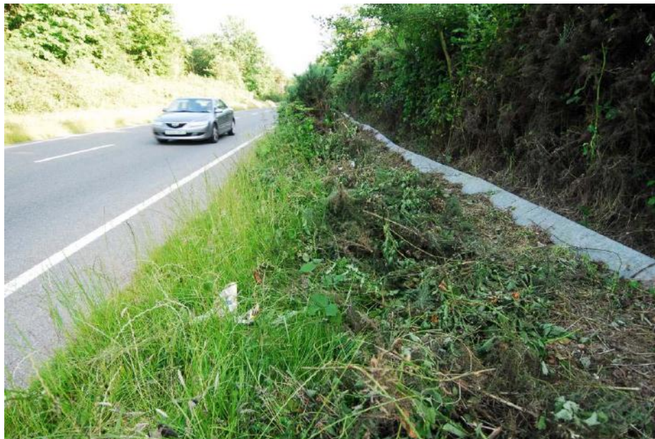
Figure 119. The vegetation on both sides of a concrete barrier for amphibians was mowed to prevent small species from using the vegetation to climb the barrier and enter the road corridor, near the town Haywards Heath, West Sussex, England (copyright: Marcel Huijser).
