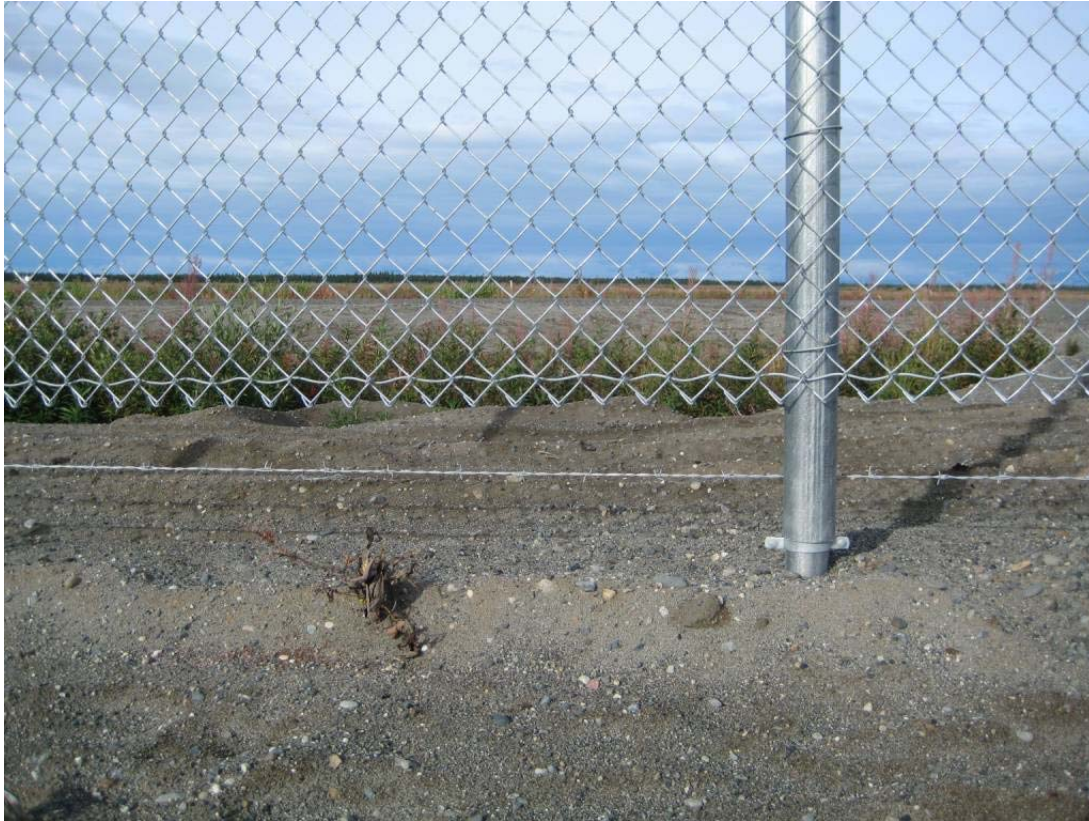
Figure 24. A chain-link moose fence near Kenai, AK, with a gap (and a barbed wire strand) at the bottom allowing small species to crawl underneath the fence (copyright: Marcel Huijser).
