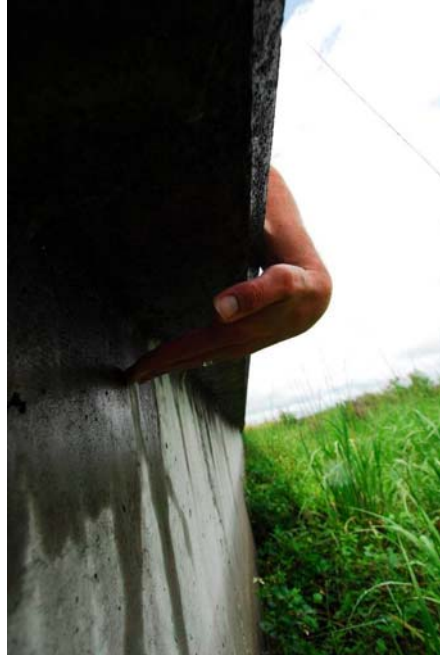
Figure 126. A closeup of the concrete barrier for amphibians and reptiles along U.S. Highway 441 through Paynes Prairie, south of Gainesville, FL (copyright: Marcel Huijser).
