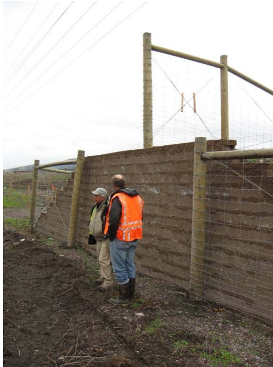
Figure 31. A jump-out along a 2.4-meter-high (8-ft-high) fence along U.S. Highway 93 in Montana (copyright: Marcel Huijser).
