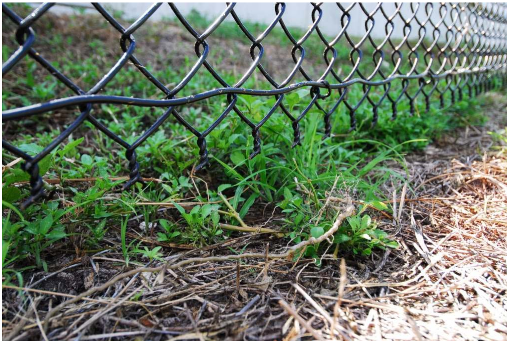
Figure 23. A 1.83-meter-high (6-ft-high) chain-link fence along U.S. Highway 1 on Big Pine Key, FL, with a 10-cm (4-in) gap allowing the endangered Lower Keys marsh rabbit access to the right of way (copyright: Marcel Huijser).
