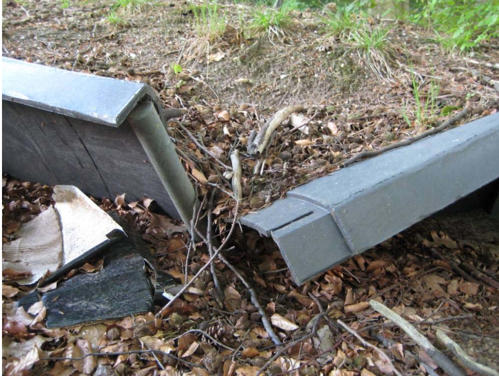
Figure 118. Plastic screens that collapsed were intended to guide amphibians toward an underpass near the town Hilversum, The Netherlands. The gap allows amphibians and other small species to enter the road corridor (copyright: Marcel Huijser).
