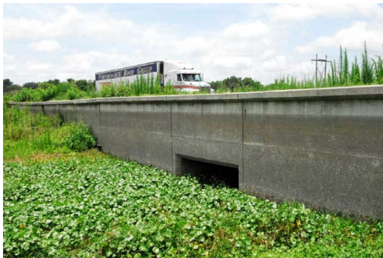
Figure 125. A concrete barrier combined with an underpass for amphibians and reptiles along U.S. Highway 441 through Paynes Prairie, south of Gainesville, FL (copyright: Marcel Huijser).
