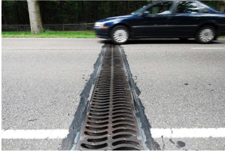
Figure 122. The open metal top of an underpass for amphibians, allowing light, air, and moisture to enter, under the road "Hilversumsestraatweg" near the town Hilversum, The Netherlands (copyright: Marcel Huijser).
