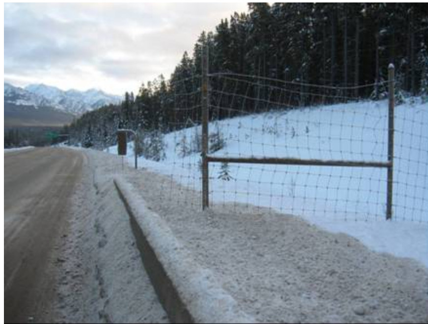
Figure 27. Fence end brought close to the road with a concrete barrier for safety in Banff National Park, just west of Castle Junction, Alberta (copyright: Marcel Huijser).
