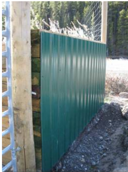
Figure 33. A jump-out along a 2.4-meter-high (8-ft-high) fence with smooth metal to prevent bears from climbing into the right of way along the Trans-Canada Highway, Banff National Park, Alberta (copyright: Marcel Huijser).
