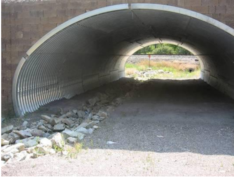
Figure 73. Wildlife underpass (large-mammal culvert) along U.S. Highway 93 in Montana with a ditch that allows water to flow (seasonally) (copyright: Marcel Huijser).
