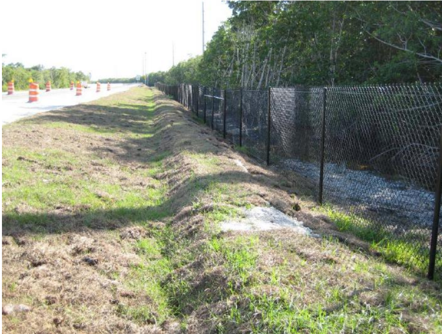
Figure 103. A 1.83-m-high (6-ft-high) chain-link wildlife fence intended for American crocodile along U.S. Highway 1 between Florida City and Key Largo, FL (copyright: Marcel Huijser).
