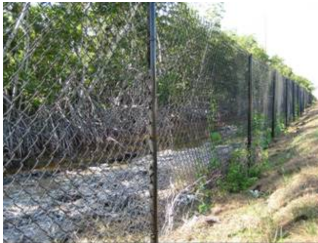
Figure 35. A 1.83-meter-high (6-ft-high) chain-link fence along U.S. Highway 1 between Florida City and Key Largo, FL, has been coated with colored plastic (copyright: Marcel Huijser).
