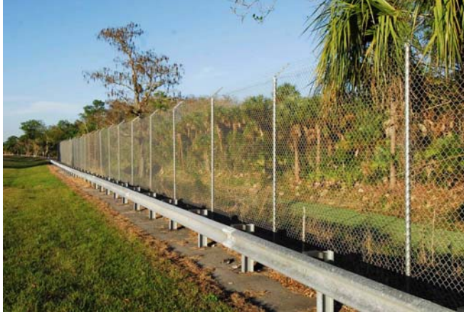
Figure 151. Wildlife fencing, with barbed wire overhang, for the Florida panther on SR 29 in southern Florida (copyright: Marcel Huijser).
