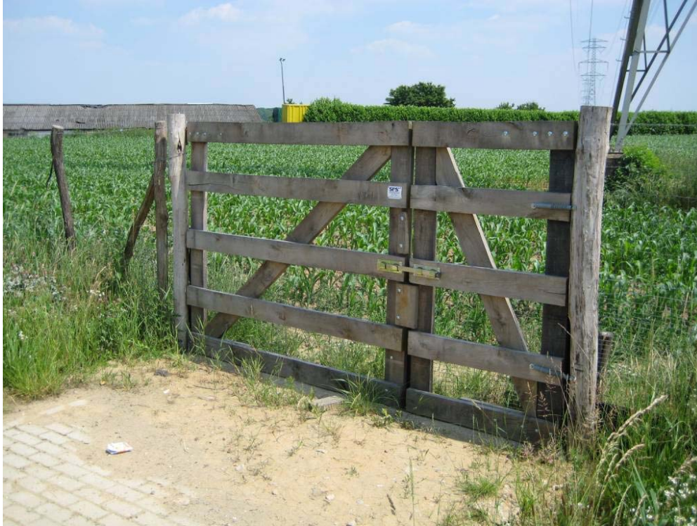
Figure 127. A gate that allows for access to a field with crops through an amphibian barrier, and a medium- and large-mammal fence, near wildlife overpass "Schinheuveld," near the town Roermond, The Netherlands. Note that the gate connects closely to a hard surface to prevent amphibians and other small species from entering the road corridor. (copyright: Marcel Huijser).
