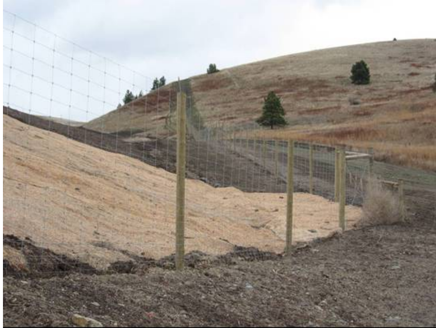
Figure 57. After construction, straw mats were used to protect slopes from erosion and rapid establishment of weeds along U.S. Highway 93 in Montana (copyright: Marcel Huijser).
