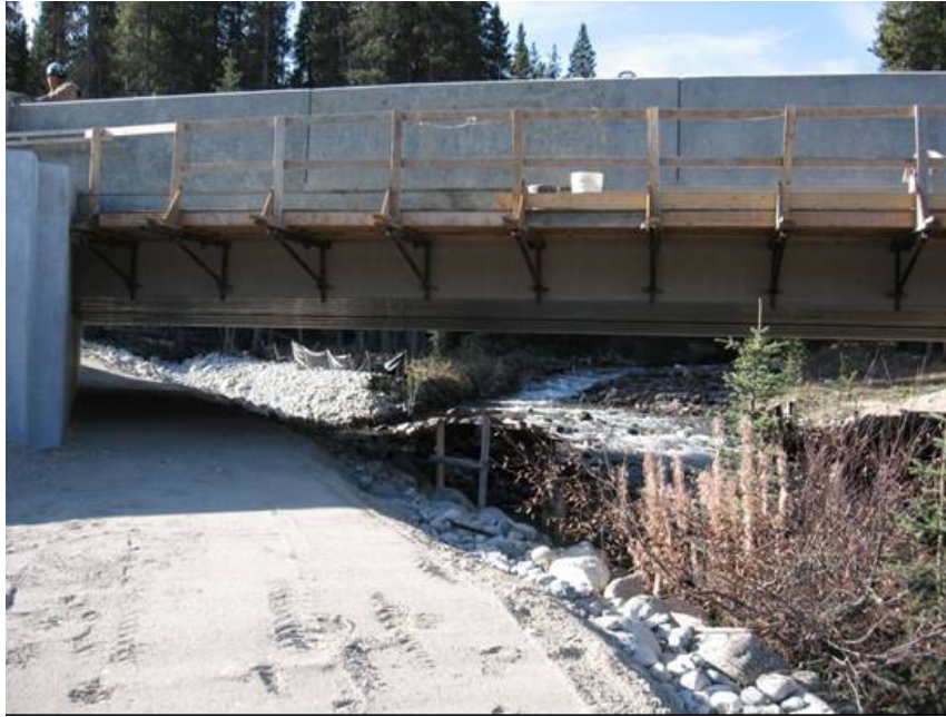
Figure 76. Over-span bridge across a stream, with a bank and walkway for terrestrial large-mammal species along the Trans-Canada Highway, Banff National Park, Alberta (copyright: Marcel Huijser).
