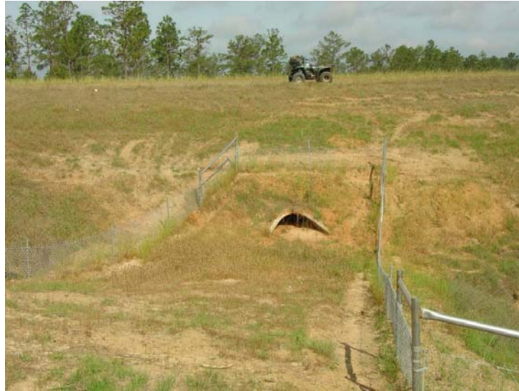
Figure 109. Fences lead gopher tortoises toward a culvert along Highway 63 in Green County, south of Leakesville, MS (copyright: Chuck Walters).
