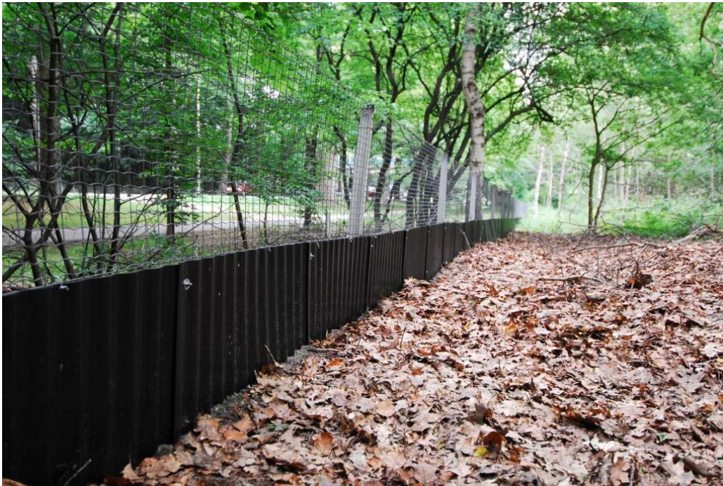
Figure 113. Plastic screens combined with a badger fence along the road "Hilversumsestraatweg" near the town Hilversum, The Netherlands (copyright: Marcel Huijser).
