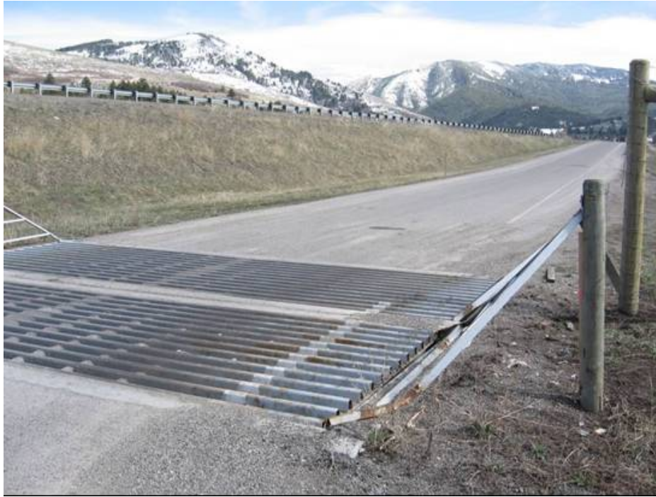
Figure 37. A wildlife guard, similar to a standard cattle guard, at an on-ramp to Interstate 90 east of Bozeman, MT (copyright: Marcel Huijser).
