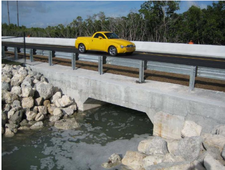
Figure 104. An underpass for American crocodiles along U.S. Highway 1 between Florida City and Key Largo, FL (copyright: Marcel Huijser).
