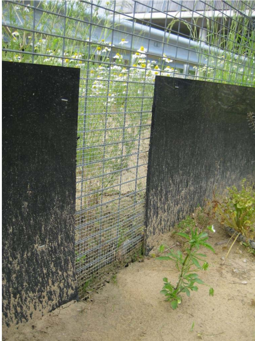
Figure 117. Plastic screens combined with a medium- and large-mammal fence guiding the animals toward an overpass (Waterloo) along the A73 motorway near the town Roermond, The Netherlands. Note that two adjacent sheets have a gap that is covered by fine mesh wire fence to prevent amphibians and other small species from entering the road corridor (copyright: Marcel Huijser).
