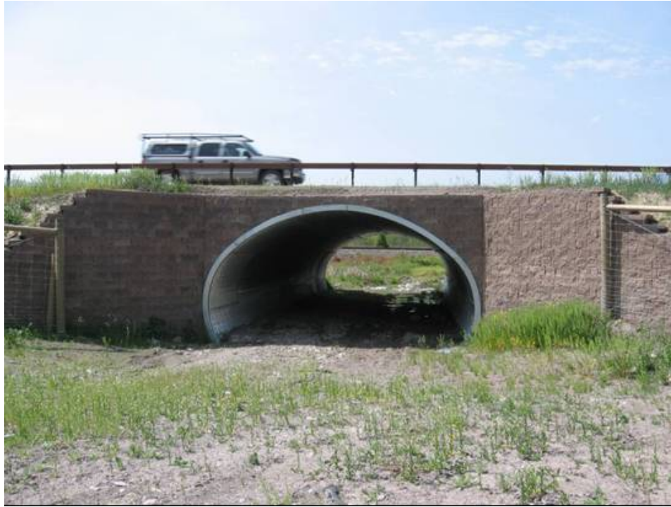
Figure 52. Wildlife fencing ties in with the underpass wing walls, preventing animals from entering the road corridor (copyright: Marcel Huijser).
