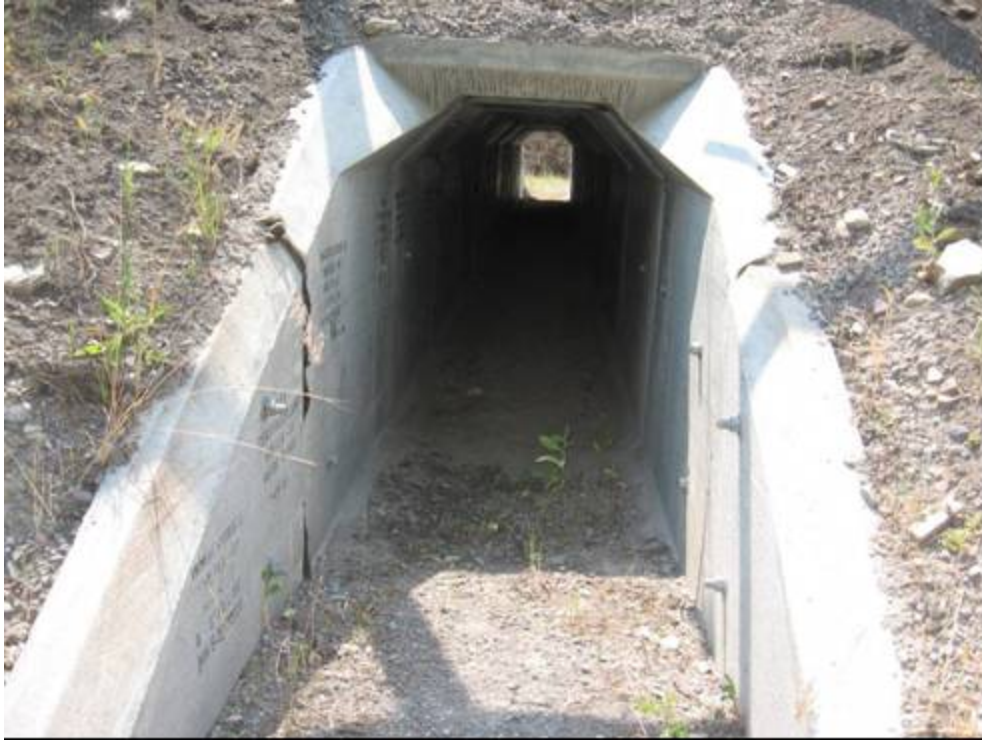
Figure 48. A medium-mammal box culvert (1.2 m (3.9 ft) wide, 1.8 m (5.9 ft) high) along U.S. Highway 93, south of Ravalli, MT (copyright: Marcel Huijser).
