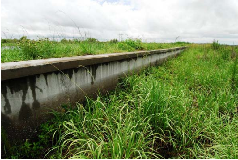
Figure 124. A concrete barrier for amphibians and reptiles along U.S. Highway 441 through Paynes Prairie, south of Gainesville, FL (copyright: Marcel Huijser).
