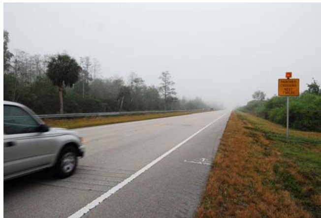
Figure 150. Permanently flashing warning sign for Florida panther, combined with a rumble strip along SR 29 in southern Florida (copyright: Marcel Huijser).
