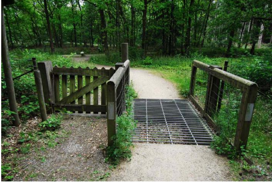
Figure 43. A swing gate for pedestrians and a wildlife guard at a bicycle path into an enclosure with large mammals (cattle), near the town "De Lage Vuursche", The Netherlands (copyright: Marcel Huijser).
