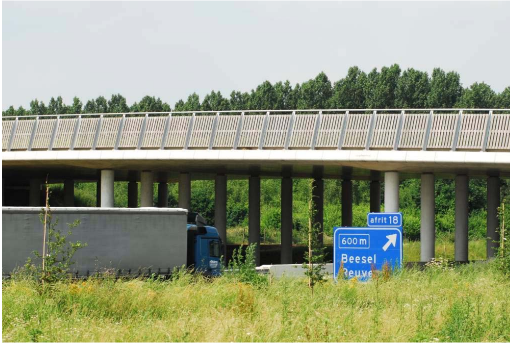
Figure 62. The wildlife overpass "Waterloo" with wildlife fencing across the A73 motorway near the town "Roermond", The Netherlands, consists of planks that also act as a light and sound barrier (copyright: Marcel Huijser).
