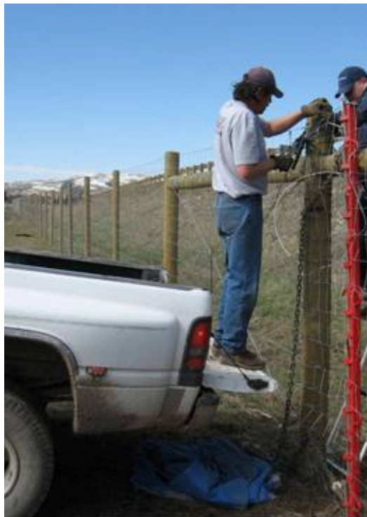
Figure 21. Fence mesh attached to the side away from the road on wildlife fence along Interstate 90 near Bozeman, MT (copyright: Marcel Huijser).
