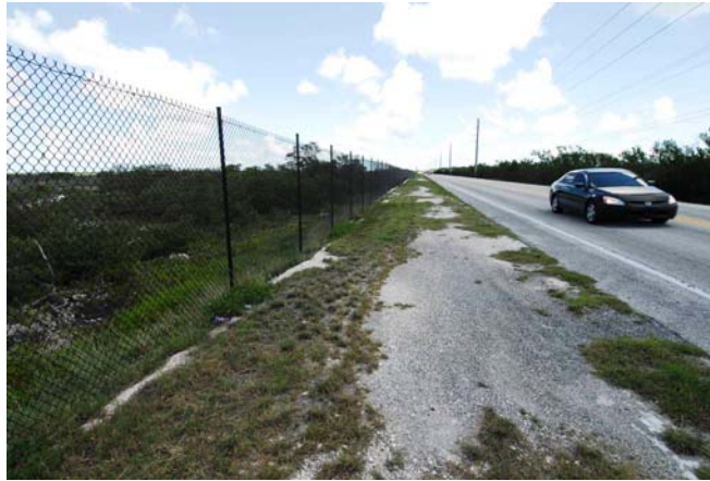
Figure 142. A 1.8-m-high (6-ft-high) fence for Key deer along U.S. Highway 1 on Big Pine Key (copyright: Marcel Huijser).
