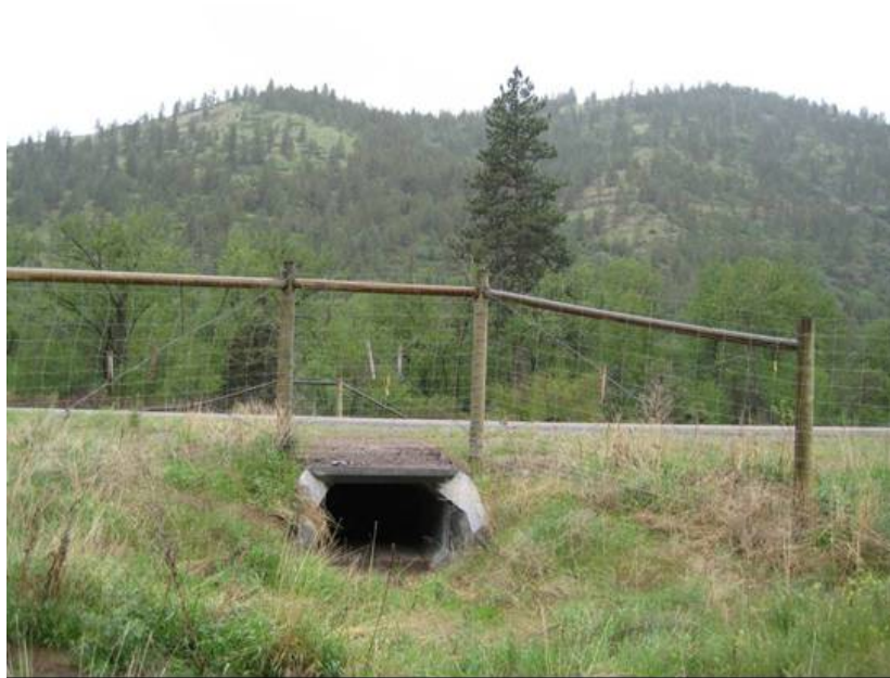
Figure 54. The wildlife fencing continues above a box culvert for medium-sized mammals (copyright: Marcel Huijser).
