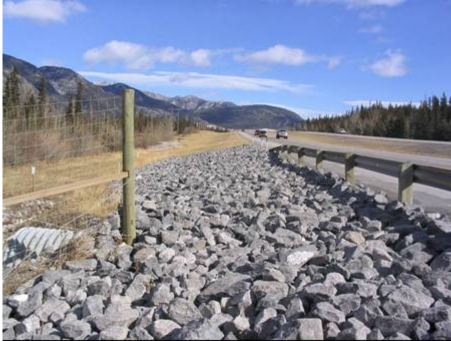
Figure 28. The boulder field at the fence end at Dead Man's Flats along the Trans-Canada Highway east of Canmore, Alberta (copyright: Bruce Leeson).
