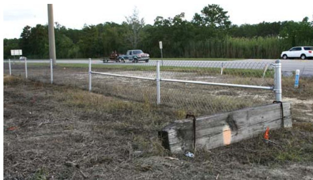
Figure 110. Fences keep Alabama red-bellied turtles from entering the roadway and lead them toward bridges where they can cross under the road (copyright: ALDOT).
