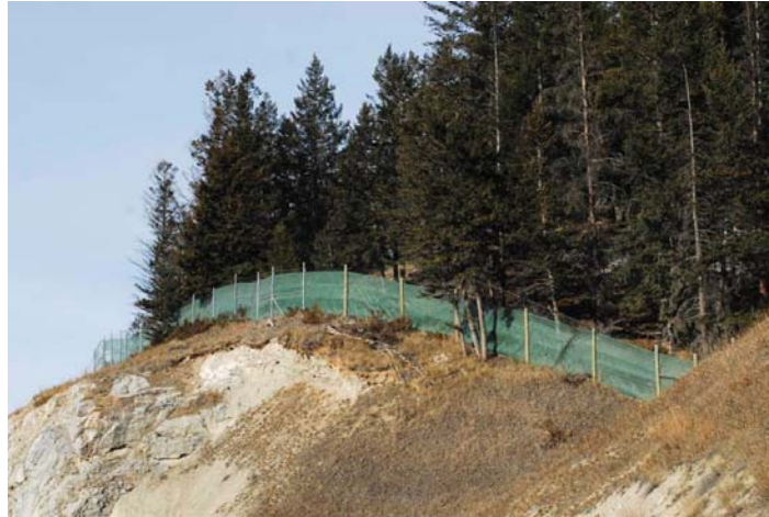
Figure 36. A 2.4-meter-high (8-ft-high) large-mammal chain-link fence along the Trans-Canada Highway between Canmore and Banff, Alberta, is equipped with green mesh to make the fence more visible to bighorn sheep (copyright: Marcel Huijser).
