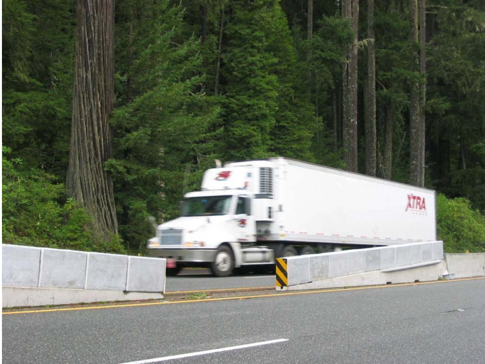
Figure 10. Opening in median barriers designed to allow wildlife to cross the road and the median barriers (copyright: Marcel Huijser).
