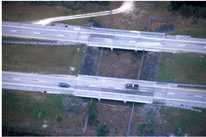
Figure 152. Underpass for hydrology (water flow) and the Florida panther along Interstate 75 in southern Florida (copyright: Marcel Huijser).
