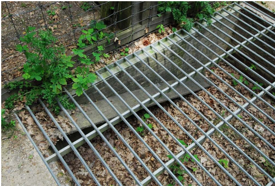
Figure 40. An escape ramp for small species from a wildlife guard pit near the town "De Lage Vuursche", The Netherlands (copyright: Marcel Huijser).
