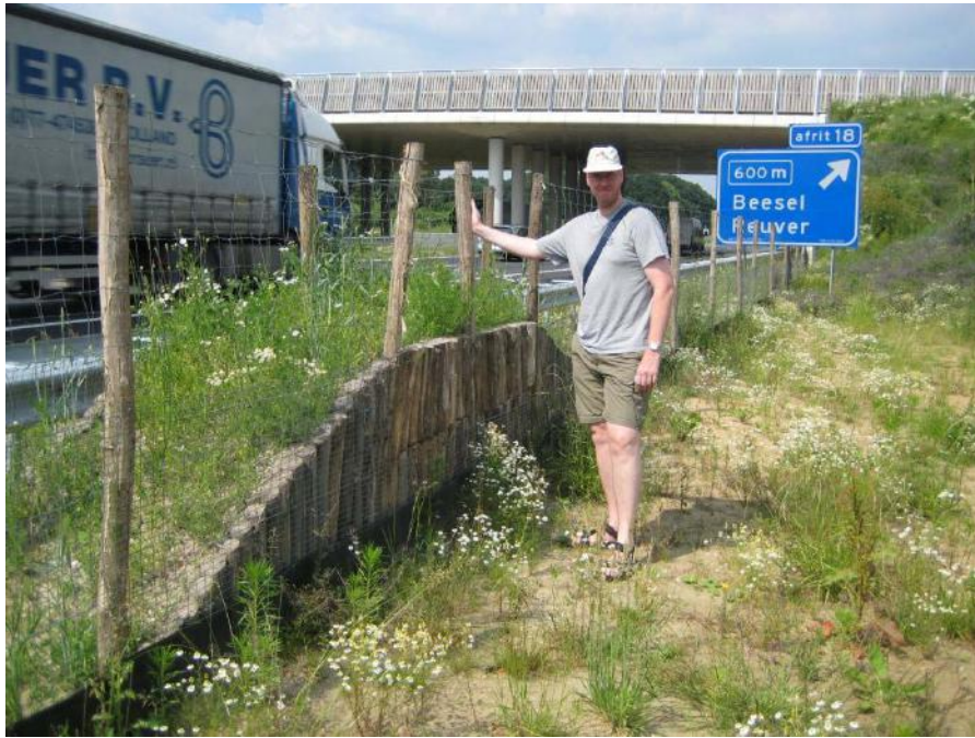
Figure 32. A jump-out intended for Eurasian badger and roe deer along a 2-meter-high (6.6-ft-high) fence along the A73 motorway near Roermond, The Netherlands. Note the wildlife overpass "Waterloo" in the background (copyright: Marcel Huijser).
