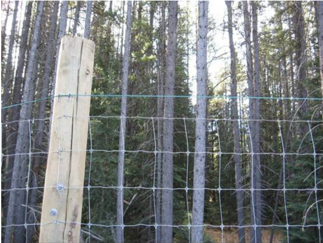
Figure 22. Large-mammal fence with protective top cable along the Trans-Canada Highway in Banff National Park, Alberta (copyright: Marcel Huijser).
