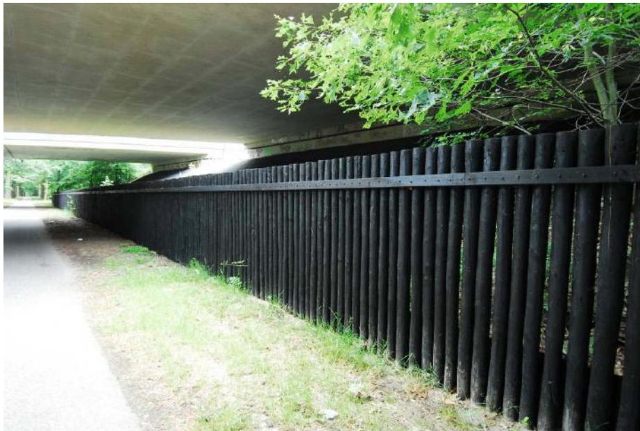
Figure 84. Close-up of the fence, painted black, aimed at reducing light and sound disturbance from traffic (copyright: Marcel Huijser).
