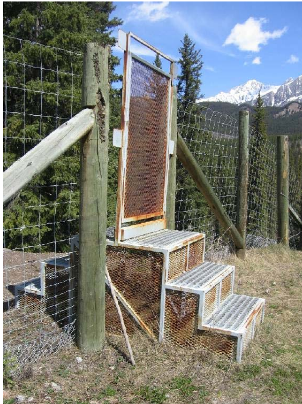
Figure 44. Spring-loaded swing gate in fence allowing access for people along the Trans-Canada Highway in Banff National Park, Alberta (copyright: Adam Ford).
