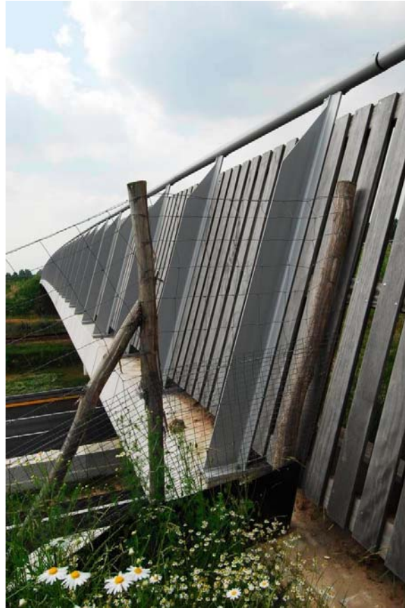
Figure 61. This fence for amphibians and medium- and large-sized mammals connects well to the fence on the wildlife overpass "Waterloo" near the town "Roermond", The Netherlands. Note that the fence on the wildlife overpass also acts as a light and sound barrier (copyright: Marcel Huijser).
