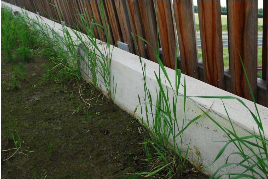
Figure 64. The wildlife fencing on the wildlife overpass "Waterloo" across the A73 motorway near the town "Roermond", The Netherlands. Note that the concrete barrier prevents small animal species from falling off the overpass (copyright: Marcel Huijser).
