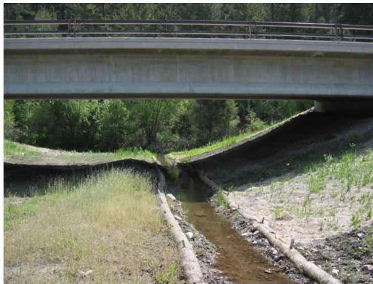
Figure 74. Wildlife underpass (over-span bridge) in combination with a creek crossing along U.S. Highway 93 in Montana (copyright: Marcel Huijser).
