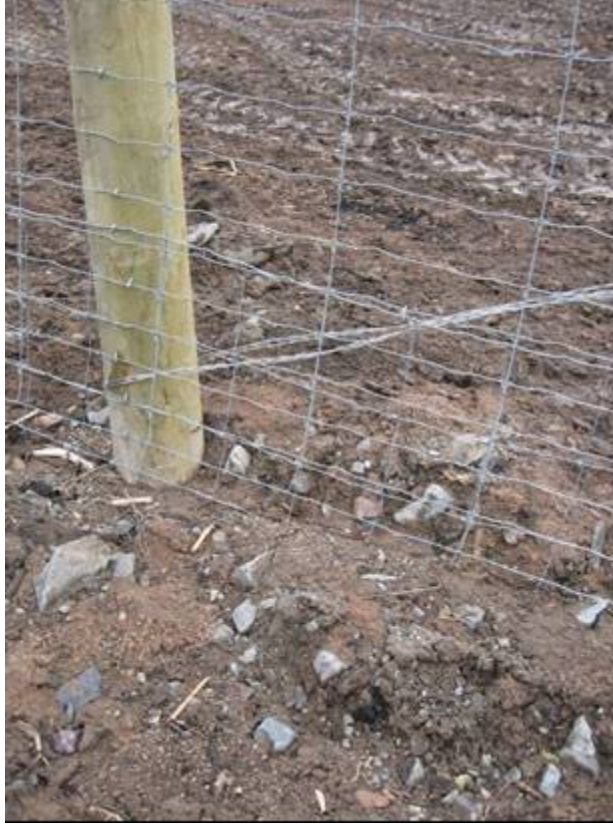
Figure 20. A 2.4-m-high (8-ft-high) large-mammal fence with smaller mesh sizes toward the bottom and additional buried apron (dig barrier) along U.S. Highway 93 in Montana (copyright: Marcel Huijser).
