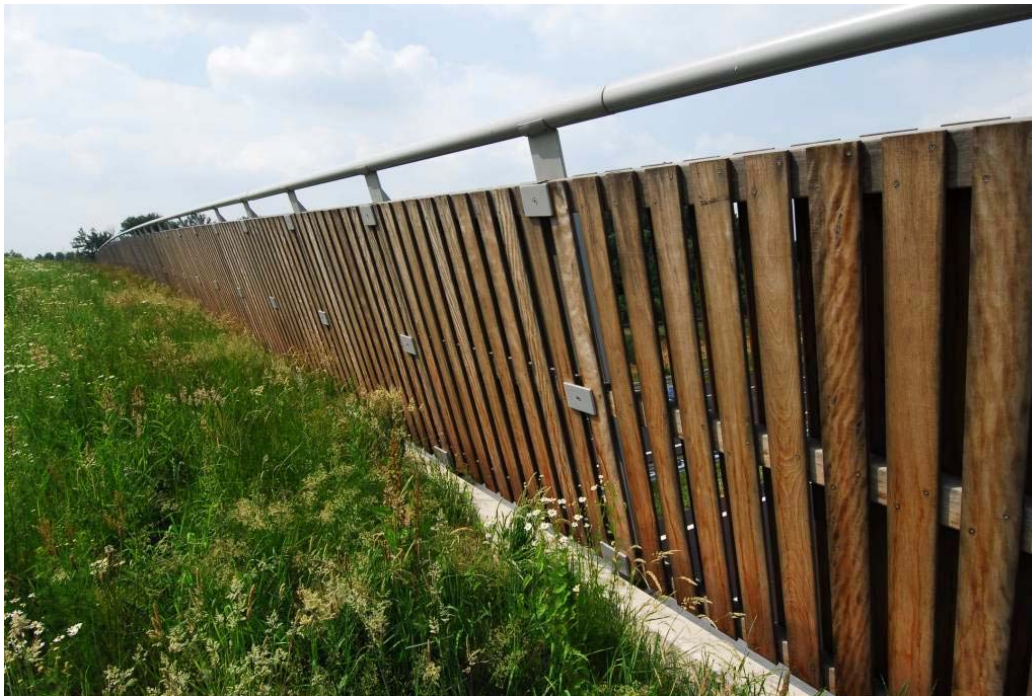
Figure 63. The wildlife fencing on the wildlife overpass "Waterloo" across the A73 motorway near the town "Roermond", The Netherlands, consists of planks that also act as a light and sound barrier (copyright: Marcel Huijser).
