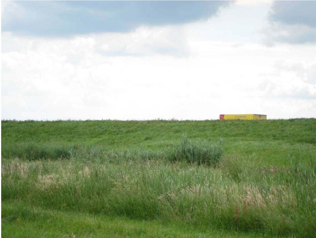
Figure 137. Embankment for birds to encourage them to fly above the traffic on the A27 motorway near Huizen, The Netherlands. Embankments are on both sides of the road, and also serve to reduce sound and light disturbance into the open grasslands. Note that the yellow top of a freight truck shows just above the embankment (copyright: Marcel Huijser).
