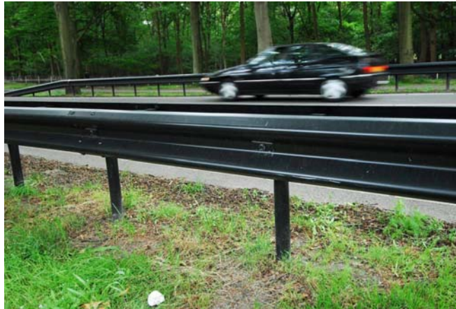
Figure 130. Guardrail painted black near amphibian tunnels and a multiple-use underpass, along the road "Hilversumsestraatweg", near the town Hilversum, The Netherlands. The painted guardrail is expected to reduce glare and light disturbance for amphibians and other species groups (copyright: Marcel Huijser).
