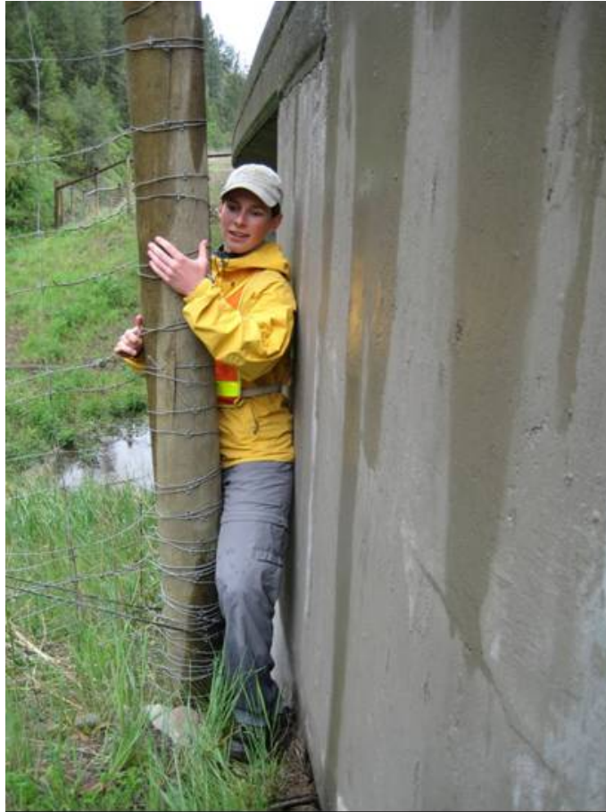
Figure 53. This fence post leaves more space than desired between the post and the wing walls of a crossing structure, allowing some medium- or large-sized mammals to enter the road corridor (copyright: Marcel Huijser).
