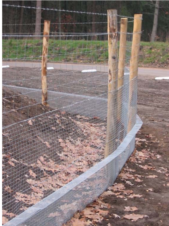
Figure 19. Large-mammal, medium-mammal and small-animal fence combined at the approach to the De Borkeld wildlife overpass across the A1 motorway in The Netherlands (copyright: Marcel Huijser).
