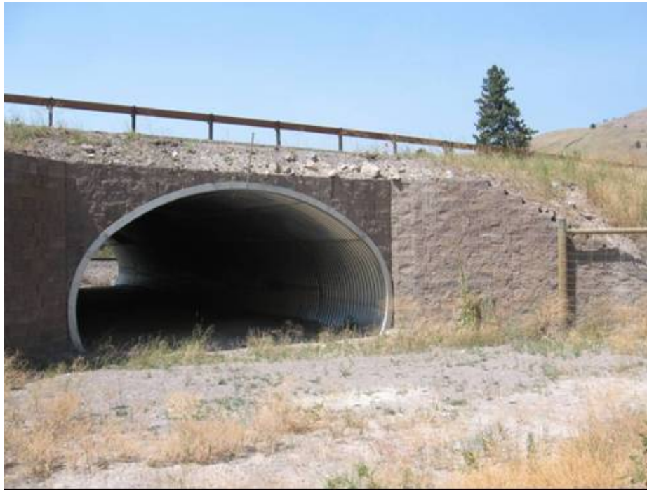
Figure 47. A large-mammal underpass (7–8 m (23-26.2 ft) wide, 4–5 m (13.1-16.4 ft) high) along U.S. Highway 93 south of Ravalli, MT (copyright: Marcel Huijser).
