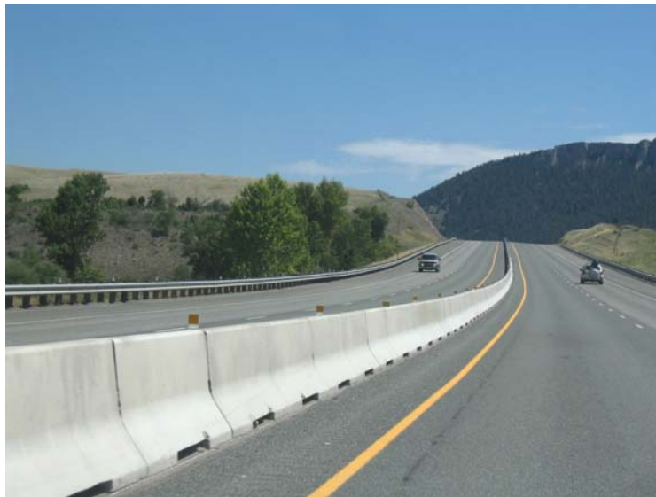
Figure 8. Long sections of median barriers are thought to increase road mortality and reduce animal movements across the road. Note that the small cutouts at the bottom of concrete median barrier are designed for drainage but also allow small animal species to cross under the median barriers (copyright: Marcel Huijser).
