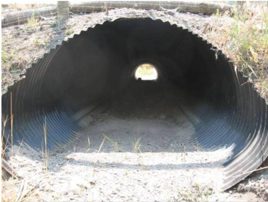
Figure 49. A medium-mammal culvert (2 m (6.6 ft) wide, 1.5 m (4.9 ft) high) along U.S. Highway 93, south of Ravalli, MT (copyright: Marcel Huijser).
