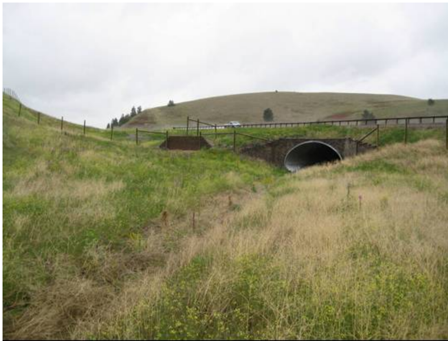
Figure 51. Wildlife underpasses are often installed in low-lying areas with road fill because construction costs are lower (copyright: Marcel Huijser).
