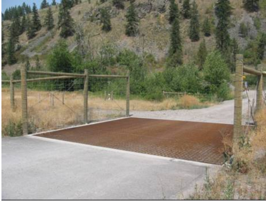
Figure 39. A modified wildlife guard (bridge-grate material) at an access road on U.S. Highway 93, south of Ravalli, MT (copyright: Marcel Huijser).
