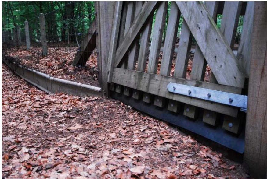
Figure 128. A gate for pedestrians through a badger fence and an amphibian barrier. Note that the gate has sheeting at the bottom to prevent amphibians and other small species from entering the road corridor. Note also that the gate is angled, so that gravity will automatically close the gate (copyright: Marcel Huijser).
