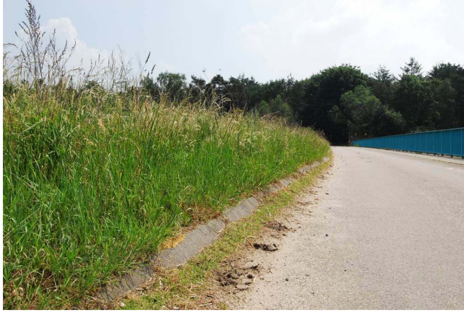
Figure 86. The same overpass as figure 85 showing the gentle grade of the concrete curb, which allows small animals to access the vegetated strip (copyright: Marcel Huijser).
