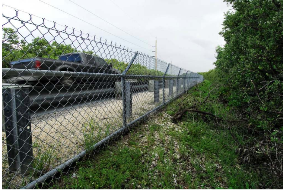
Figure 105. A short section of fencing (30 m (100 ft) long, 90 cm (3 ft) high) aimed at directing American crocodiles to 1.8-m-wide (6-ft-wide) culverts along Highway 905A, just south of the Card Sound Bridge in Key Largo (copyright: Marcel Huijser).
