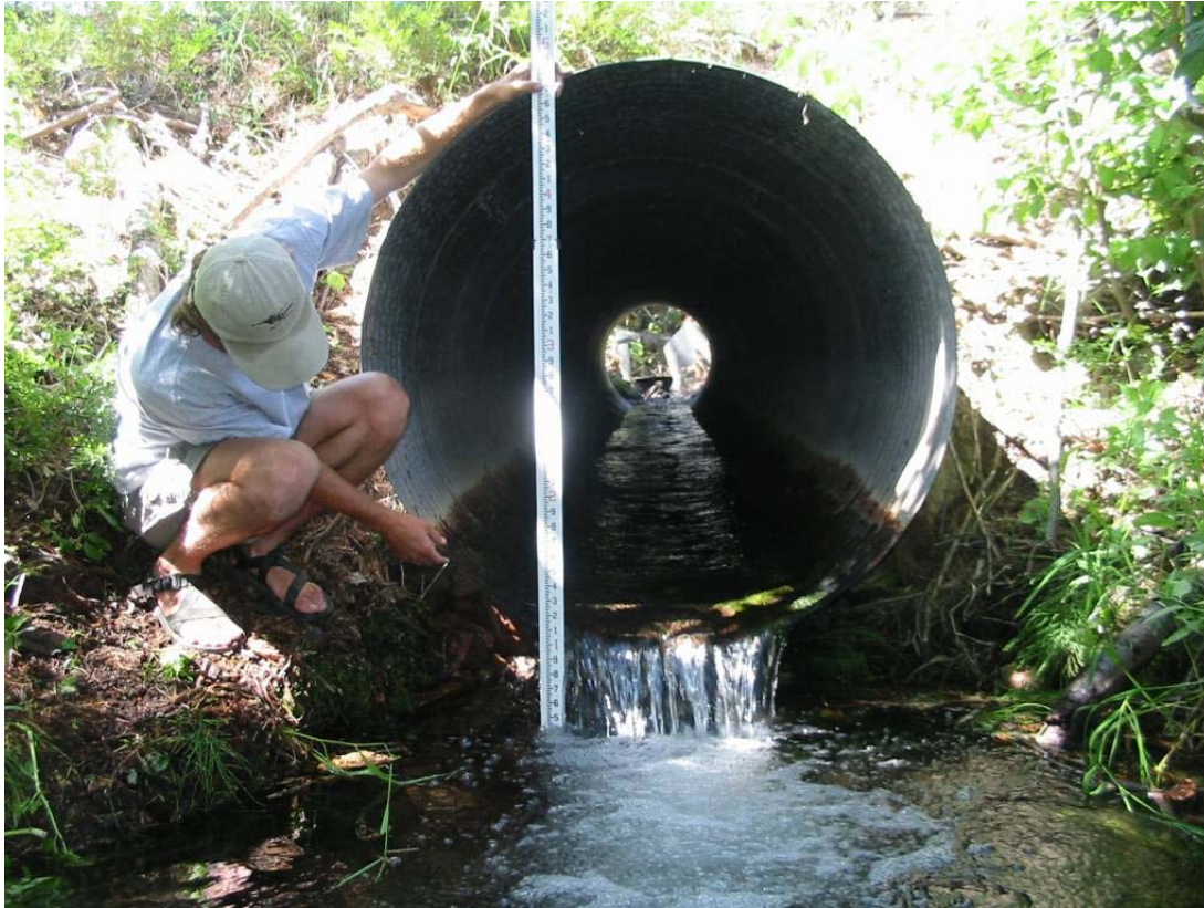
Figure 70. Structures built to pass water typically should be designed to avoid erosion and allow passage of aquatic species. The structure shown has no adaptations for terrestrial species and is also likely to be impassable for many aquatic species (copyright: Matt Blank).
