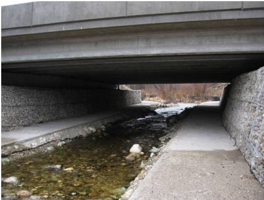
Figure 77. Concrete walkways for wildlife on both banks of a creek at an over-span bridge along U.S. Highway 93, south of Missoula, MT (copyright: Marcel Huijser).
