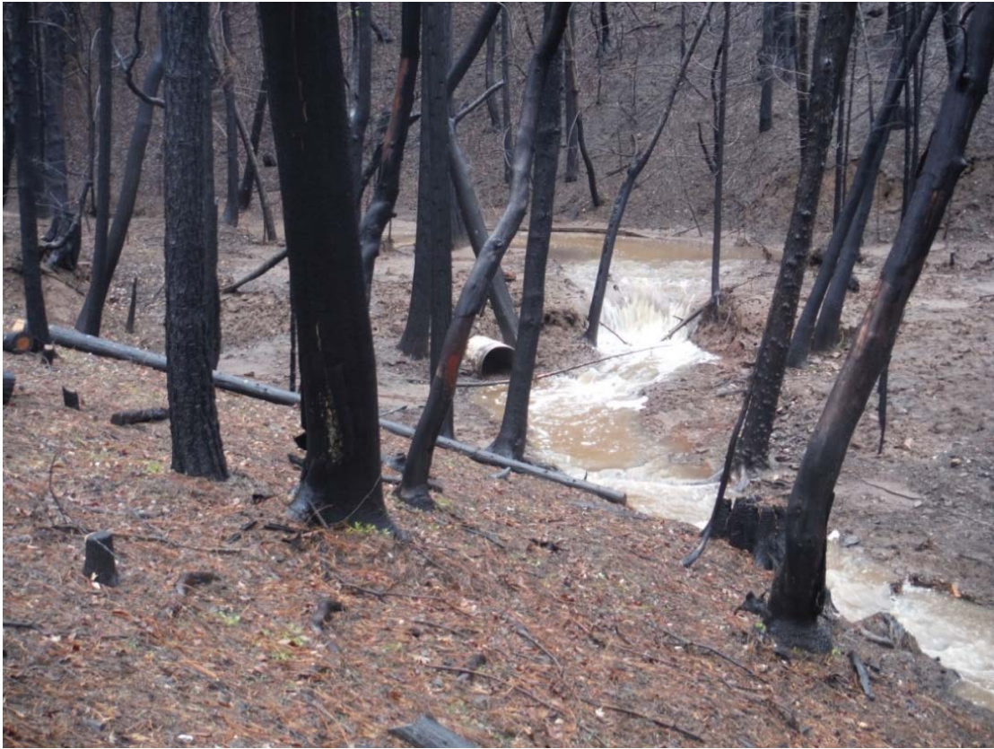
Figure 17. Plugged culvert located in the 2015 Butte Fire area (Calaveras County) during winter storms in March 2016 (photo provided by Cheryl Hayhurst, CGS).
