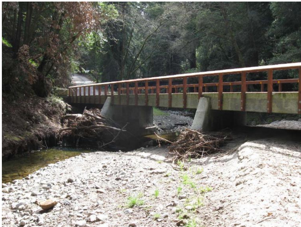
Figure 33. Heavily reinforced concrete bridge with sacrificial wood railings that is designed to be overtopped in the event of a flood event, located in Santa Cruz County.
