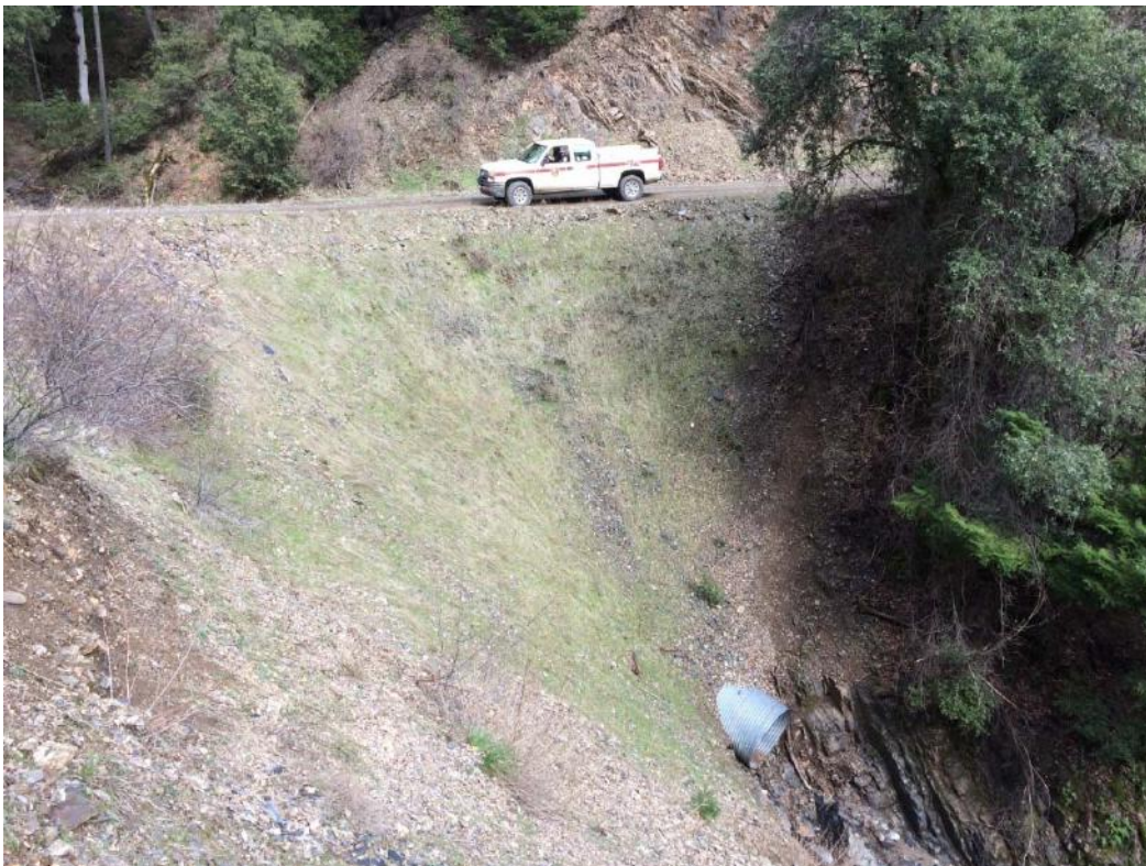
Figure 19. Example of a watercourse crossing with a large fill and a relatively small culvert.
