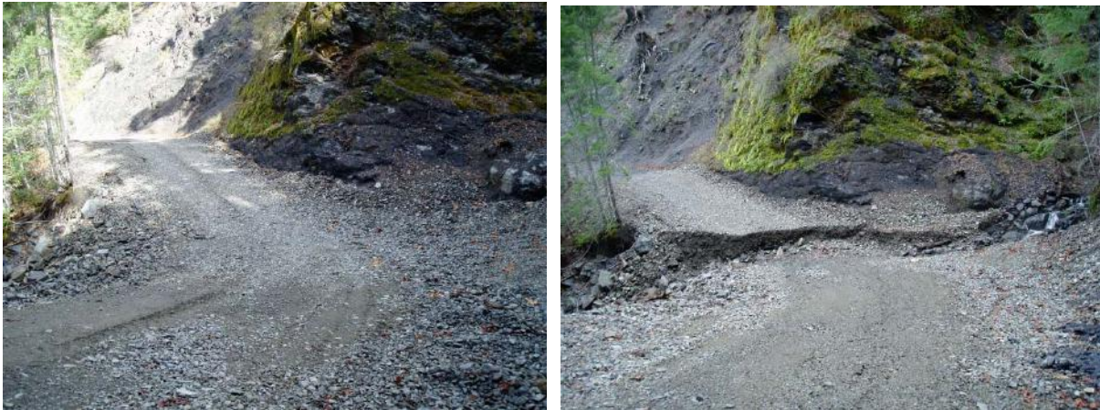
Figure 21. Rock-armored crossing where the outlet rock was undersized, poorly placed, and with insufficient quantity, resulting in post-construction failure. This situation illustrates the need for appropriate sizing of the rock on the outboard edge and close oversight during construction.
