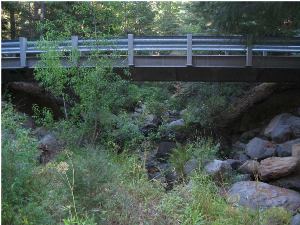
Figure 28. Permanent bridge installed in Shasta County. The bridge spans the entire channel and is positioned above the anticipated flood flow elevation.
