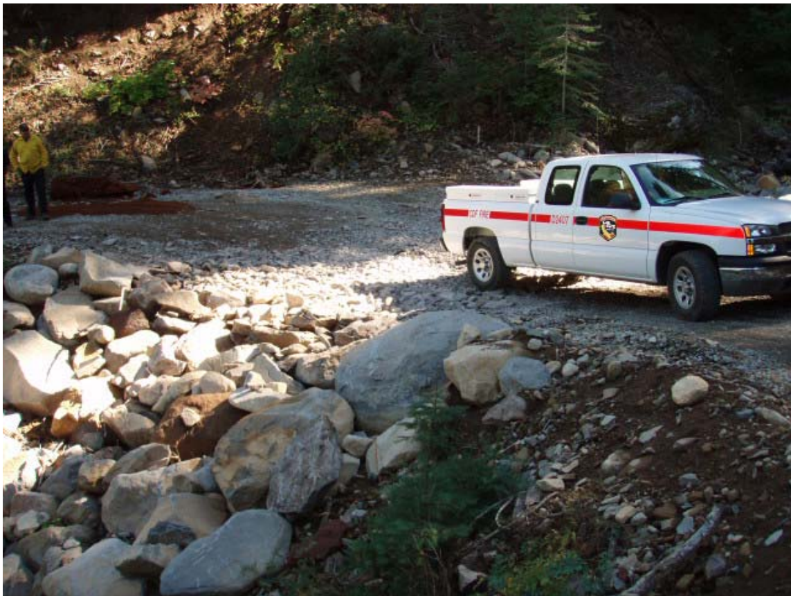
Figure 20. Example of a rock-armored crossing installed in LaTour Demonstration State Forest, Shasta County.
