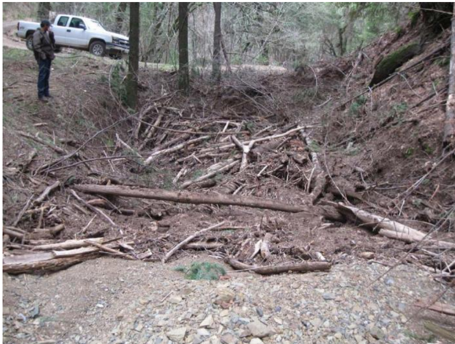
Figure 8. Example of woody debris blocking a culvert inlet following a January 2012 storm event in northern California. The culvert, which is not visible under the debris, is narrower than the channel is wide immediately upstream of the crossing.
