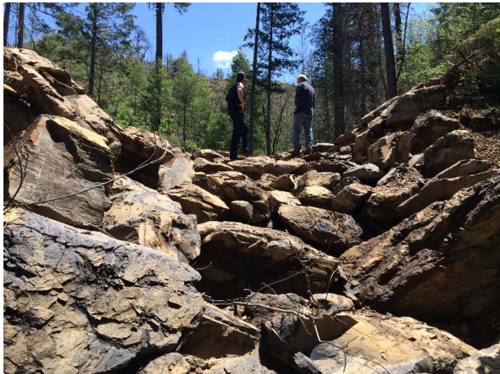
Figure 27. A rock-armored crossing with well-defined armored outfall looking downslope (upper photo) and upslope (lower photo), located in northeastern California.
