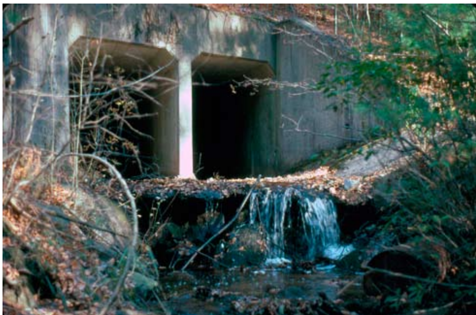
Figure 1.21—Outlet drop formed by scour at the downstream end of an asphalt apron. Photo: Scott Jackson, University of Massachusetts.
