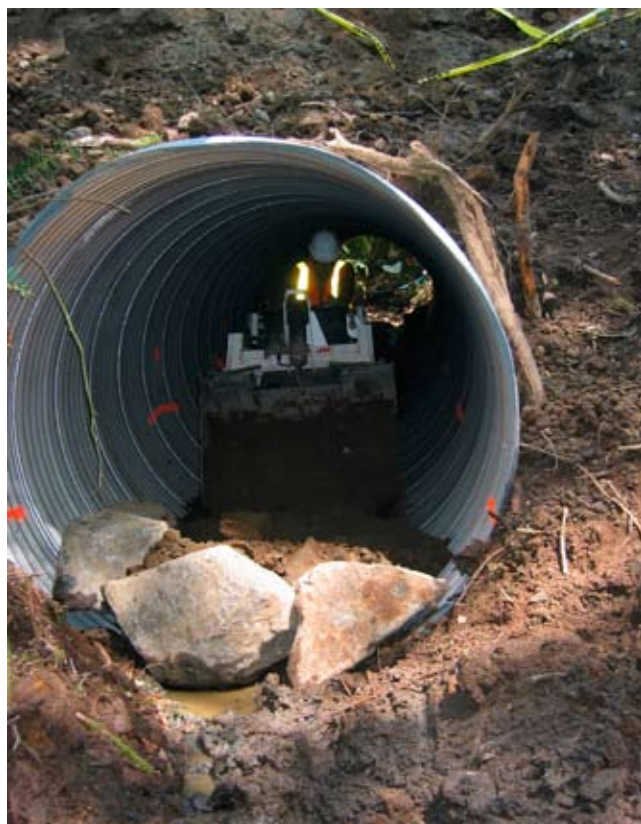
Figure 7.13—Hand labor walk-behind equipment.
