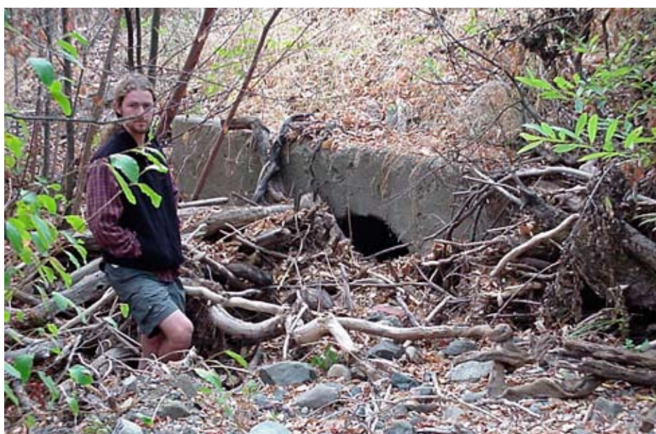
Figure 1.16—Debris and sediment at culvert inlet can be a fish barrier. Photo courtesy of Ross Taylor and Associates, McKinleyville, California.
