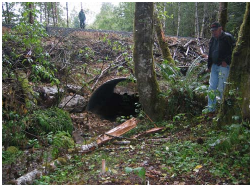
Figure 7.11—Clearing debris scattered for erosion control.
