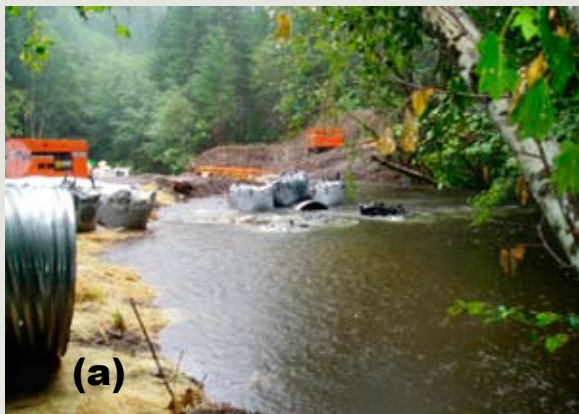
Figure 8.9—Unusual summer storm overwhelms bypass system. (a) Looking downstream at bypass pipe, now in mid-channel. (b) Looking downstream through the open excavation.
