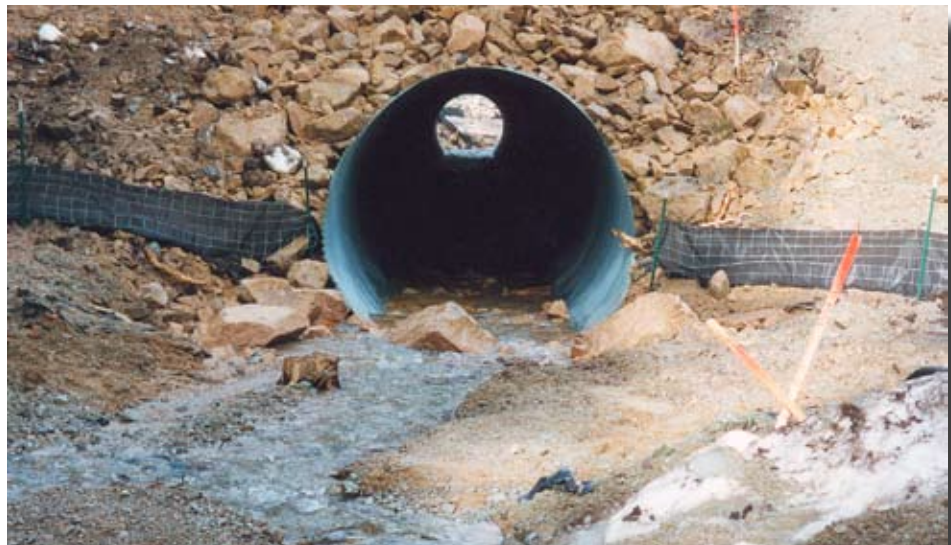
Figure 7.22—Typical silt-fence installation.
