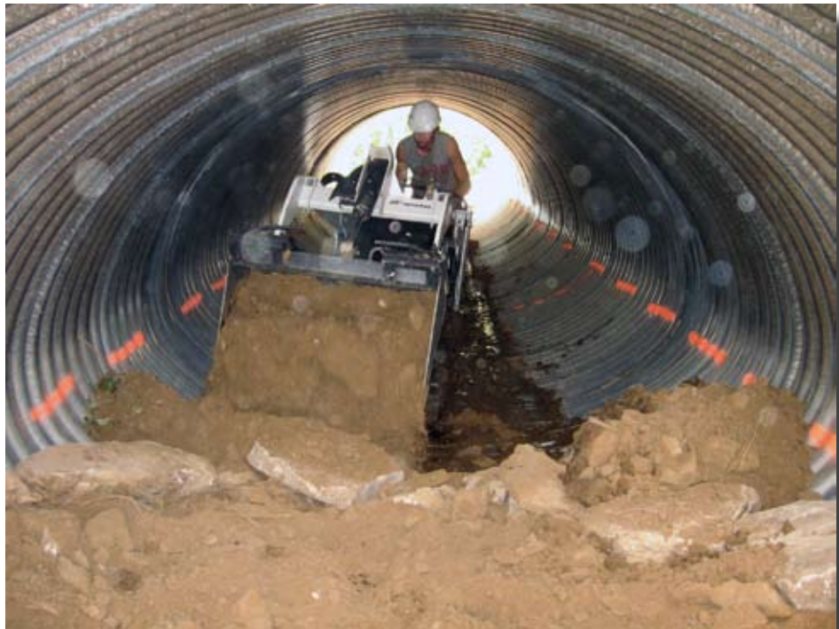
Figure 8.15—Bobcat placing bed material to marked elevation.
