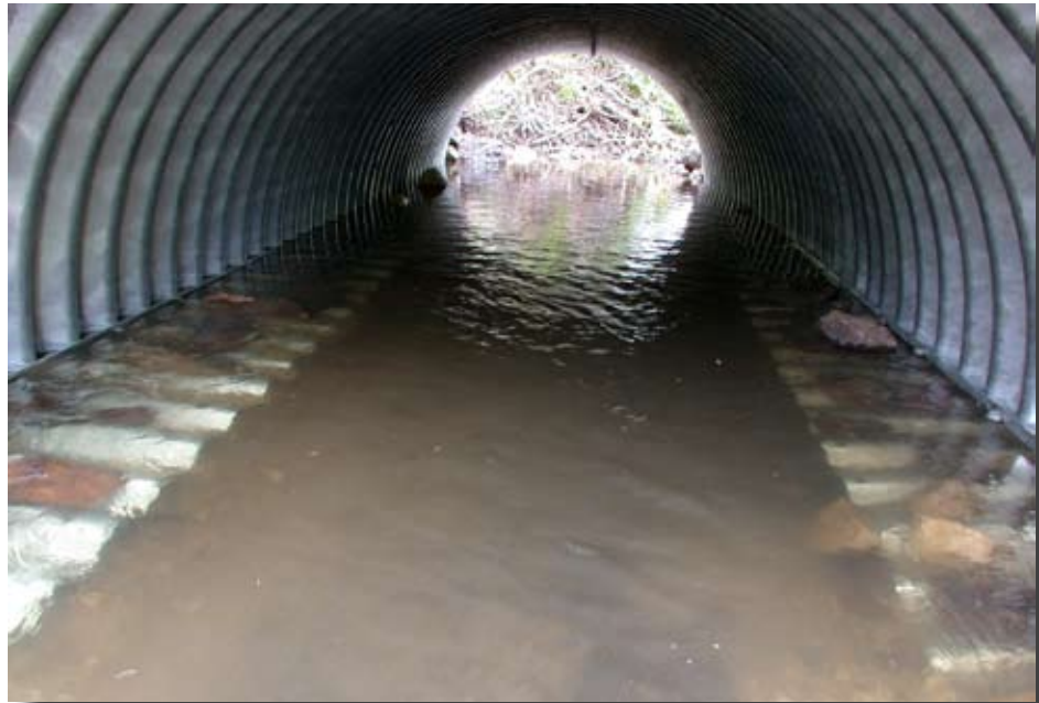
Figure 7.7—Open-bottom pipe arch with metal footings.
