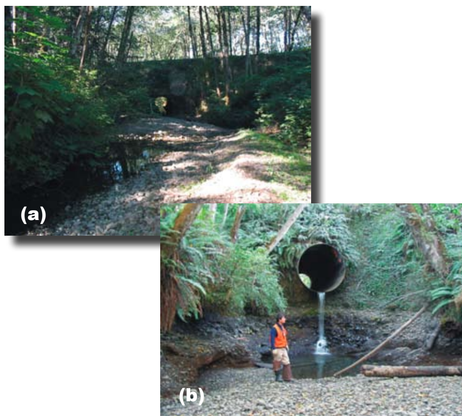
Figure A.1—(a) Aggraded (filled) channel upstream of narrow culvert; (b) incised (scoured) channel downstream of culvert, Save Creek, Olympic National Forest, Washington.
