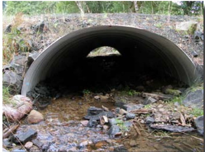
Figure 7.3—1-piece corrugated metal pipe arch (embedded).
