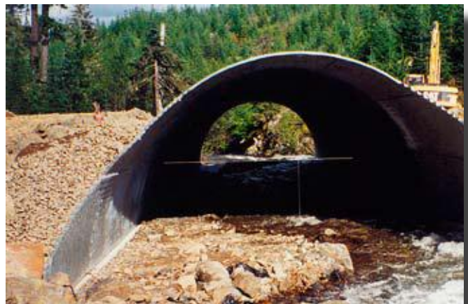
Figure 7.5—Multiplate open-bottom pipe arch.
