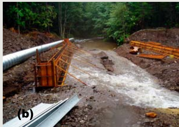
Figure 8.9—Unusual summer storm overwhelms bypass system. (a) Looking downstream at bypass pipe, now in mid-channel. (b) Looking downstream through the open excavation.
