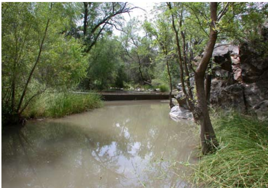
Figure 1.20—Elevated concrete-slab ford eliminates aquatic habitat area directly underneath the structure and blocks fish passage at low flows. However, it may not significantly alter the character of aquatic habitats upstream and downstream.
