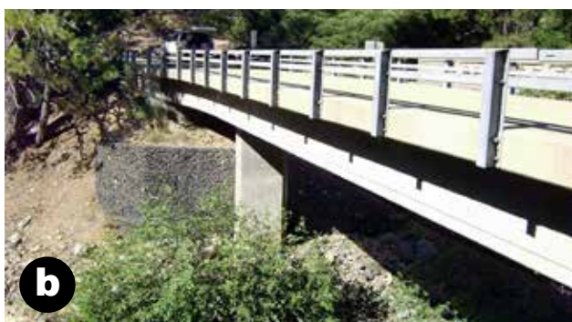
Figure 112—Bridges with rock riprap (a) and gabion (b) scour protection around the abutments since the bridges are located on bends in the stream (river bends are problematic locations).
