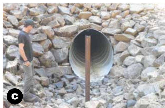
Figure 78—Examples of trash racks added to small culvert pipes to prevent plugging. Note that the riser with trash rack (a) is downstream of a fire area where considerable sediment is anticipated that often plugs small pipes. Debris can float over the culvert inlet at high flows (b). The single post (c) upstream of the pipe is used to help orient debris to go through the pipe rather than plugging across the inlet.
