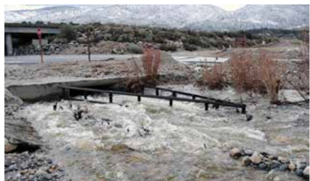
Figure 77—Use of trash racks to prevent plugging of a culvert or bridge from upstream large boulders and debris. (Bottom photo courtesy of Vincent Barandino.)
