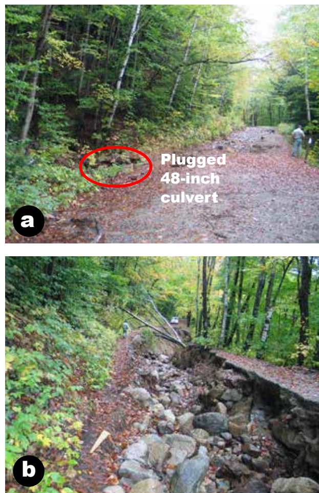
Figure 35—Stream diversion caused by a plugged 48-inch corrugated metal pipe that forced water down the road (a) and caused the roadway fill washout (b) when it exited the road, White Mountain National Forest. (Courtesy of Bob Gubernick.)
