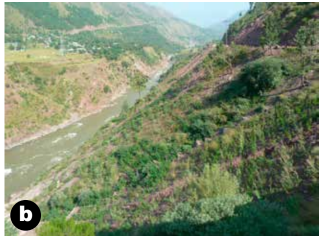
Figure 142—Before (a) and after one season (b) photos of brush layering used to stabilize an entire hillside after storm damage in Pakistan. (Photos courtesy of Asif Faiz, World Bank.)
