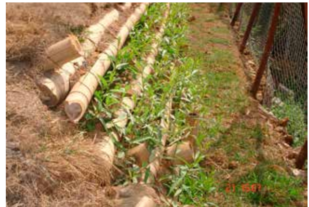
Figure 142—Before (a) and after one season (b) photos of brush layering used to stabilize an entire hillside after storm damage in Pakistan. (Photos courtesy of Asif Faiz, World Bank.)
