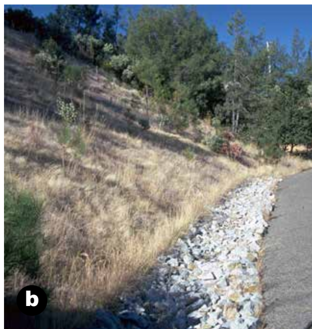
Figure 48—Common types of vegetative erosion control measures including grasses on a closed road (a) and deep-rooted shrubs and trees (as well as grass) on a cutslope (b).
