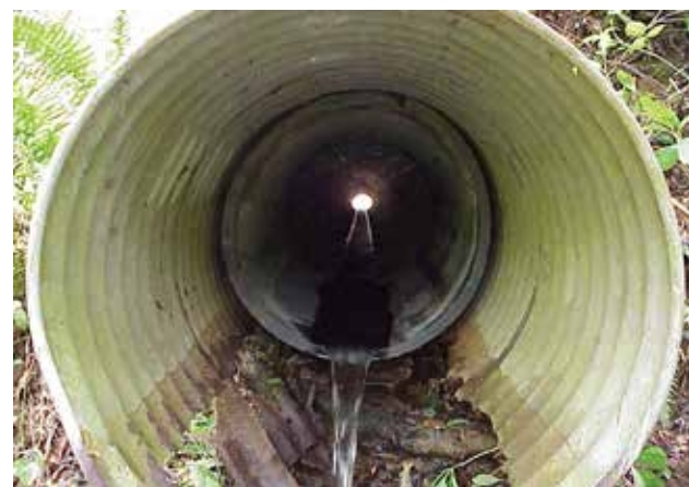
Figure 73—Culvert rehabilitation with a cement grout or a new rubber slipliner. (Bottom photo courtesy of Clackamas County, Oregon.)
