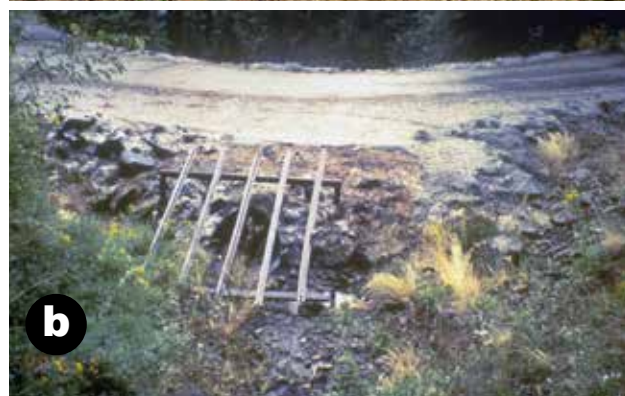
Figure 77—Use of trash racks to prevent plugging of a culvert or bridge from upstream large boulders and debris. (Bottom photo courtesy of Vincent Barandino.)
