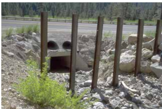
Figure 72—Increase culvert capacity using multiple pipes or stacking pipes on top of the original pipe. Typically, stacking pipes is only an emergency solution. Also note that multiple pipes increase the risk of plugging.
