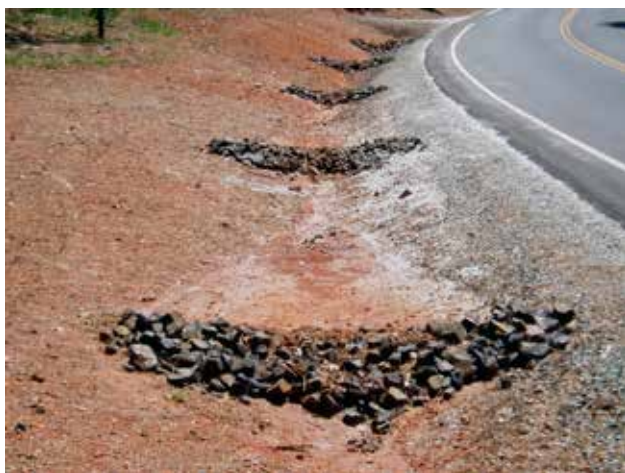
Figure 29—Check structures of rock or bagged gravel installed in the ditch to reduce flow velocity and trap sediment.
