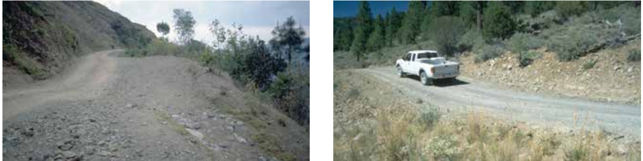
Figure 16—The form of rolling dip cross drains on various roads.
