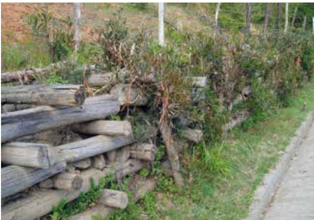
Figure 142—Before (a) and after one season (b) photos of brush layering used to stabilize an entire hillside after storm damage in Pakistan. (Photos courtesy of Asif Faiz, World Bank.)
