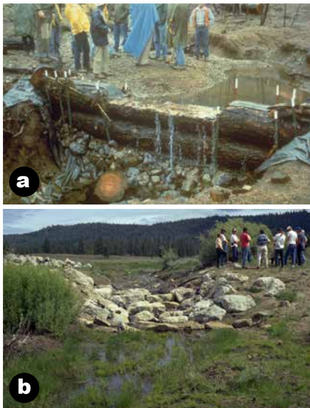
Figure 124—Gully stabilization structures made of logs (a) and of loose rock (b).
