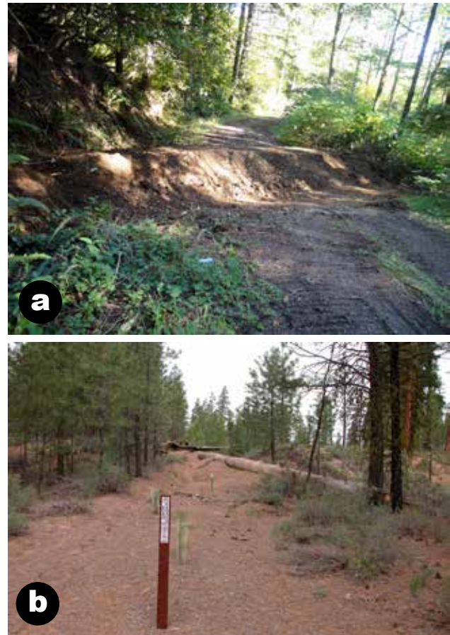
Figure 154—Examples of roads that have been placed into storage. Photo (a) shows a road that has been closed using a waterbar. (Courtesy of Ken McCall/Karen Bennett.) Photo (b) shows the road has been closed with a log and berm, plus some vegetation. (Courtesy of Greg Napper.)
