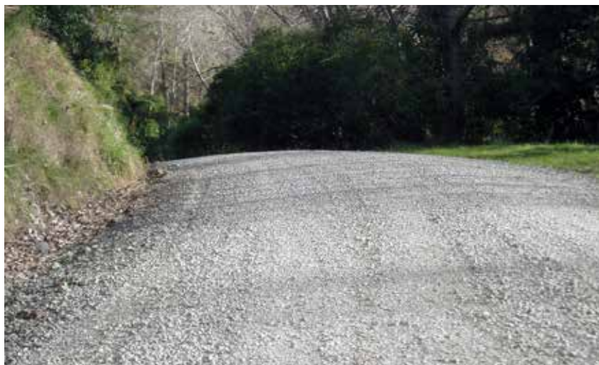
Figure 13—Basic road surface drainage options of an inslope, outslope, or a crown section. The photo shows a crown road with an inside ditch.
