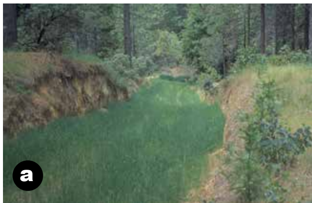
Figure 48—Common types of vegetative erosion control measures including grasses on a closed road (a) and deep-rooted shrubs and trees (as well as grass) on a cutslope (b).
