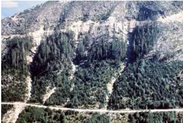
Figure 57—Debris slides, often triggered during a storm event from failing fills, that started at the upper road and ultimately impacted the lower road. (Courtesy of Jim Doyle.)
