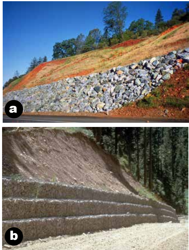
Figure 131—Commonly used retaining structures, such as a rock buttress (a) and a gabion wall (b).
