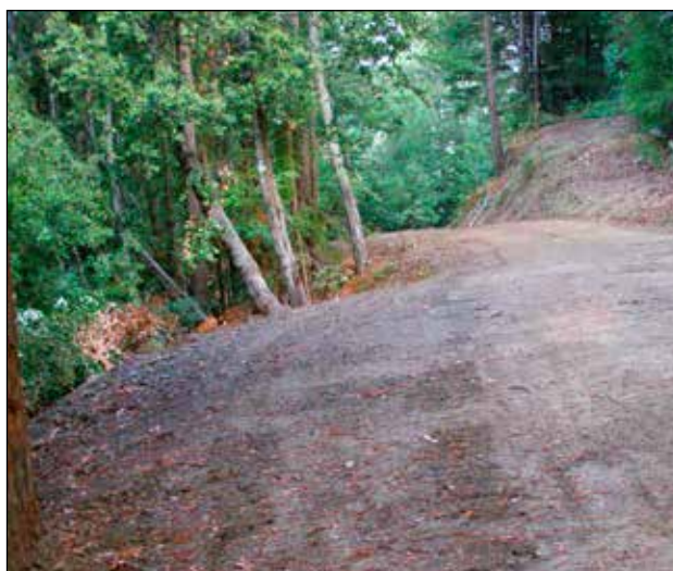
Figure 14—Examples of a rolling grade to minimize concentration of water on the road.
