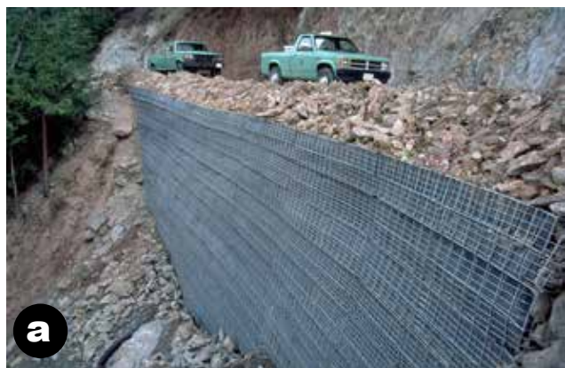
Figure 133—A welded wire MSE wall (a) and a geotextile wall (b), both used because of their relatively low cost and ease of construction.
