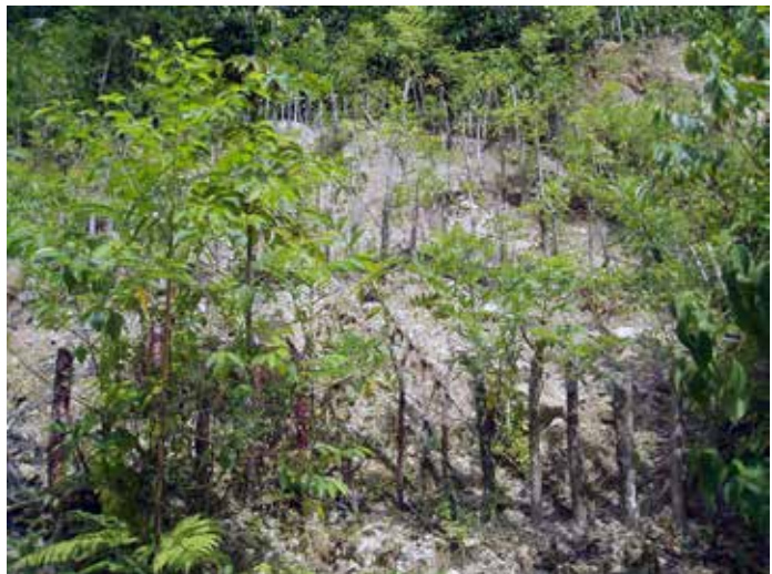
Figure 140—Use of live stakes for slope stabilization. (Sketch (a) courtesy of Robbin B. Sotir & Associates, Inc.)
