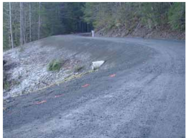
FIGURE 38 Deep patch during and after construction in Gifford Pinchot National Forest in Washington (Courtesy: B. Collins).
