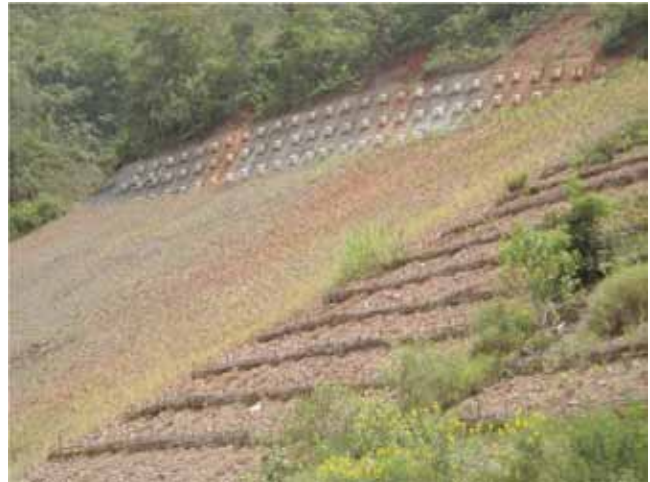
FIGURE 24 Live fascines (Courtesy: G. Keller).
