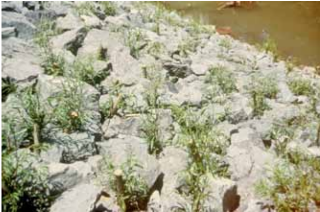
FIGURE 27 Rock joint planting (Courtesy: R. Sotir).
