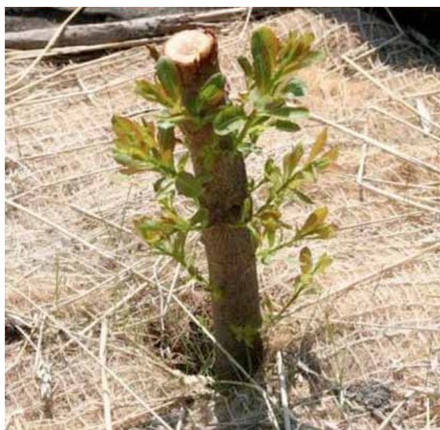
FIGURE 23 Live stake used to pin down matting (Courtesy: R. Sotir).
