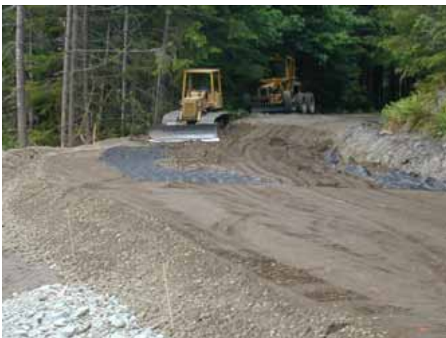
FIGURE 38 Deep patch during and after construction in Gifford Pinchot National Forest in Washington (Courtesy: B. Collins).
