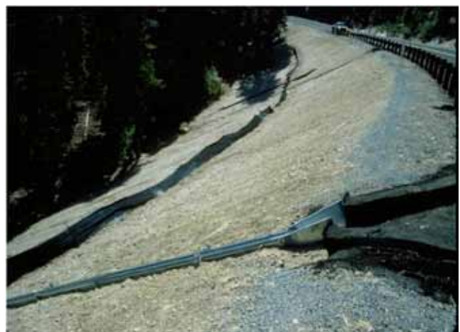
FIGURE 7 Down-drain (Courtesy: G. Keller).
