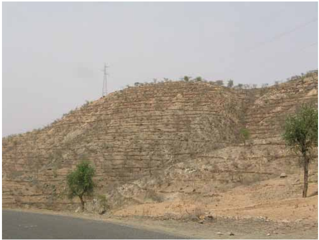
FIGURE 43 Constructed terraces on exposed slopes, Asmara-Assab Road, Eritrea (Courtesy: A. Faiz).
