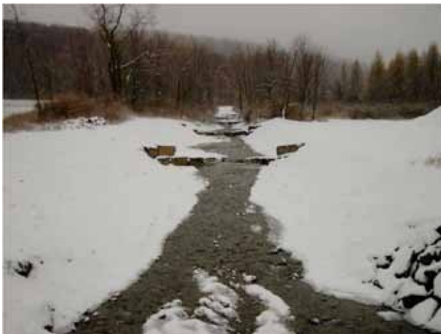
FIGURE 20 Stone check dams (Courtesy: D. Orr).
