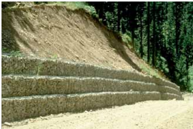
FIGURE 35 Low gabion wall and gabion wall stabilization at top of fill slope in Timor (Courtesy: G. Keller and C. Bennett).
