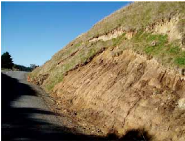
FIGURE 4 Shallow cut failure just below grass root depth. Use deep-rooted vegetation for slope stabilization (Courtesy: G. Keller).
