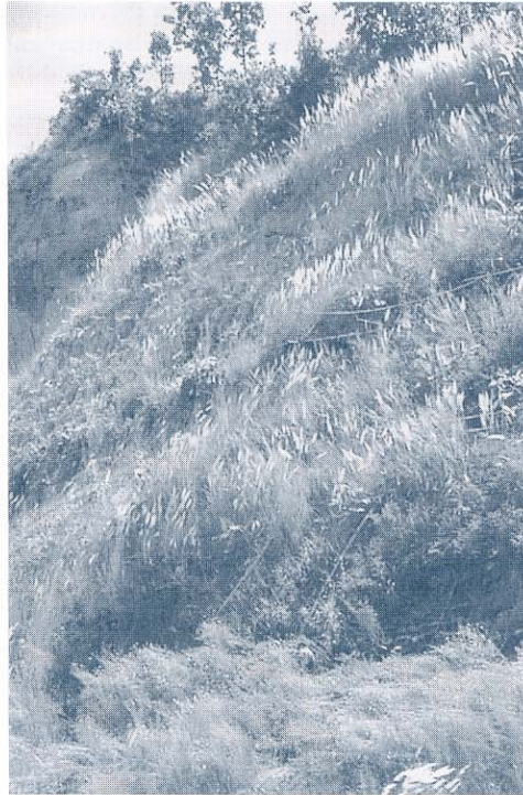
hydro-seeding can yield spectacular results for surface covering, but this example was estimated to cost about thirty times more than the manual method
