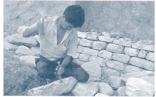
Dressing stone during the construction of dry stone dentition
