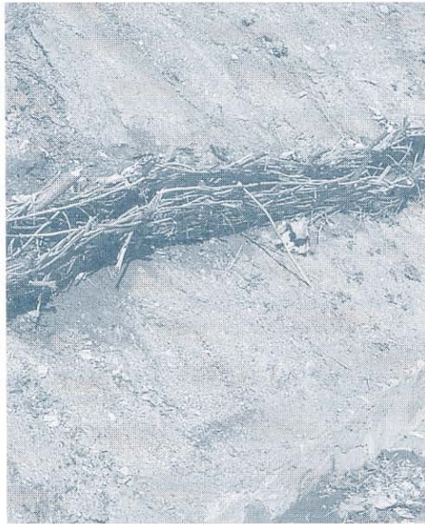
Live wattle fences can be effective at catching falling debris on gentle slopes
