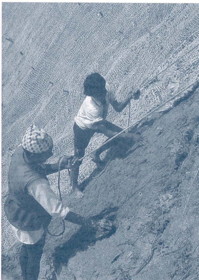
Placing jute netting on a steep cut slope
