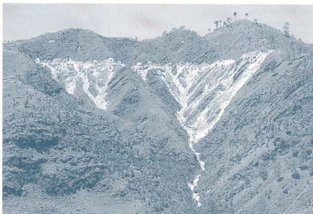
Careless spoil disposal on long, steep slopes can cause very extensive damage
