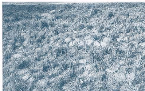
Cobbling with vegetation planted between the stones provides strong armouring
