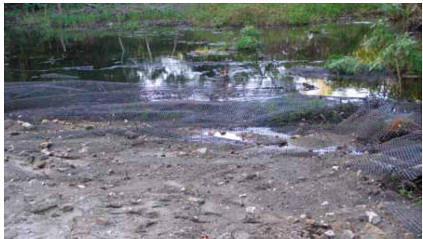
Figure 3-57—Geogrid has been rolled out over a swamp to provide reinforcement for the roadway fill (note that this is a poor road location).
