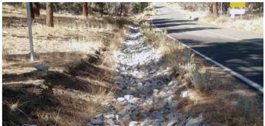
Figure 3-95—A rock-armored ditch to control the waterflow and prevent downcutting of the ditch.
