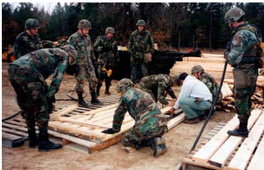
Figure 3-147—Wood pallets used for a temporary road.
