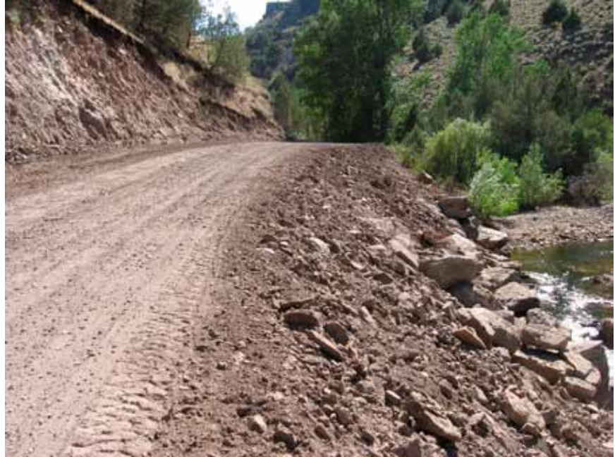
Figure 3-142—Road centerline is shifted away from the river after reconstruction with a flatter, stable fillslope and riprap armor along the river (courtesy of Mike Balen).
