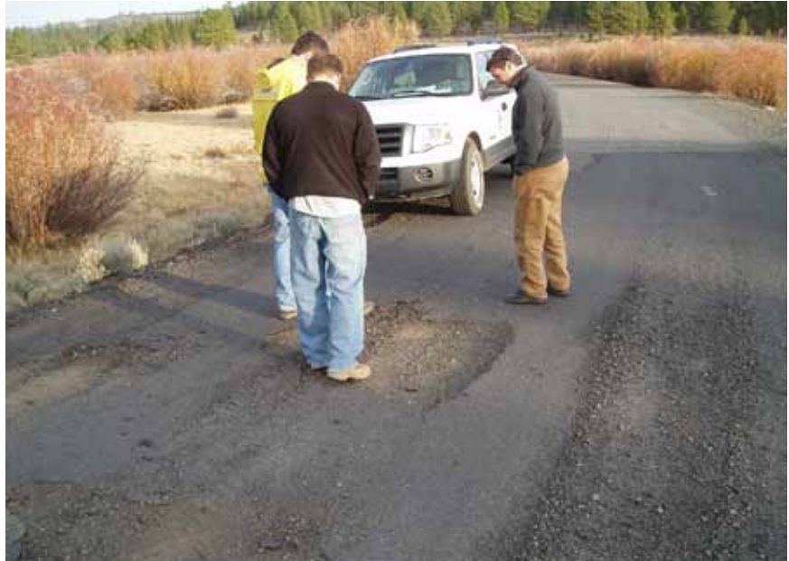
Figure 2-17—Bituminous surface treatment failures on old chip seal road surfaces.
