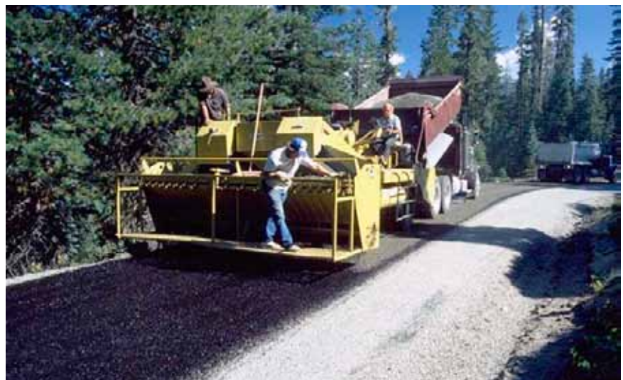
Figure 3-73—A BST (chip seal) operation with chips being spread on an emulsified asphalt over base aggregate.
