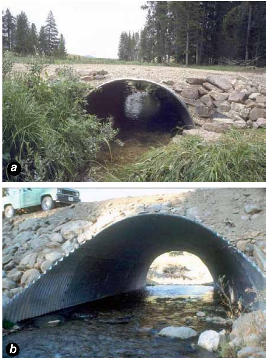
Figure 3-120—(a) and (b) Small and large embedded fish-friendly culverts with a natural stream bottom for aquatic organism passage.
