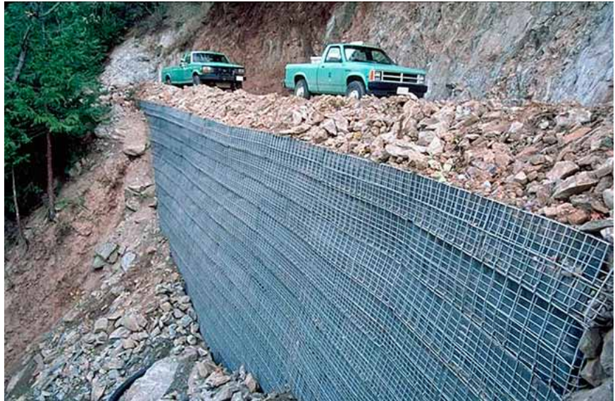
Figure 3-35—A welded wire MSE wall, commonly used by the Forest Service.
