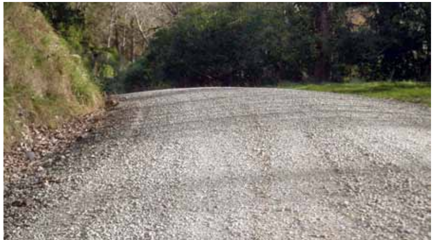
Figure 3-81—A road with a good crown, where the road is half insloped and half outsloped, breaking surface water concentrations into two parts.
