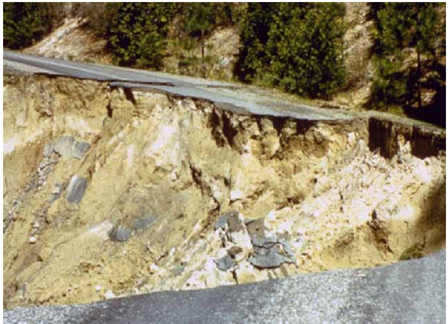
Figure 2-10—A fillslope settling or beginning to fail, and a failed roadway fill.
