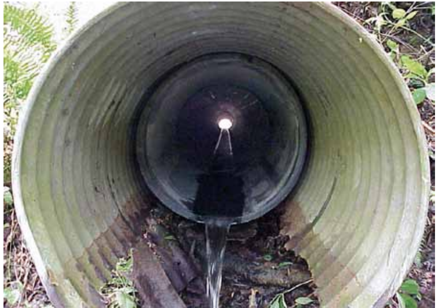
Figure 3-118— New high density polyethylene pipe that has been pulled inside the old CMP pipe with a badly corroded invert (photo courtesy of Clakamis County, Oregon).
