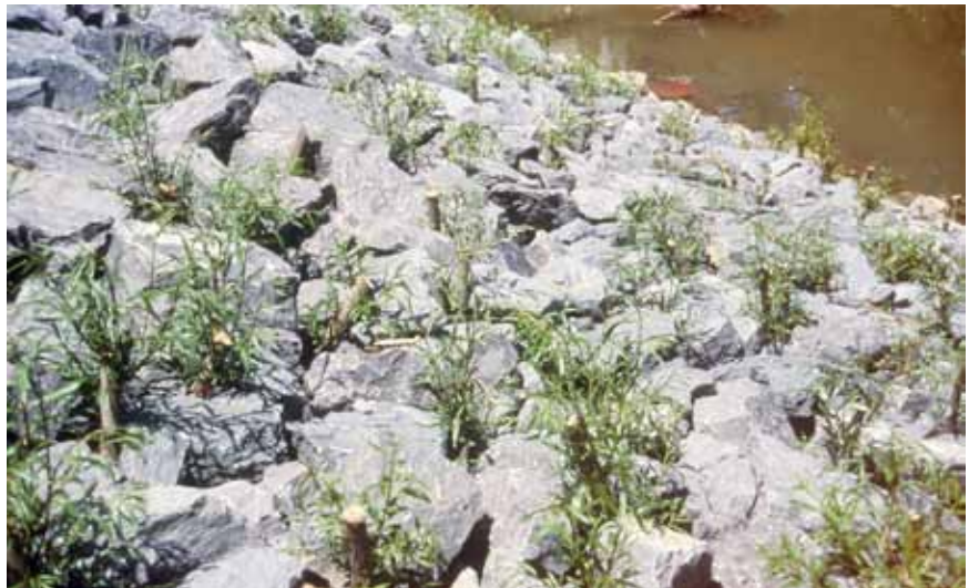
Figure 3-133—An installed joint planting system (courtesy of Robbin B. Sotir & Associates, Inc.).
