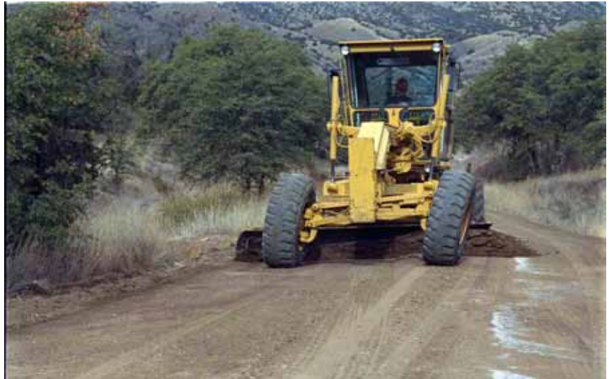
Figure 3-54—Use grader maintenance to keep the road surface properly shaped and drained.
