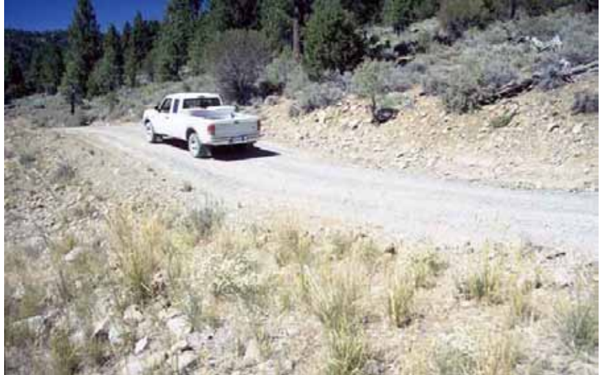
Figure 3-101—Rolling dip cross drains are not susceptible to plugging when shaped properly.
