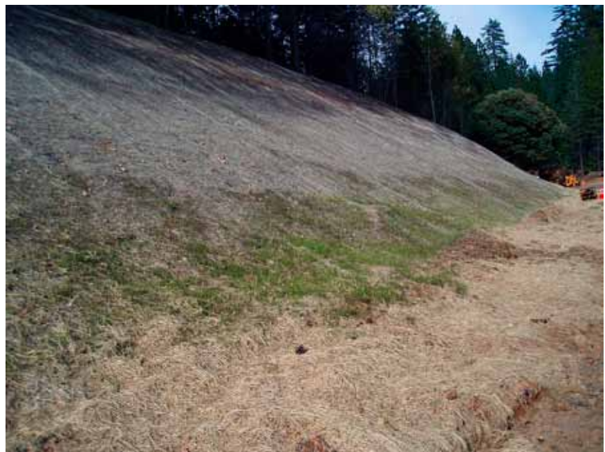
Figure 3-6—Erosion control netting over grass and straw mulch on a cutslope.
