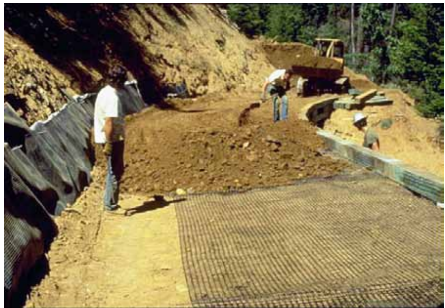
Figure 4-2—Geogrid reinforcement in a timber-faced retaining wall.
