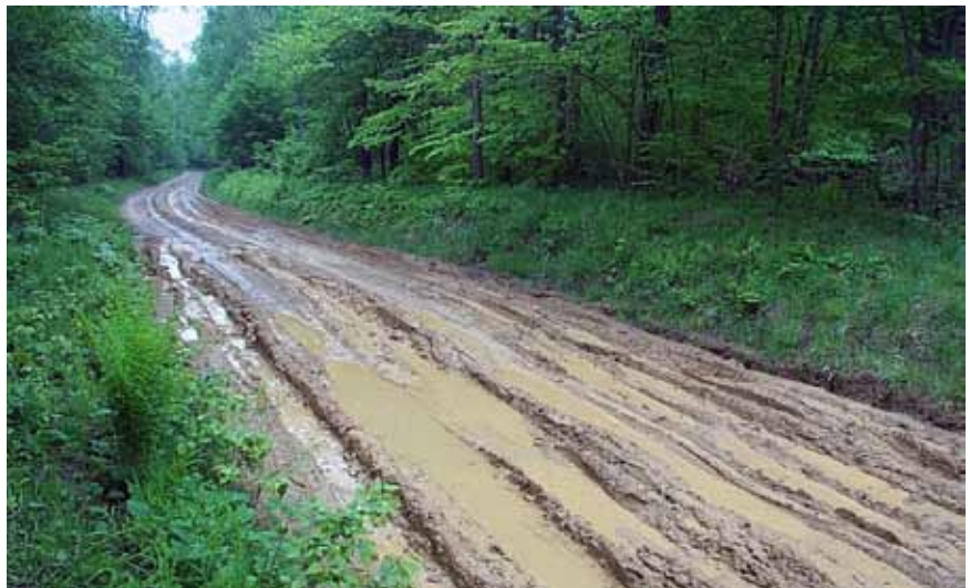
Figure 3-83—An entrenched road where water cannot be diverted off the road.
