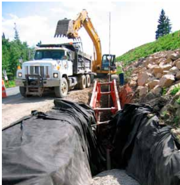
Figure 3-106—Construction of an underdrain with shoring (courtesy of FHWA).
