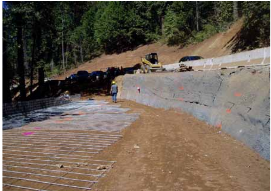
Figure 3-45—A slope stabilized with soil nails and a shotcrete face (stabilizing the excavation behind a welded wire wall under construction).
