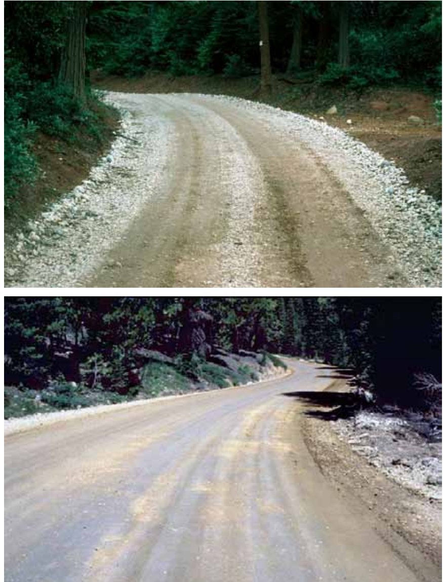
Figure 3-59—Gravel road surfaces that are reasonably firm and performing well.
