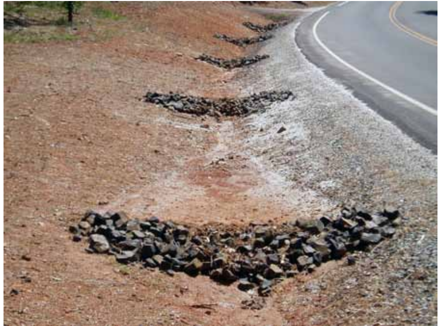
Figure 3-93—Rock check structures in the ditch (Oroville-Quincy Highway).
