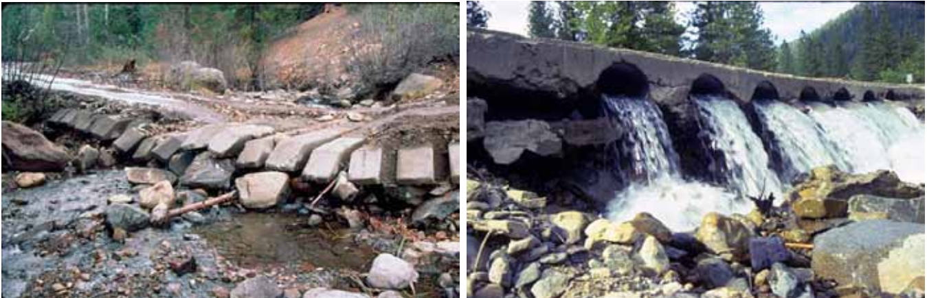
Figure 2-22—Low-water crossing structures damaged after a storm from scour moving materials beneath the concrete planks or concrete slab.
