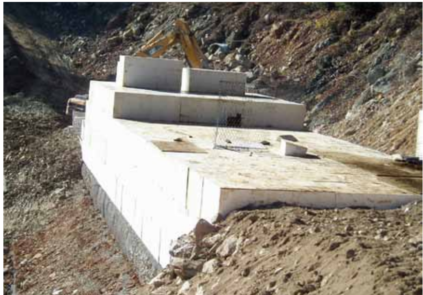
Figure 3-49—Geofoam wall under construction.
