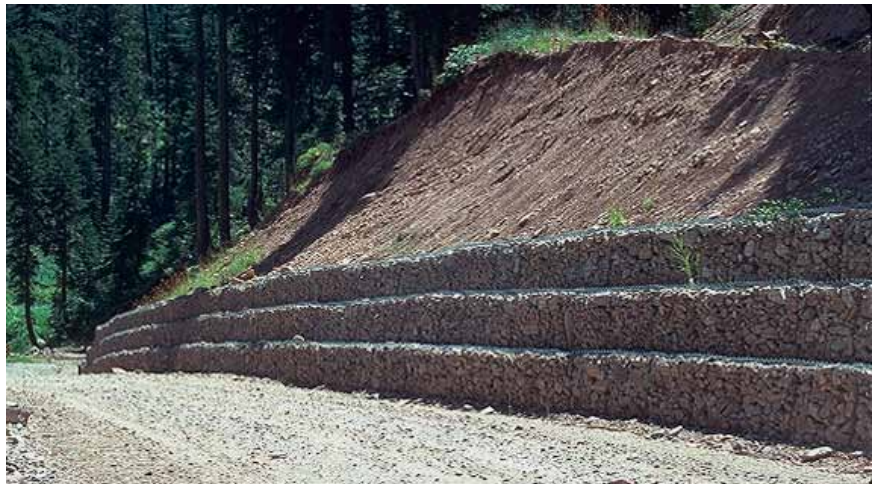
Figure 3-31—Gabions are a commonly used type of low gravity retaining structure because they use locally available rock and are relatively inexpensive.
