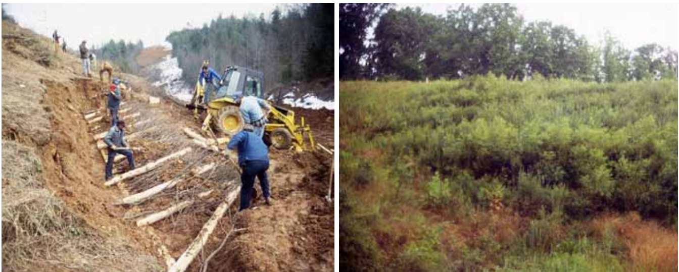
Figure 3-34—A live cribwall during construction and completed with sprouted vegetation (courtesy of Robbin B. Sotir & Associates, Inc.).
