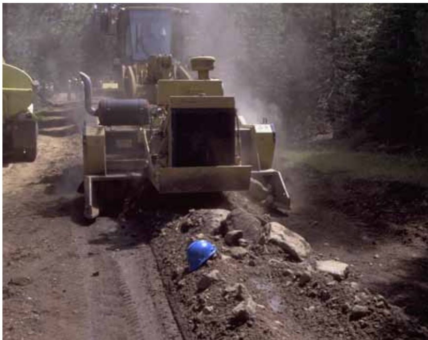
Figure 3-64—A mobile rock crusher processing a windrow of roadway material with boulders (Note hardhat for scale).
