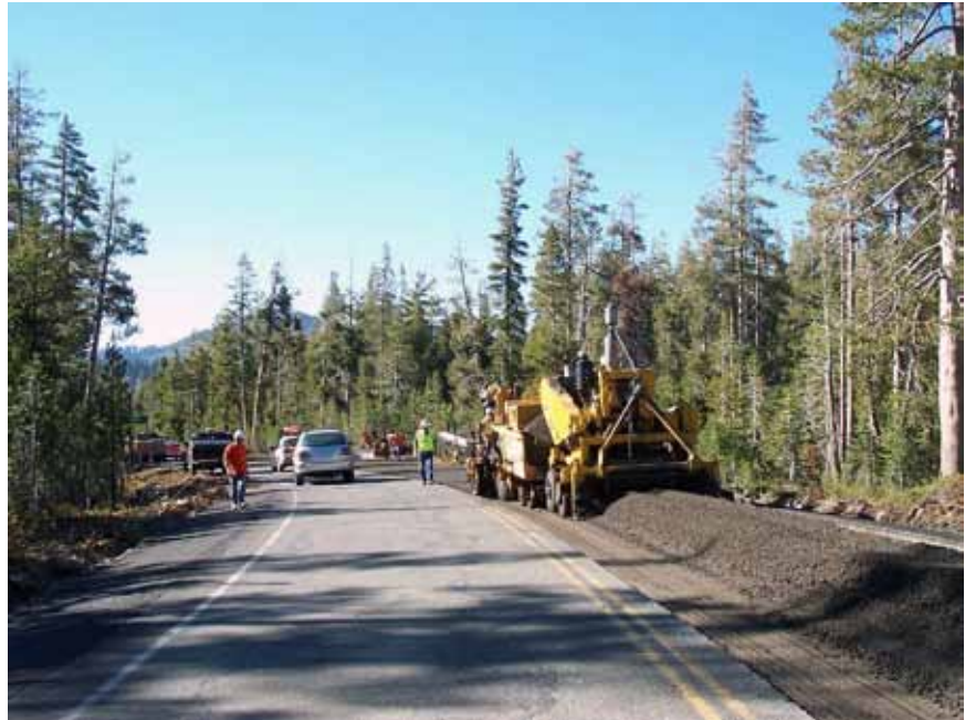
Figure 3-76—Milled asphalt being reused on a forest road.
