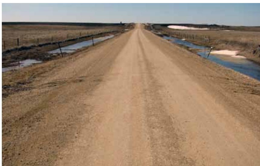
Figure 3-80—A gravel road with a 26-foot (9 m) driving surface, yet everyone drives in the middle. (Courtesy of South Dakota LTAP, Ken Skorseth)
