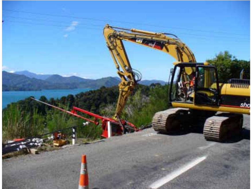
Figure 3-47—Installation of launched soil nails from the road (Courtesy of Bob Barrett).
