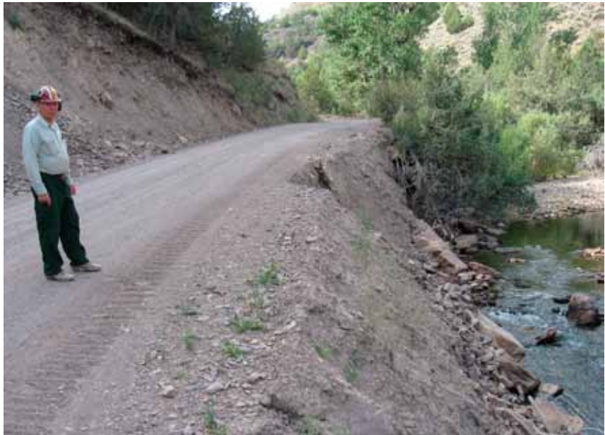
Figure 3-141—Steep and scoured fillslope extending into the river before reconstruction (courtesy of Mike Balen).
