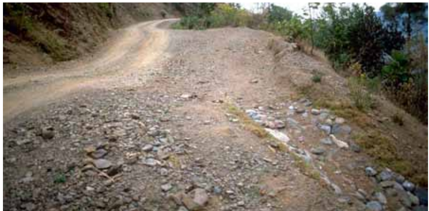
Figure 3-100—Rolling dip (broad-based dip) cross drains.
