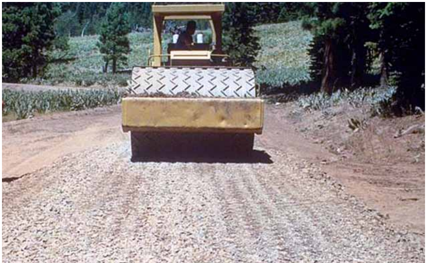
Figure 3-63—A soft volcanic rock broken down under an Elliott Grid Roller.
