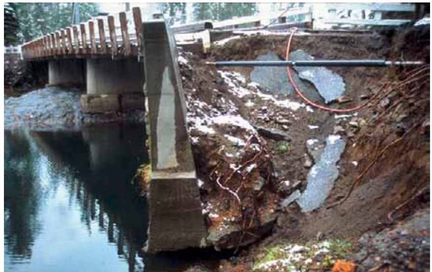
Figure 2-25—Bridge abutment undermined by scour.
