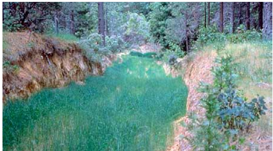
Figure 3-11—Vegetation (grasses) used to stabilize a closed road.
