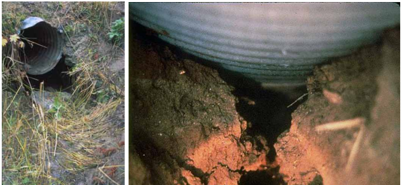
Figure 2-20—Piping failures underneath culverts.
