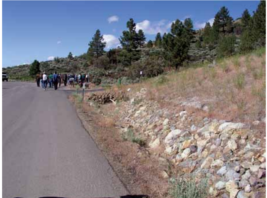
Figure 3-1—Relatively recent cutslope armored with rock and vegetated with native grasses.
