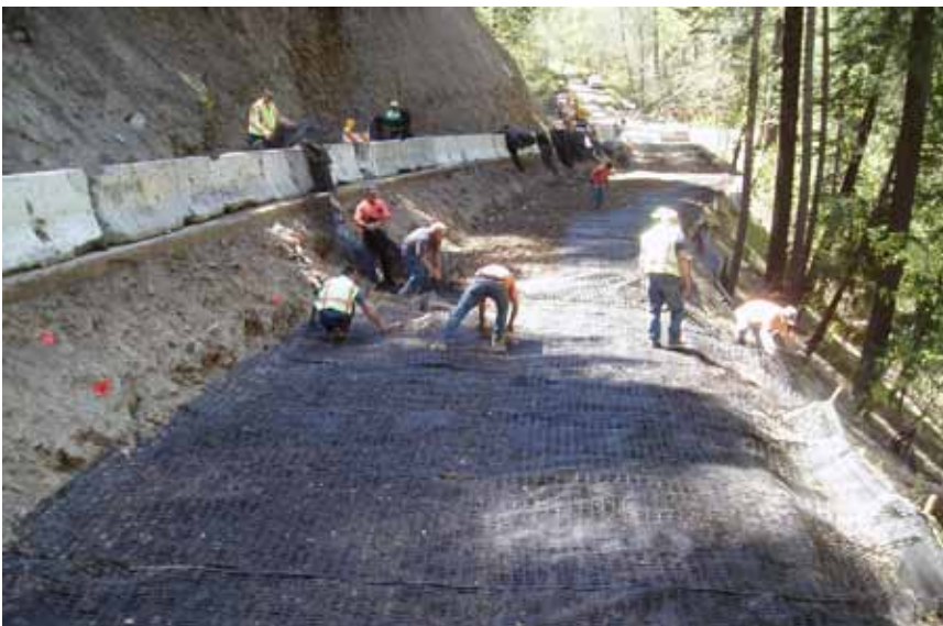
Figure 3-43—Geosynthetic reinforcing material (a geogrid) being placed in a deep patch shoulder repair.
