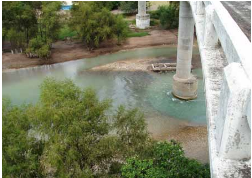
Figure 2-24—Bridge scour at a midchannel pier.
