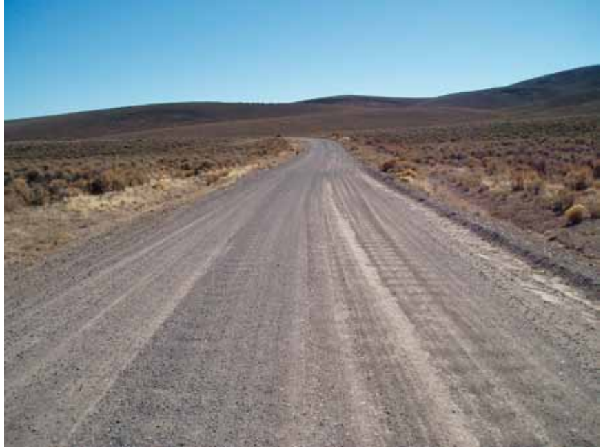
Figure 2-14—Washboarding forming in a gravel road surface.
