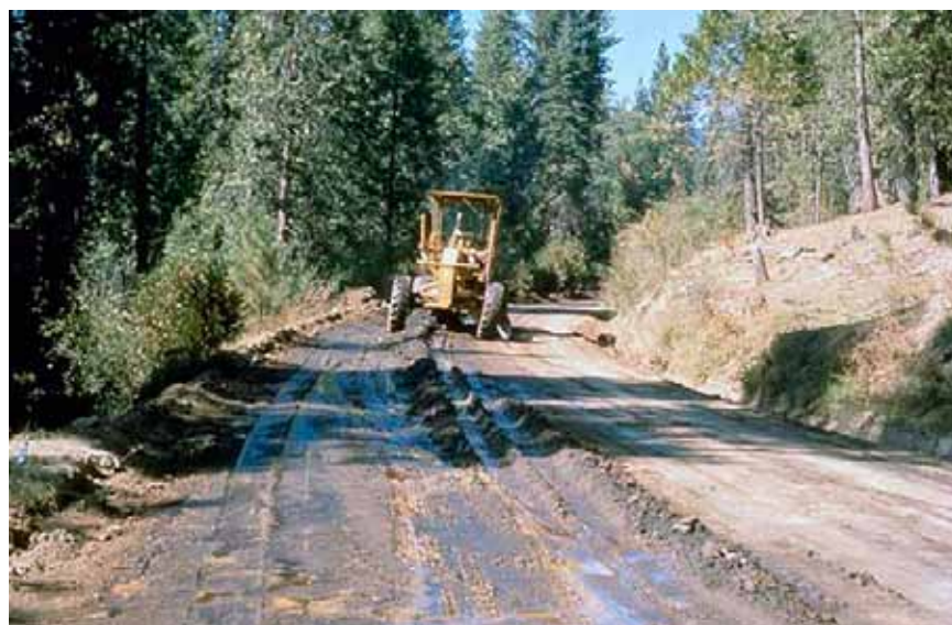
Figure 3-72—A dust palliative application being blade-mixed into a road surface.
