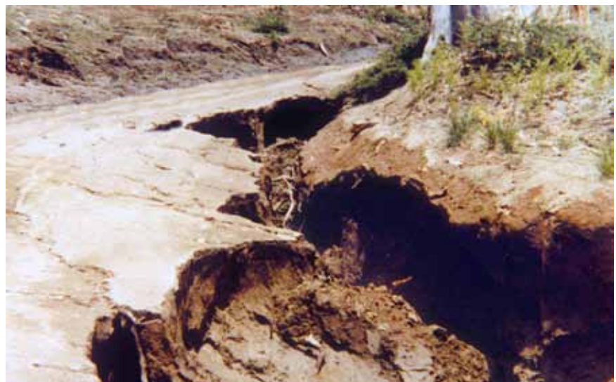
Figure 2-4—Typical gully erosion on a road.
