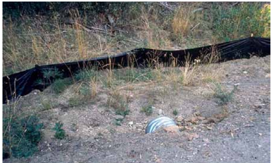
Figure 4-7—Geosynthetic silt fencing used to trap sediments and control erosion.
