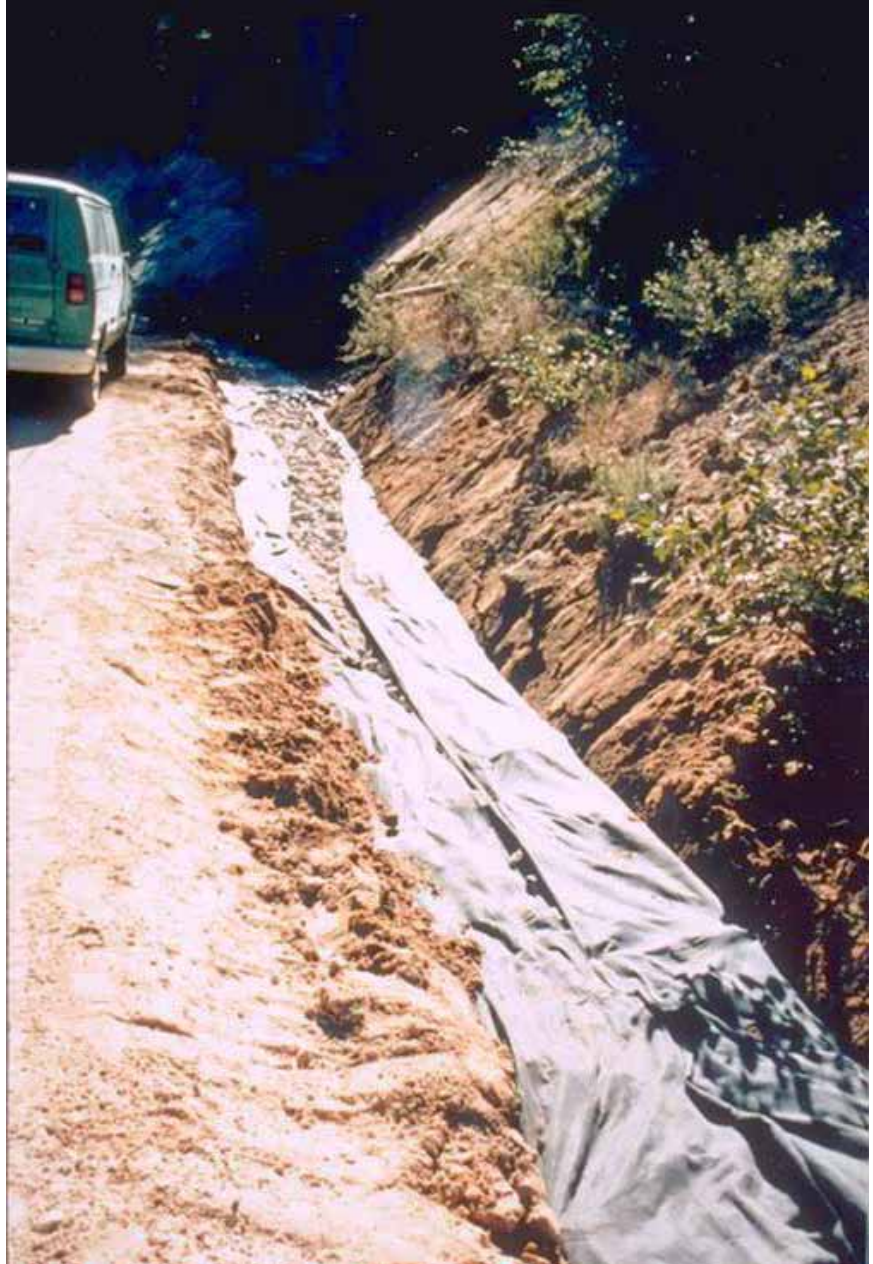
Figure 4-4—A geotextile wrapped underdrain for subsurface drainage.
