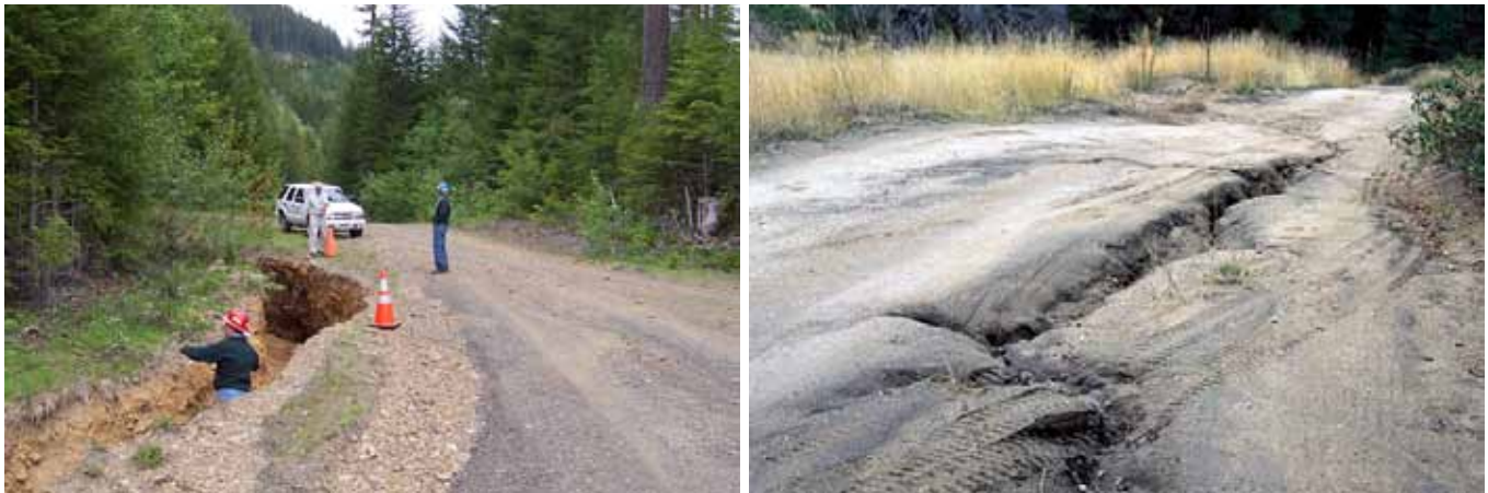
Figure 2-18—Examples of poor surface drainage causing erosion and damaging the road surface.
