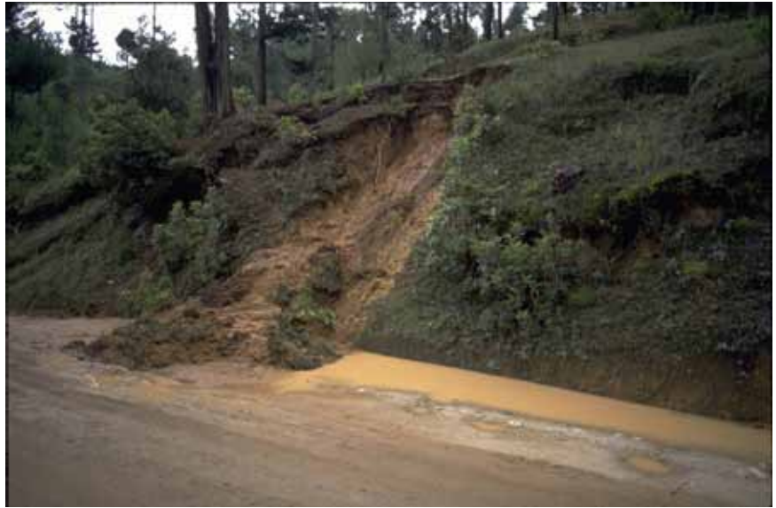
Figure 3-30—Oversteep slopes, wet areas, or existing slide areas can cause instability problems for a road and increase repair and maintenance costs, as well as sediment production.
