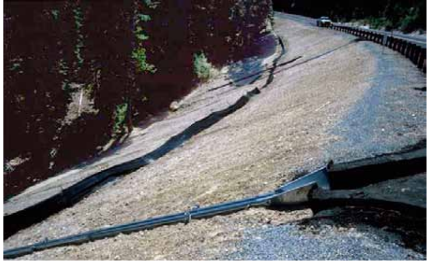
Figure 3-98—A downdrain used to move water to the toe of the fill.
