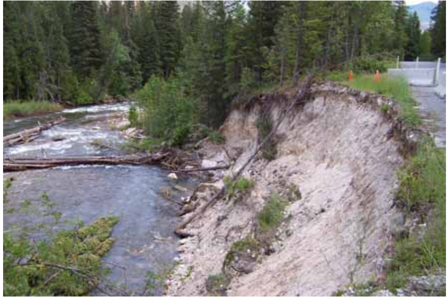
Figure 2-27—Streambank erosion.
