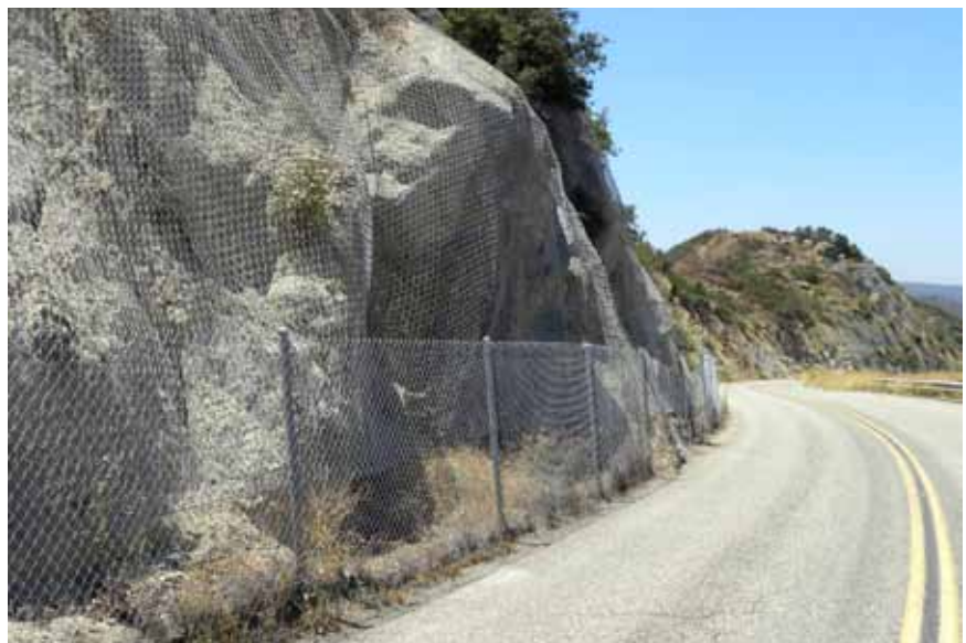
Figure 3-52—Rockfall prevention netting that traps rocks before they hit the highway.
