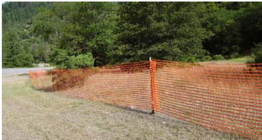
Figure 4-8—Geosynthetic fencing used for temporary protection of a sensitive site during construction.
