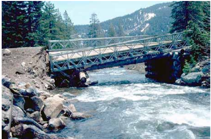
Figure 2-23—A bridge abutment washout due to contraction scour on a short span bridge (one-half of the span of the natural channel).
