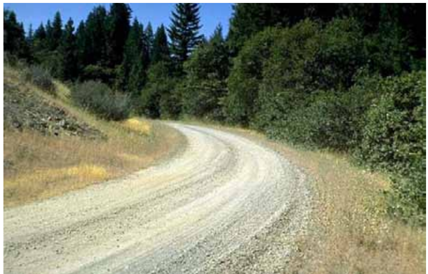
Figure 3-82—An outsloped single-lane road template, directing flow to and off the downhill shoulder.
