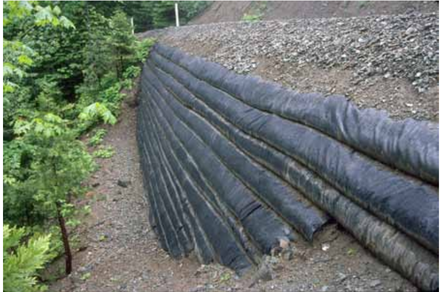
Figure 3-39—A geotextile wall constructed to support the roadway prism.
