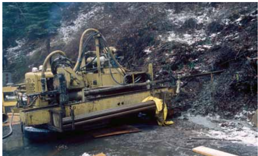
Figure 3-21—Horizontal drains being drilled to stabilize a landslide.
