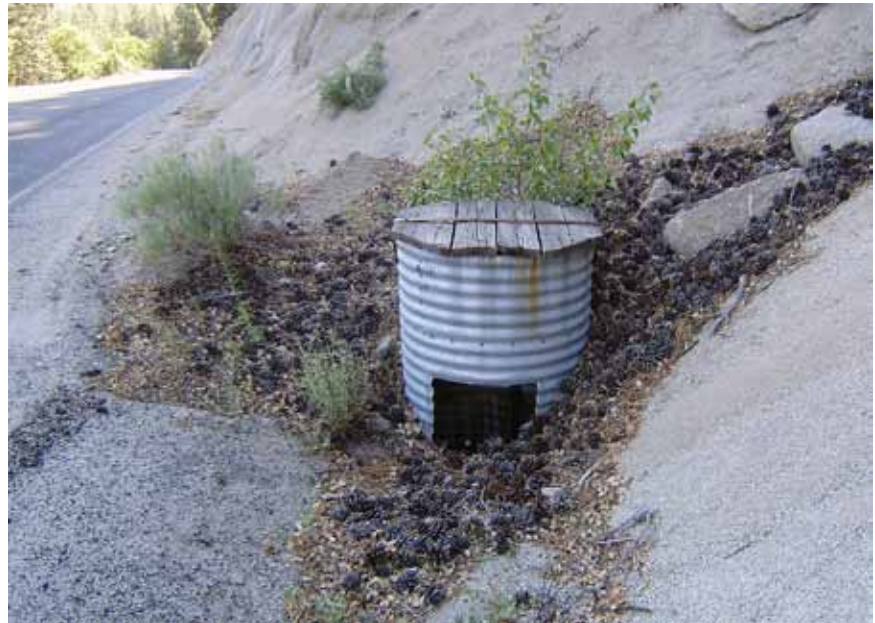
Figure 3-87—Typical drop inlet structure.
