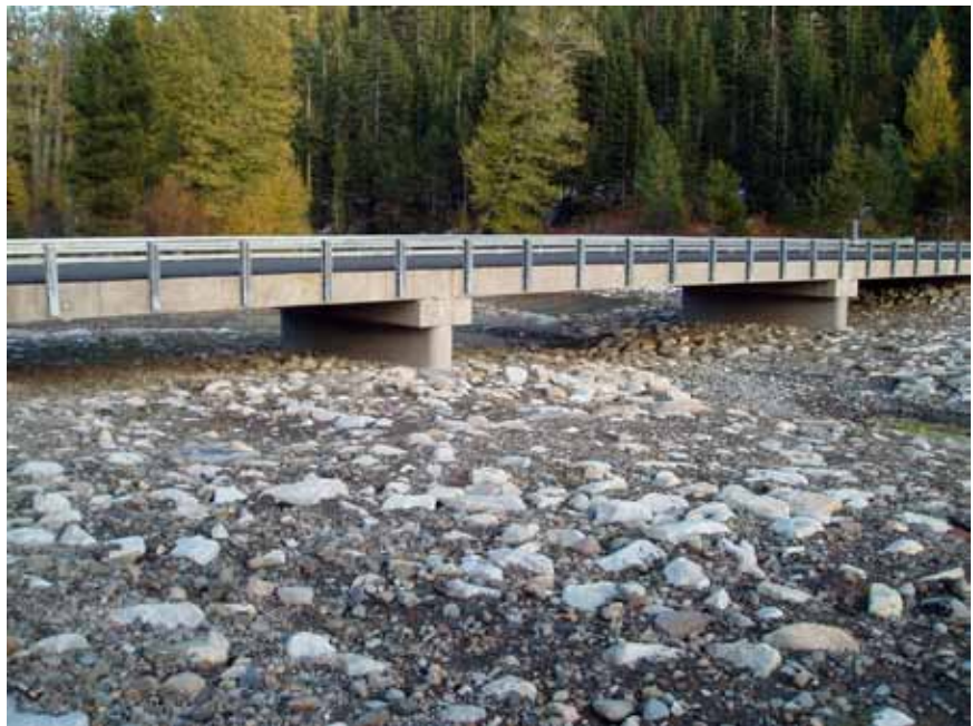
Figure 3-130—A concrete bridge that is durable and uses multiple spans to cross a broad flood plain.
