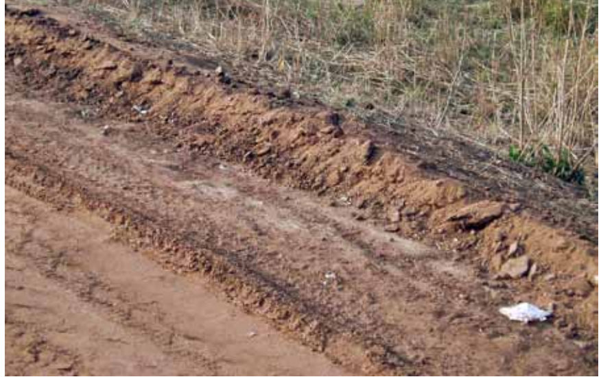
Figure 3-97—A berm formed at the edge of the road, typically by poor grader maintenance practices.
