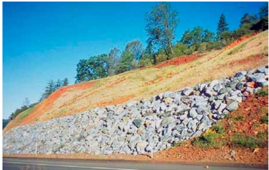
Figure 3-33—A drained rock buttress used to stabilize a cutslope failure.
