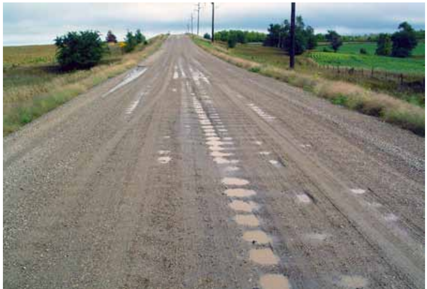
Figure 3-55—A road that lacks a good crown for surface drainage. There is centerline corrugation (washboarding), a problem that grows worse when there is inadequate crown or infrequent maintenance (Skorseth et al. 2000).
