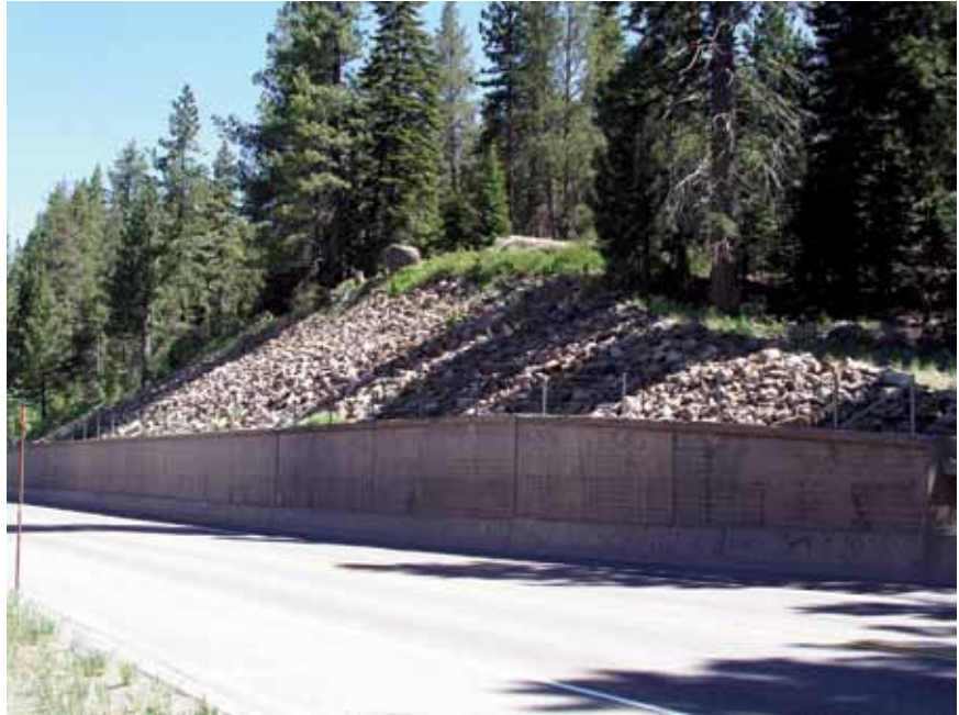
Figure 3-9—Riprap erosion protection on a cutslope above a retaining wall.
