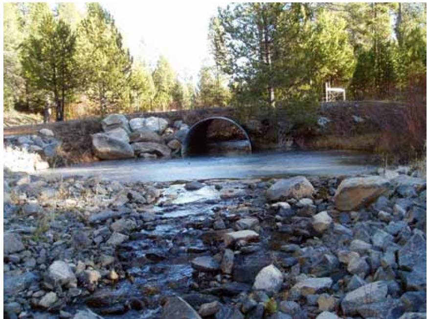
Figure 3-122—An old shotgun or perched pipe with water flooded back through the pipe for fish passage with use of a downstream elevated rock weir.
