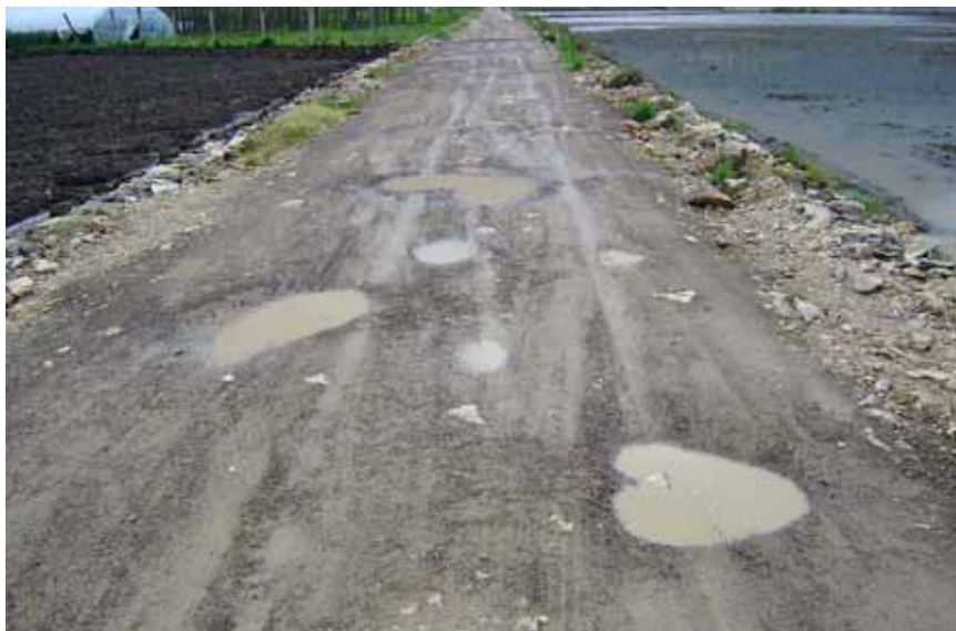
Figure 3-79—Potholes in the road surface pond water, weaken the roadway structural section, accelerate surface damage, and make driving difficult.
