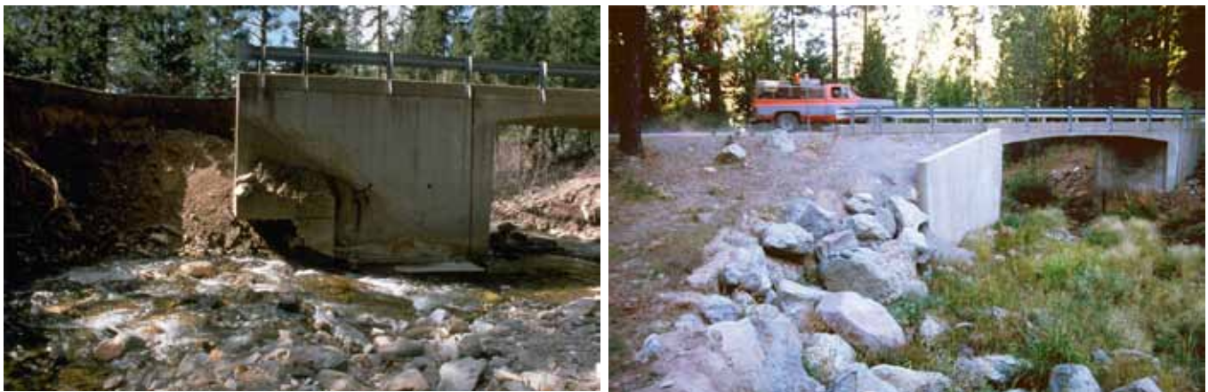
Figure 3-128—Scour due to lateral migration of the channel (left), and the repair (right) with streambank armor using a concrete wing wall and riprap. Scour is one of the most common causes of bridge failure.
