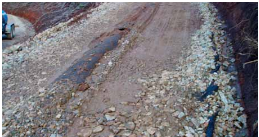
Figure 3-56—Geosynthetics and gravel placed over a local soft area in a road. Note that the geotextile is showing on the road surface so more cover aggregate is now needed.
