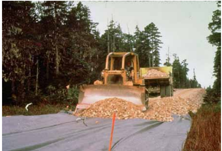
Figure 4-3—Geotextile used to separate aggregate from a weak subgrade.
