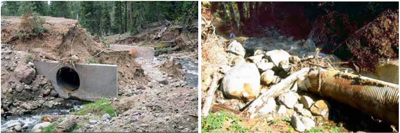
Figure 2-19—Failed culverts probably caused by plugging.
