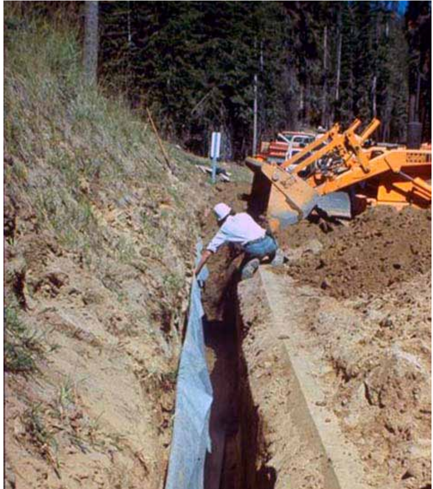
Figure 3-108—A geocomposite underdrain during installation.
