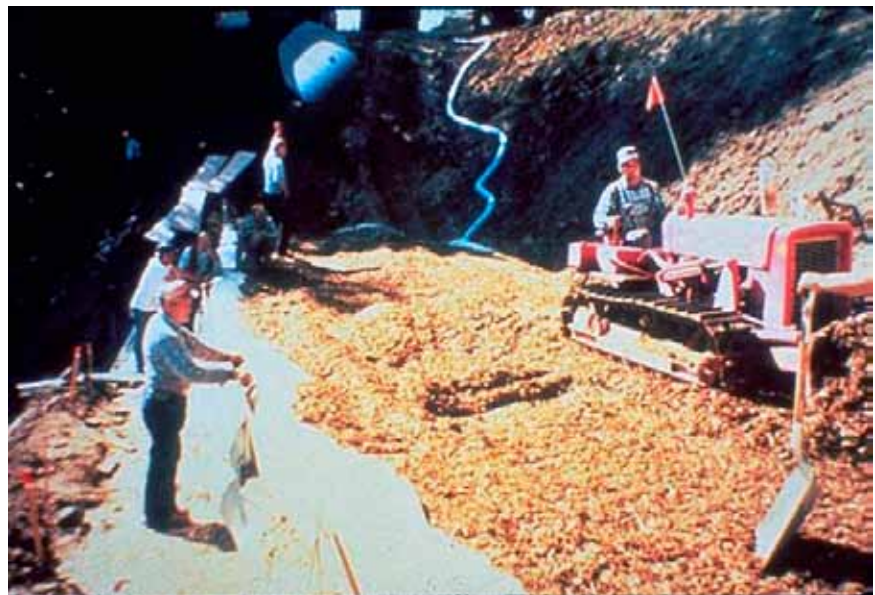
Figure 3-48—Lightweight wood chips in a MSE retaining wall.
