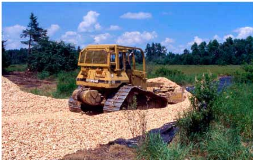
Figure 3-70—Wood aggregate (chunkwood) being used for temporary stabilization of a road surface over a soft, wet area.
