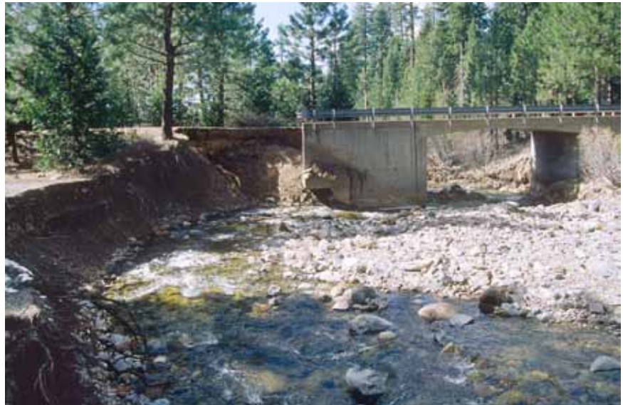
Figure 2-26—Abutment fill scour due to a shifting channel and streambank scour (with little damage to the bridge itself).
