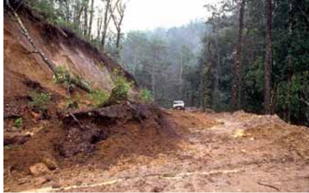
Figure 2-7—A cutslope slide closing the road.
