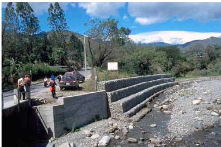
Figure 3-140—Gabions and concrete wall streambank protection at a bridge.
