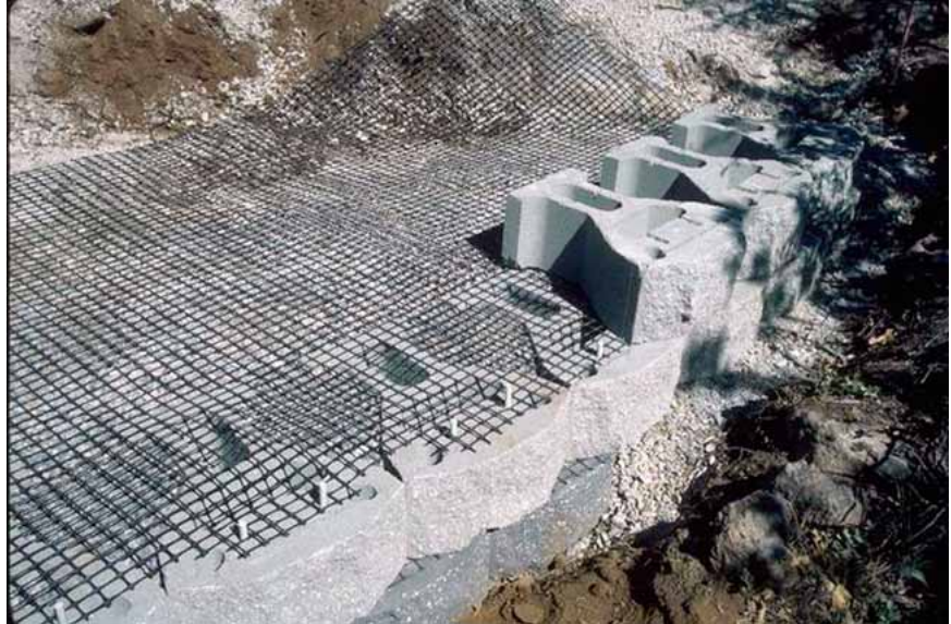
Figure 3-36—Concrete block-faced MSE wall under construction.
