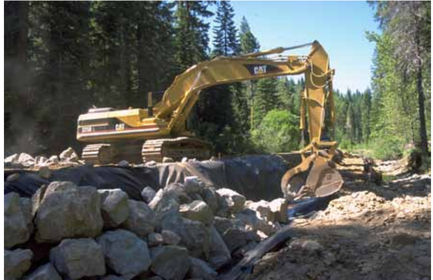
Figure 4-5—A geotextile used as a filter layer behind riprap.
