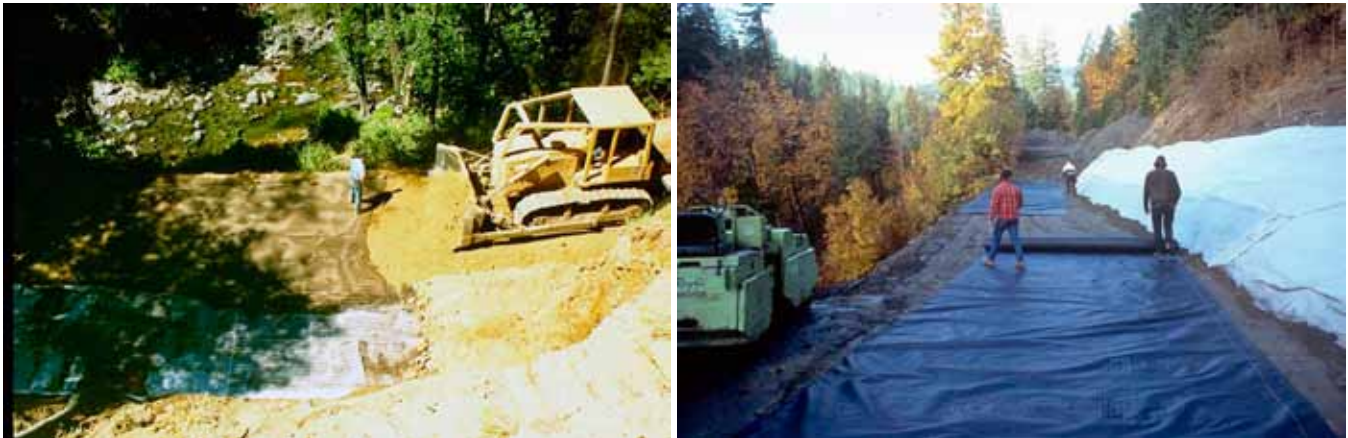
Figure 3-41—Construction of reinforced fills using layers of geogrid or geotextile.
