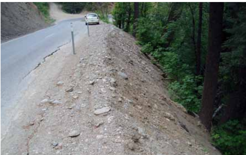
Figure 3-42—Oversteep settling fillslope before deep patch repair.
