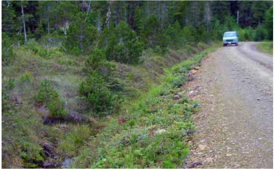
Figure 3-94—A vegetative-lined ditch.
