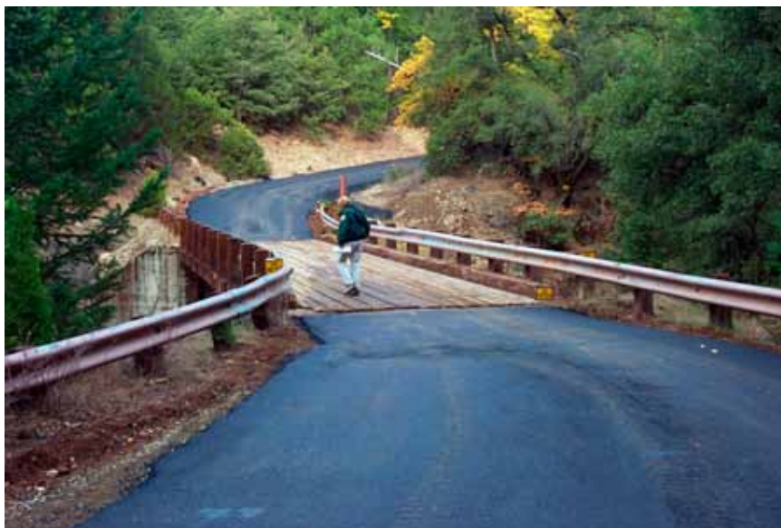
Figure 3-131—A bridge with paved bridge approaches to prevent sediment movement into the drainage.
