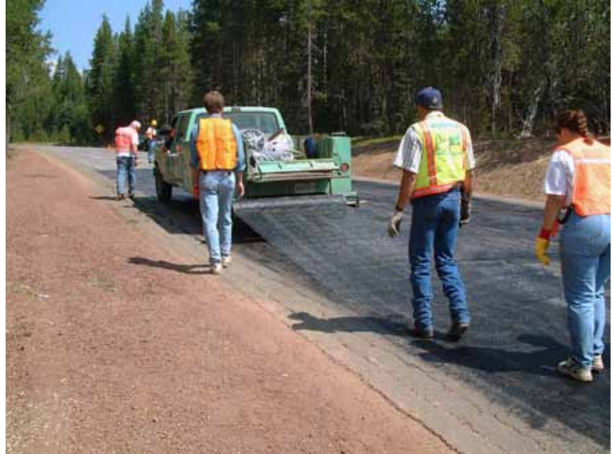
Figure 3-75—Placement of a high-strength, low-elongation paving geotextile prior to an asphalt overlay. Photo courtesy of Gordon Hanek.
