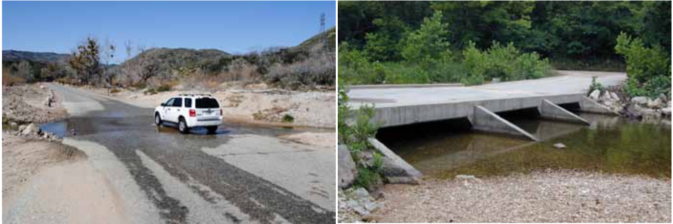
Figure 3-127—A simple concrete ford (left) and a vented ford (right), ideal for fish passage, both on low-volume roads.
