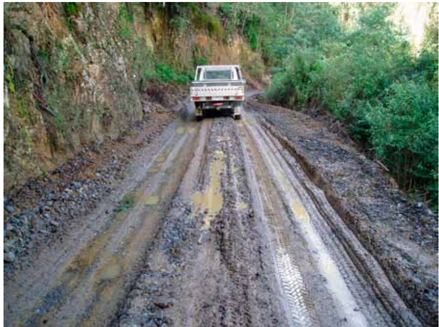
Figure 2-12—Ruts in soft soil road surfaces.
