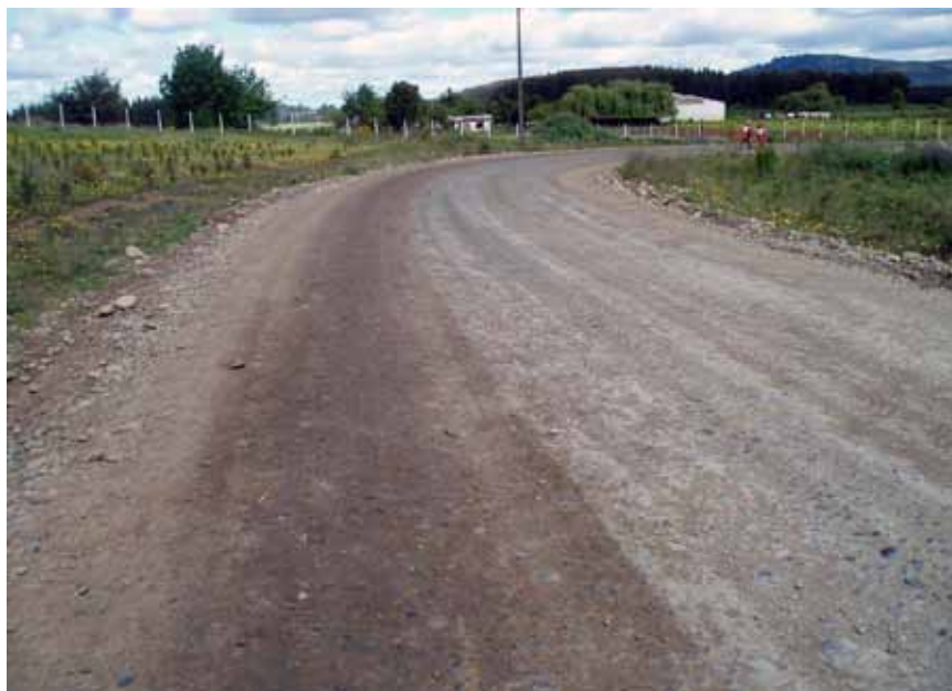
Figure 3-71—A calcium chloride dust palliative applied to a logging road.
