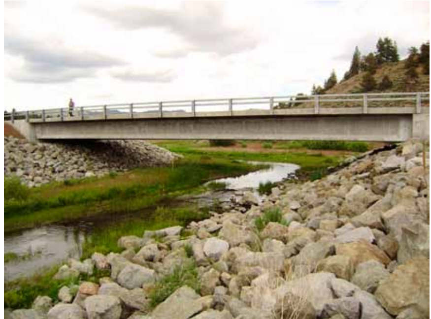
Figure 3-139—Large riprap armoring used for streambank protection through a bridge that is located near a bend in the creek.
