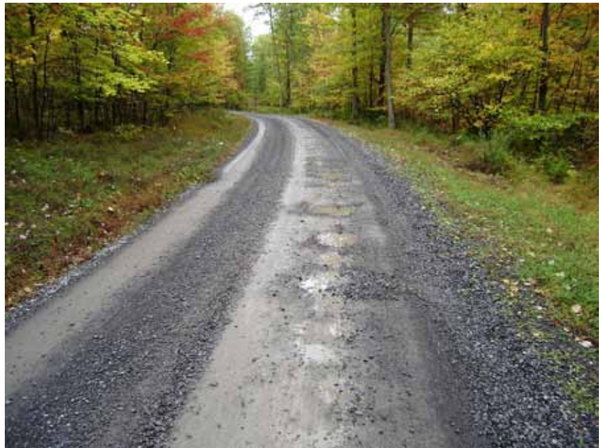
Figure 2-13—Potholes in the road surface. These potholes pond water, weaken the roadway structural section, accelerate surface damage, and make driving difficult.
