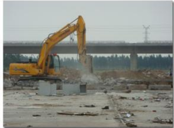
Ongoing Reclamation in Former Beam Factory
