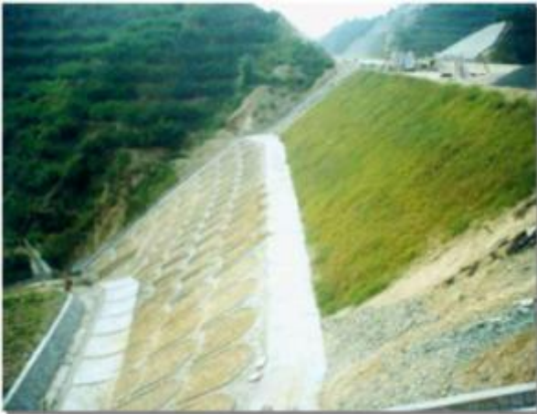
Slope Erosion and Protection Control
