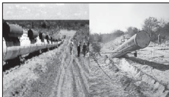
Figure 3. Conventional river crossing versus drilling under river beds for pipeline construction, Gasbol.
