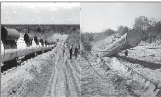
Conventional river crossing vs. directional boring under river beds for pipeline construction
