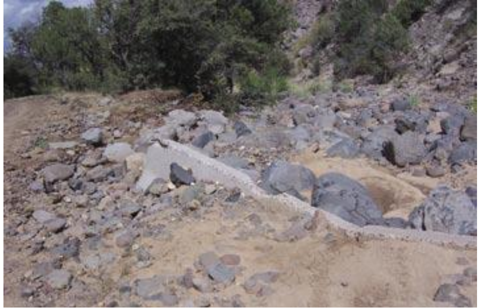
Figure A19. High flows have outflanked one of the ford structures.
