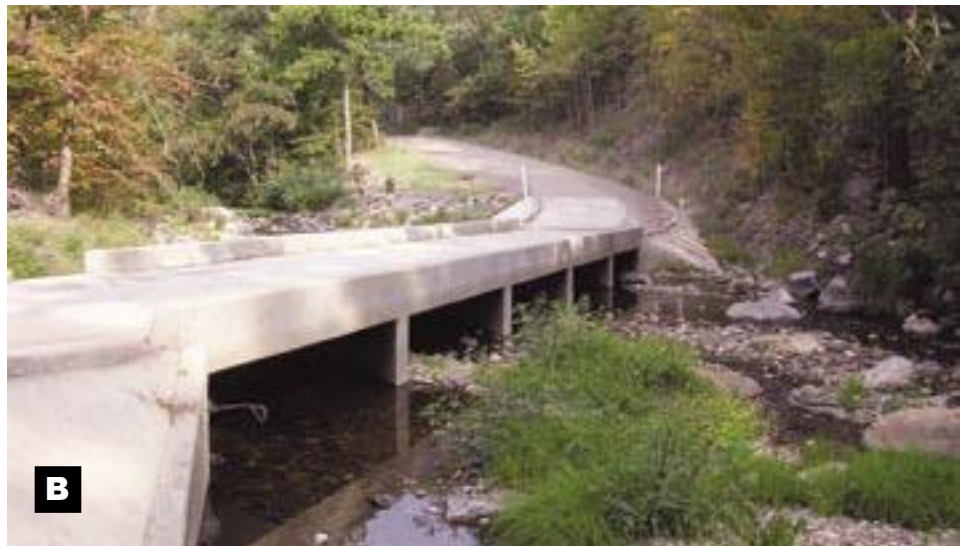
Figure 1.6—(A) Low-VAR ford on the Eldorado National Forest, Northern Sierra Nevada, California. (B) High-VAR ford on the Ouachita National Forest, Arkansas. Note that this site is on a curve and needs safety warning signs.
