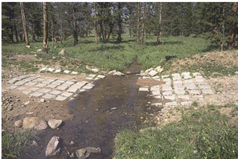
Figure A33. Copper Creek tributary, Bighorn National Forest. At this drier site with less traffic, the mat is considered the best crossing option because of its low maintenance requirement and installation cost.
