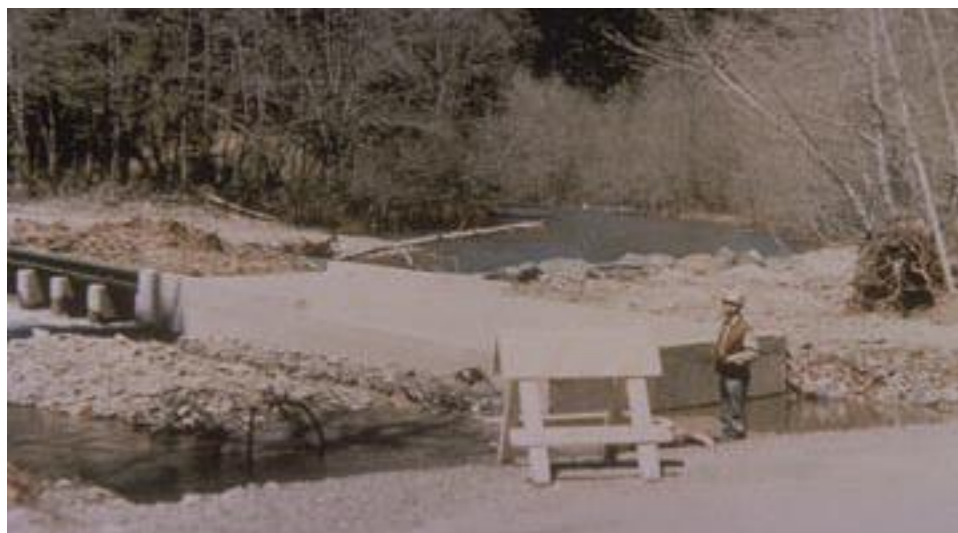
Figure A117. Scour around the east end of the structure after the 1986 flood. The concrete driving surface was then extended 50 feet.
