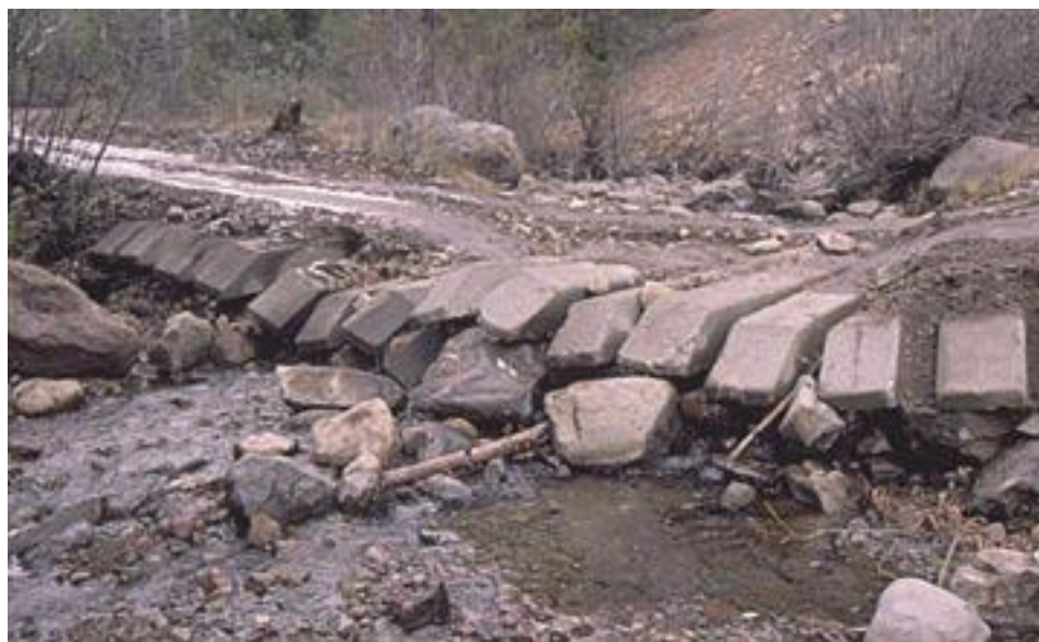
Figure A26. The crossing was damaged in the 1997 flood by scour of fine bedding materials under the planks. The planks had to be reset into coarser materials and the downstream edge protected with riprap.
