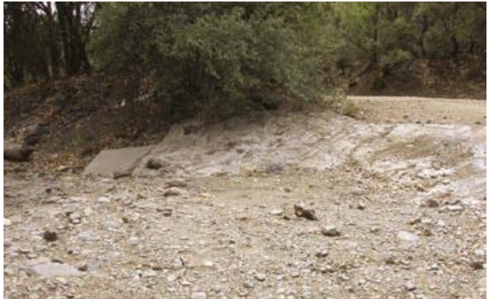
Figure A51. Concrete apron and grouted riprap prevent downstream scour and scour around edges of the ford.
