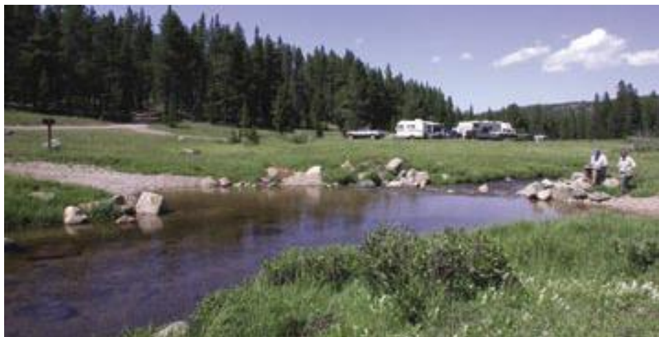
Figure A38. Soil compression on the approaches to the ford causes the stream to widen and lowers the elevation of the ends of the GEOWEB mat. Currently the geocell mat protects only part of the crossing during high flows.
