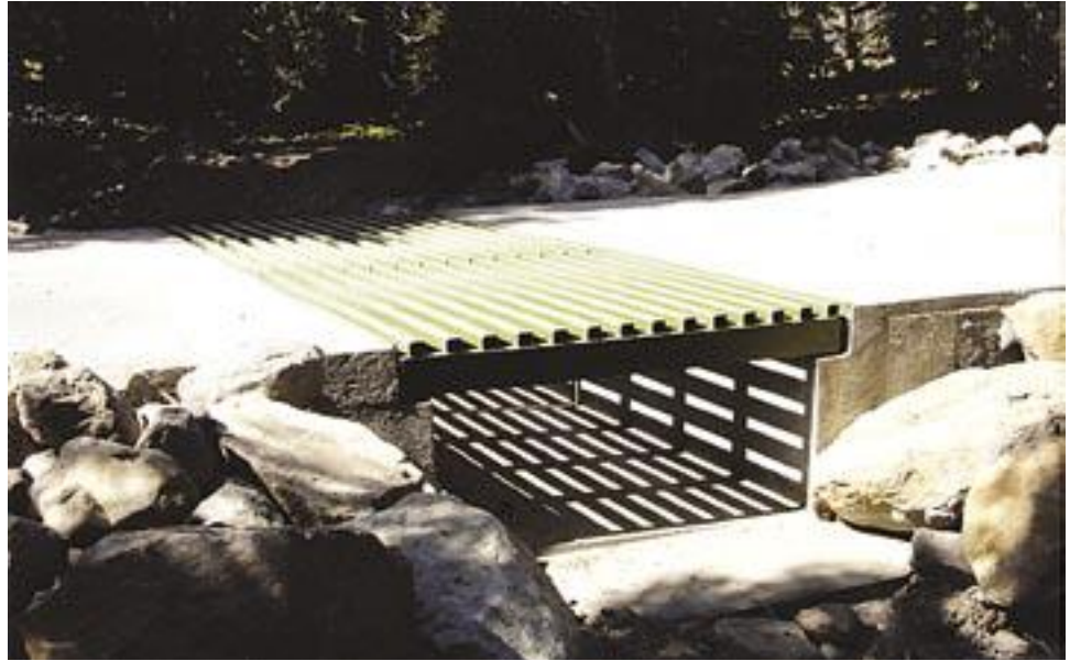
Figure A84. Close up of grated-top vented ford.
