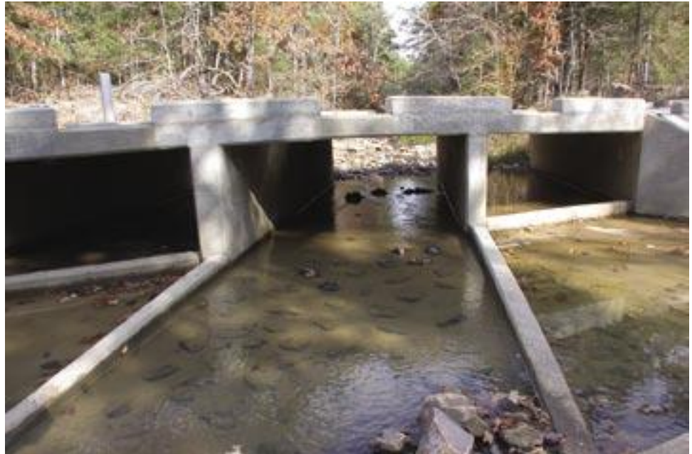
Figure A92. The floor of the central box has a thin veneer of sediment at low flow.
