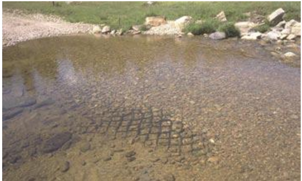
Figure 5.7—Geoweb installation on the South Fork Tongue River, Bighorn National Forest, Wyoming. Note exposure of geoweb due to traffic and water flow.
