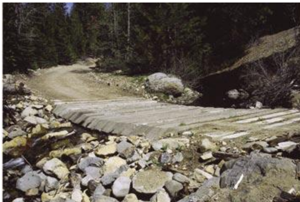
Figure A22. Willow Creek concrete plank ford.
