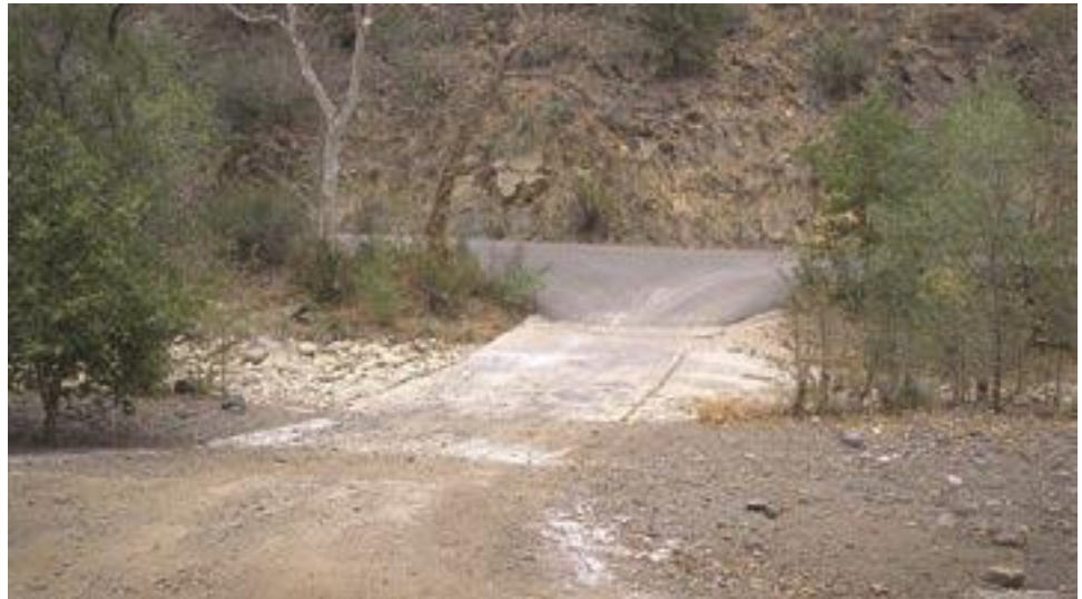
Figure 5.3—Old concrete slab ford with grout apron, Ashdale Administrative Site, Tonto National Forest. (case study 8)
