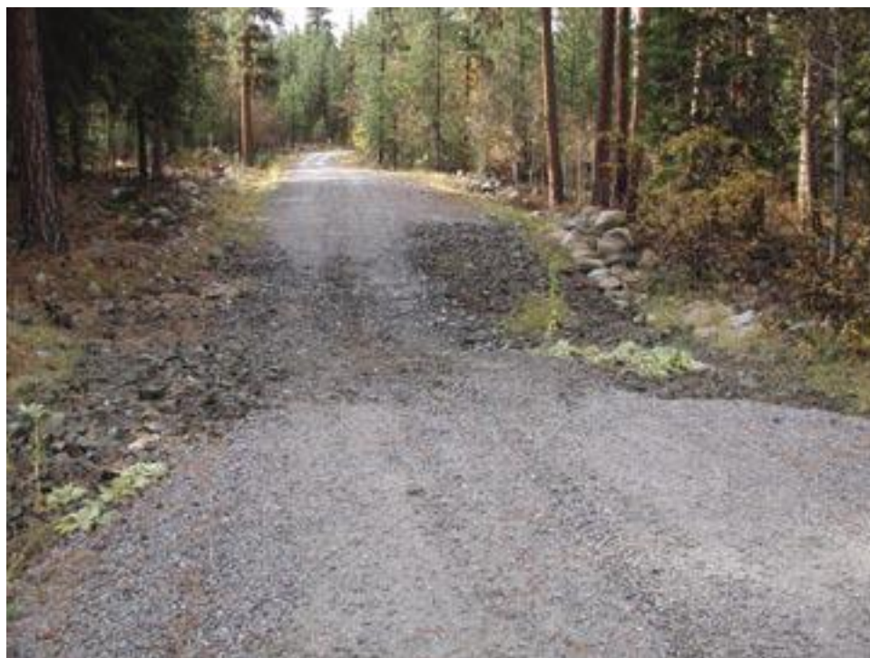
Figure A4. Hardened rock ford on East Chewuch Road.
