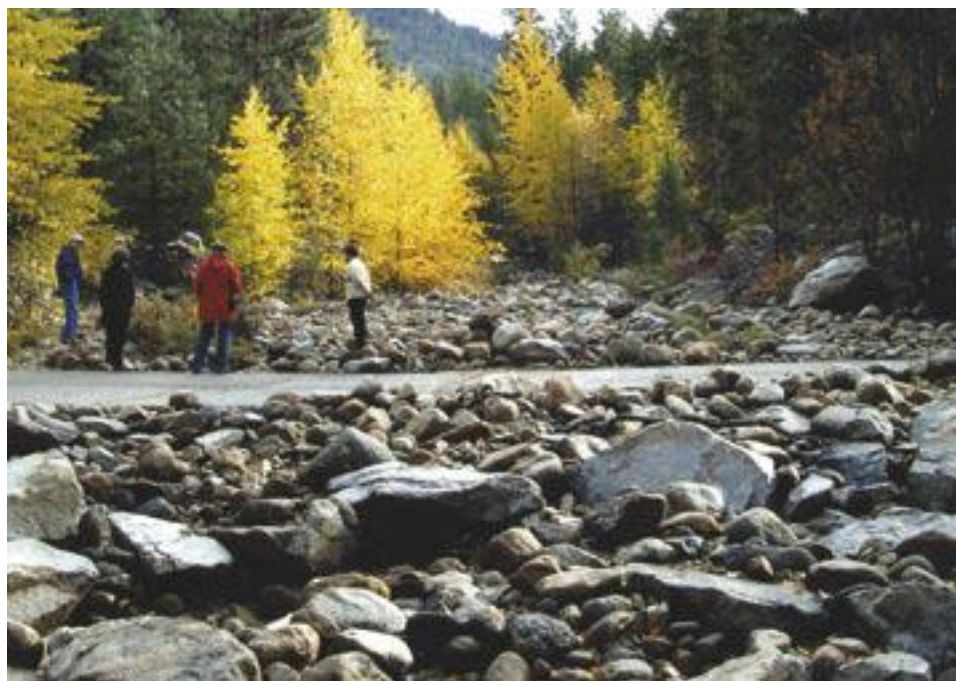
Figure A6—Vented ford plugged with boulders.
