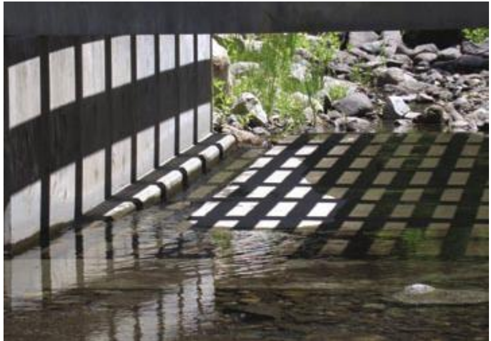
Figure A83. Vented ford showing low-flow trench at left and partial backwatering. Fish were attempting to move upstream in July 2002, but flow in the trench was too shallow and too fast.
