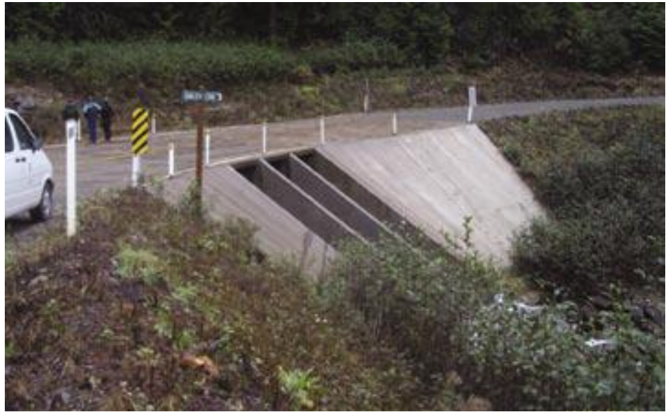
Figure A110. Safety markers on ford and approaches.
