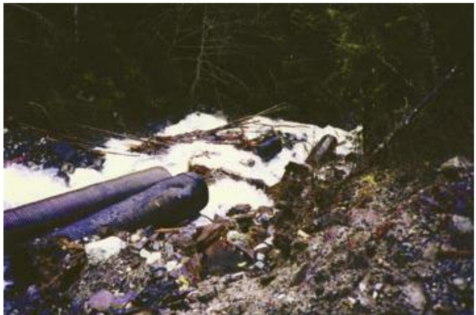
Figure A106. Two-culvert crossing on Sibley Creek blew out in November 1995.
