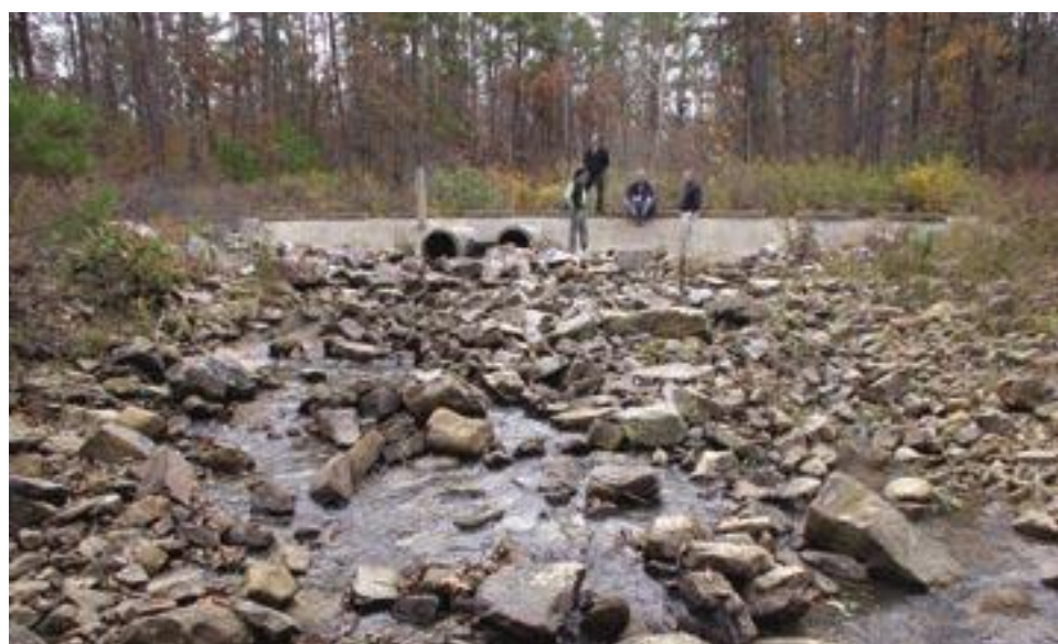
Figure A70. Lower Harris Creek concrete vented ford.
