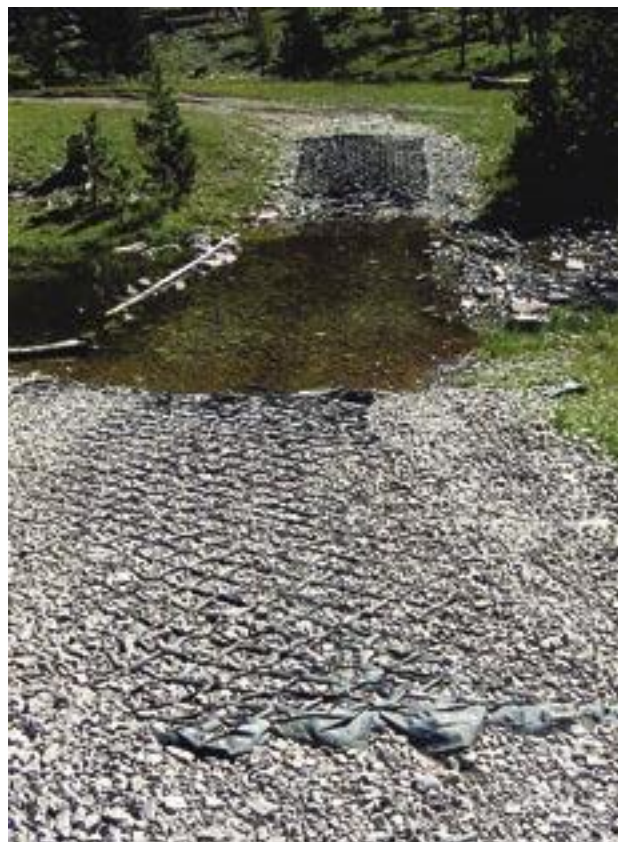
Figure 5.8—Geoweb exposed by tire action on road approaches, Ashley National Forest, Utah.
