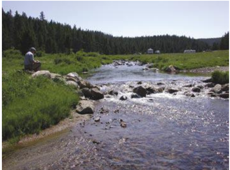
Figure A35. A boulder cascade was constructed at the downstream edge of the ford to control scour caused by placing the GEOWEB very slightly above streambed elevation.
