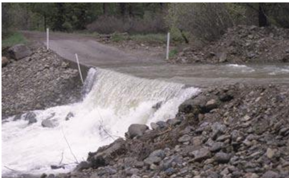
Figure A99. Damage to the Moonlight low-water crossing after the 1997 flood. The downstream rock armoring was undermined and washed away, partially undermining the concrete slab driving surface.
