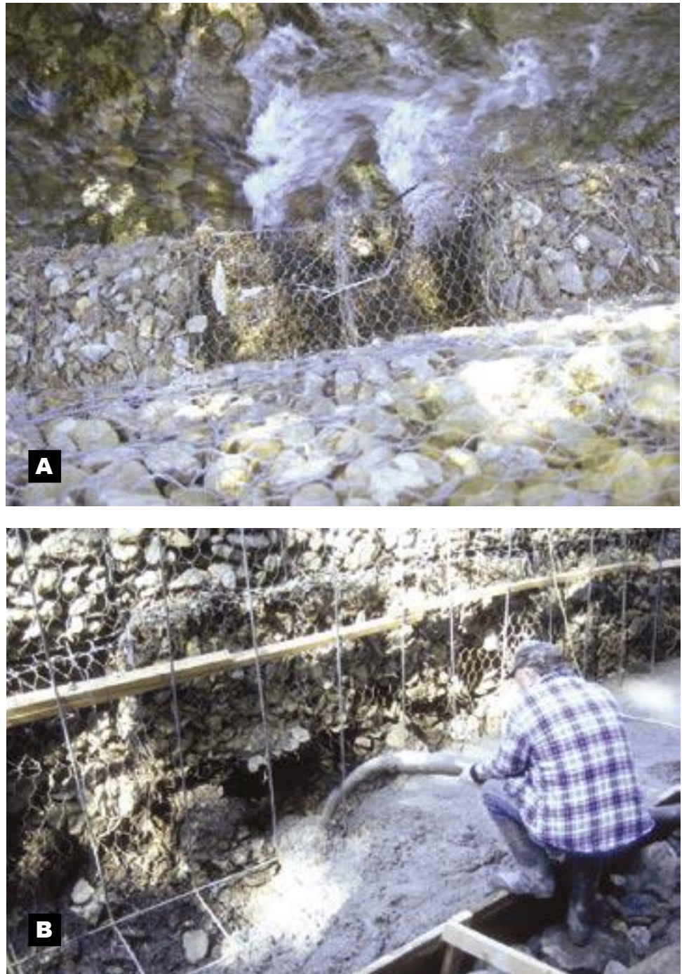
Figure 4.20—Gabion-basket failure and maintenance. a) Looking down at gabion baskets constructed to stabilize streambanks on Soda Creek, Plumas National Forest. Wire has rusted, allowing rock to wash away. b) To repair the stabilization structure, a concrete wall was poured in front of the damaged gabions.
