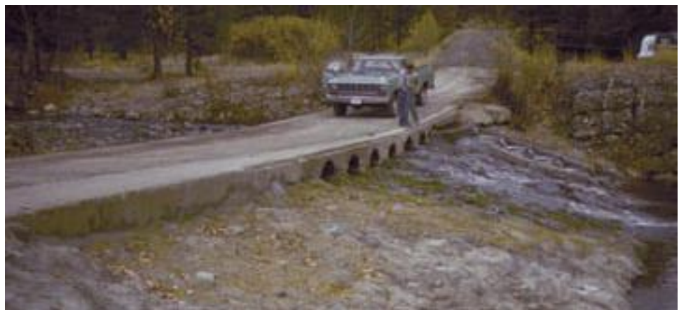
Figure A98. Moonlight Crossing prior to the 1997 flood. Note the weakly grouted small riprap armoring the downstream apron. There is no cutoff wall.
