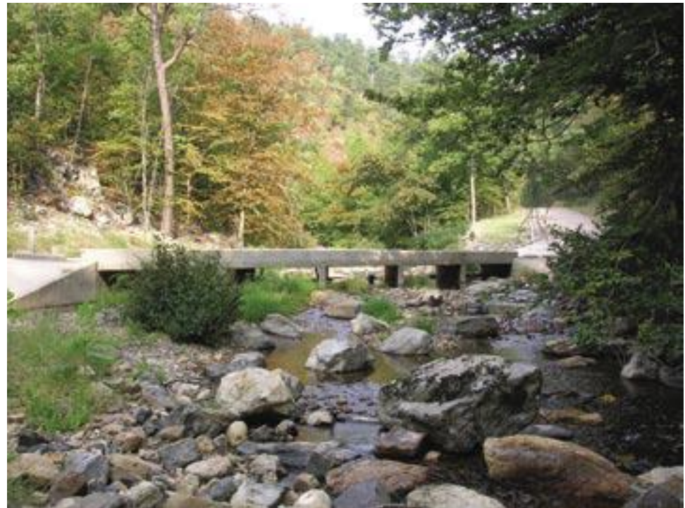
Figure A94. Looking upstream at the embedded box culverts that replaced the unvented ford in 2004.
