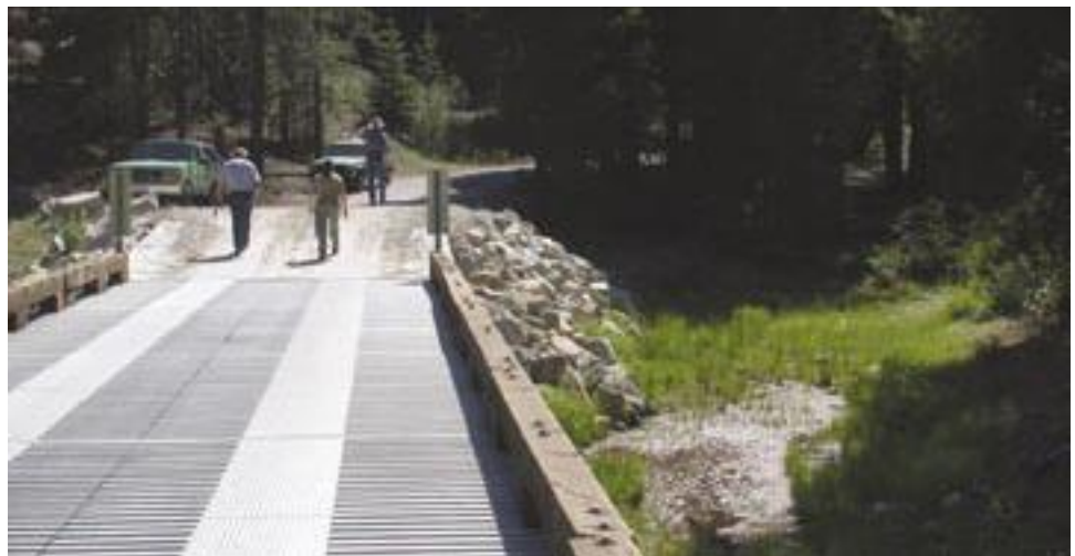
Figure A136. Note concrete abutment with riprap, grating with tire runways, and wood curbs.
