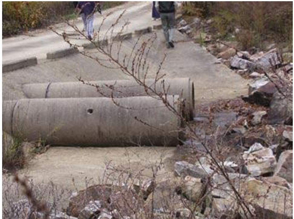
Figure A72. Concrete pipes outlet on splash apron with riprap downstream. Fillslope is also protected by concrete. Note erosion to side of fillslope concrete armor.
