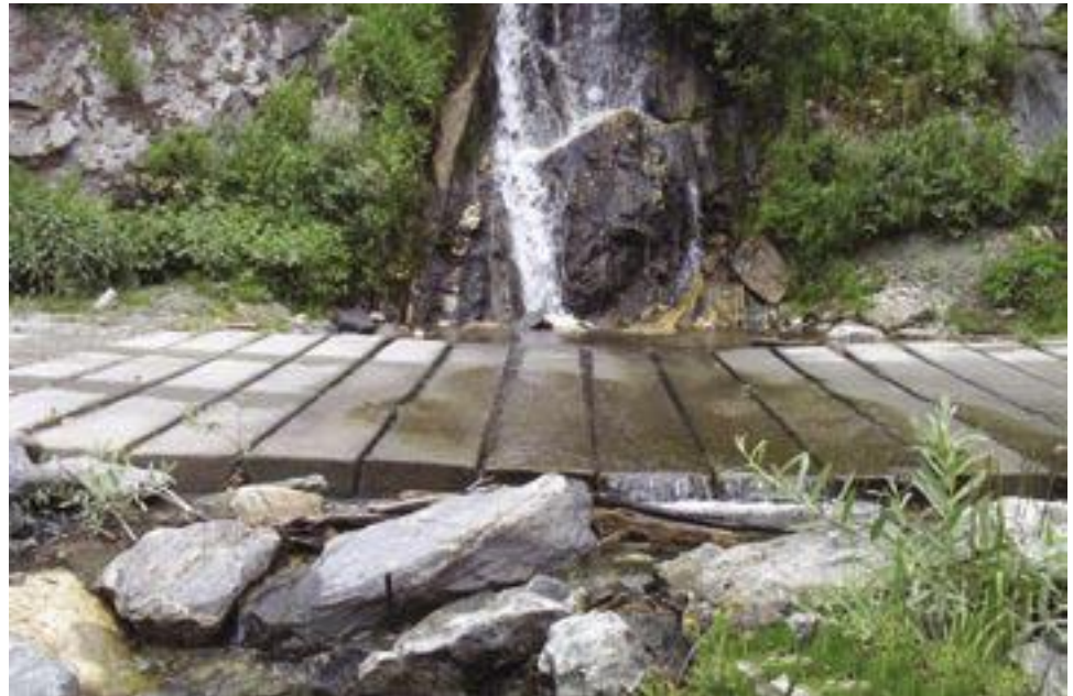
Figure 5.5—Concrete plank ford at edge of the North Fork Clearwater River, Clearwater National Forest, Idaho.
