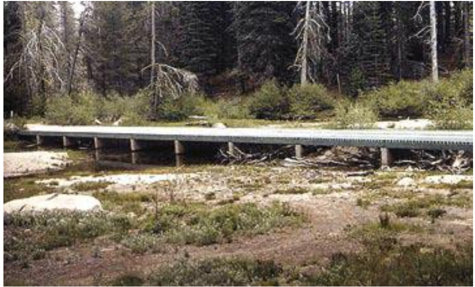
Figure A137. Looking downstream at Capps bridge with debris trapped under deck, 1988.
