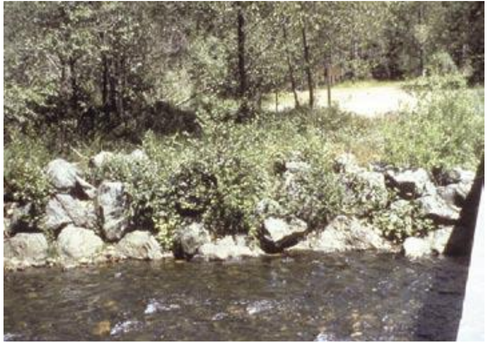
Figure 4.17—Large riprap with vegetation used for streambank stabilization, French Creek Crossing, Plumas National Forest.
