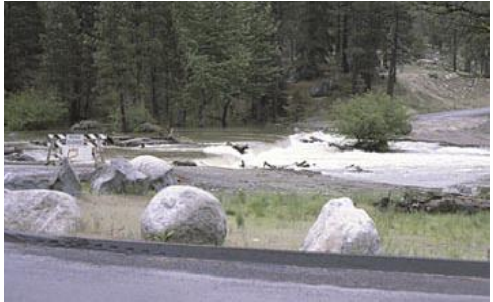
Figure A66. Crossing during a flood event. It is clearly not passable at this time. Note the amount of energy and “scour power” where the flow drops several feet over the structure.
