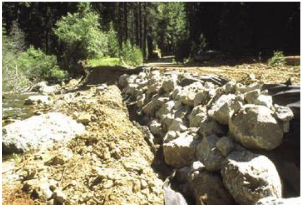
Figure 4.14—Poplar Creek riprap streambank stabilization structure under construction, Plumas National Forest, 1998. The geotextile prevents erosion of fine soil through the voids in the riprap.
