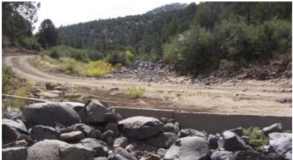
Figure A17. Looking upstream across another jersey barrier ford on FR 732. Sloped road approaches prevent diversion and large rock is placed downstream to prevent scour.
