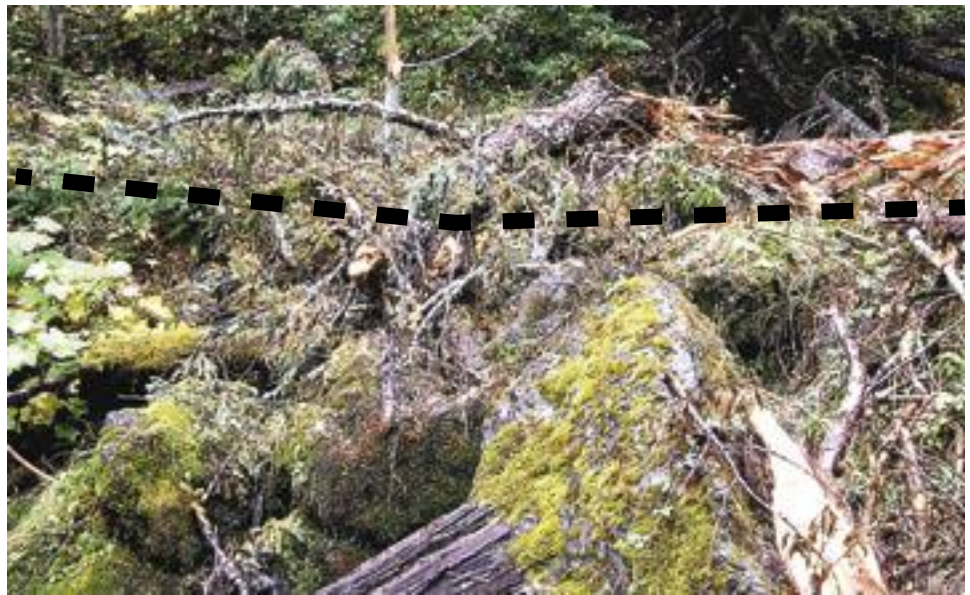
Figure A13. Stable, moss-covered rocks on the splash apron with pieces of fallen snag. Dashed line indicates approximate road surface.
