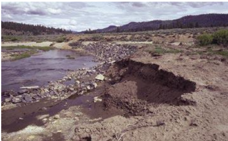
Figure 4.16—Looking downstream at a failed riprap installation on Red Clover Creek, Plumas National Forest.
