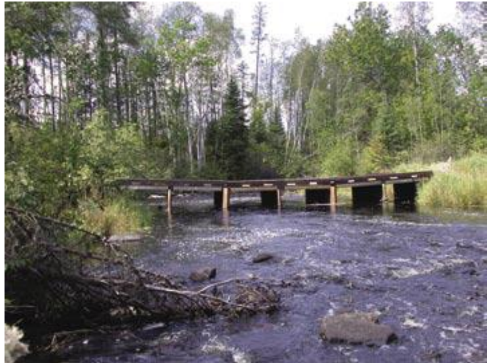
Figure A112. Stony River box culvert ford.
