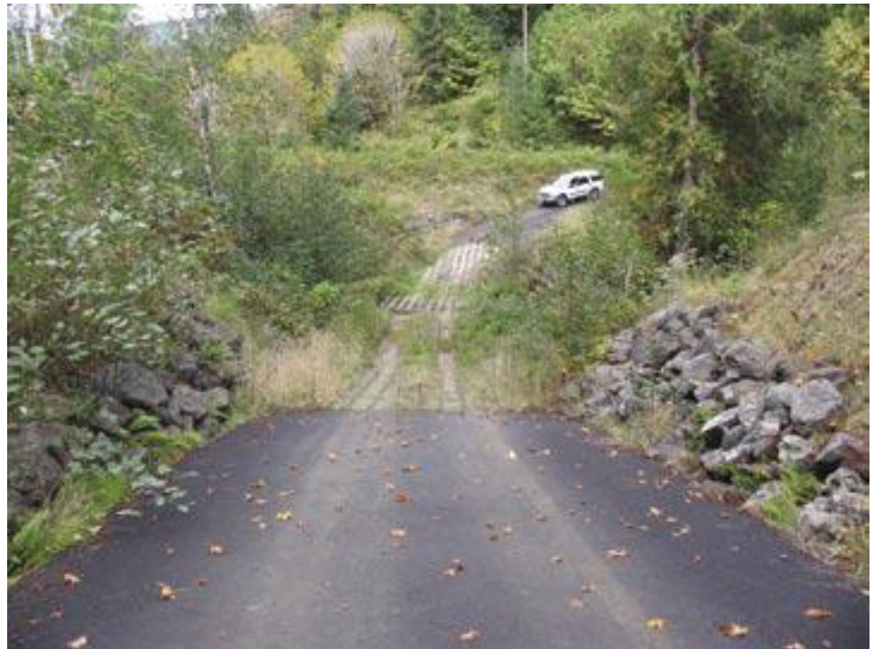
Figure A27. Fitzpatrick cable concrete mat ford.
