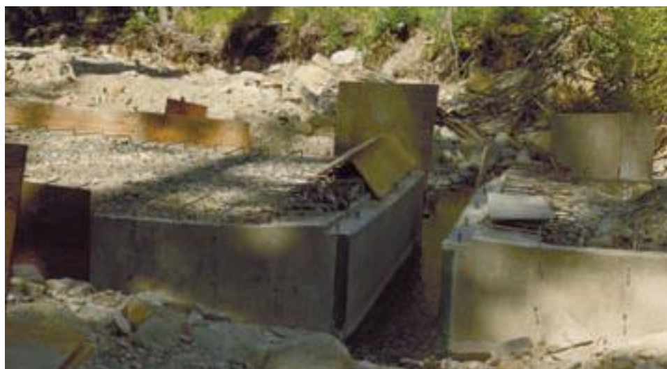
Figure A76. A 3-foot wide gap left between the two sides of the ford forms a narrow concrete-floored vent.
