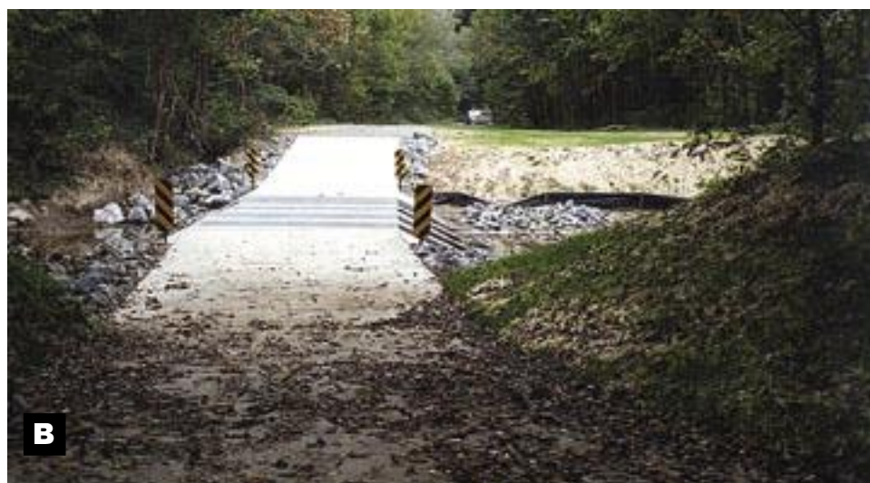
Figures A126a and A126b. Kinkaid crossing just after construction in 2001. A126a. Close up of embedded boxes; A126b. View along vented ford showing riprap.
