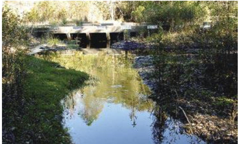
Figure A131. Sand and silt deposit downstream of the bridge (2003).
