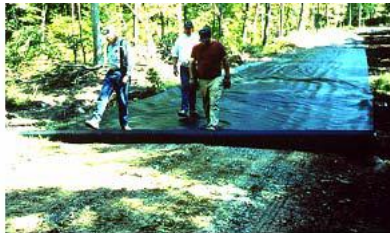
↑ Rolling out the fabric ↑
