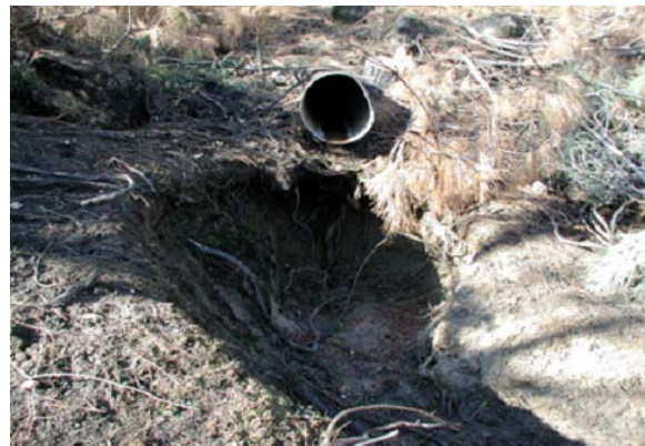
ESMP#8-01 Severe erosion at a pipe outlet.
