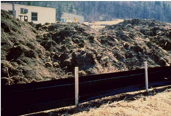
5-06 This installation will not control much sediment!
