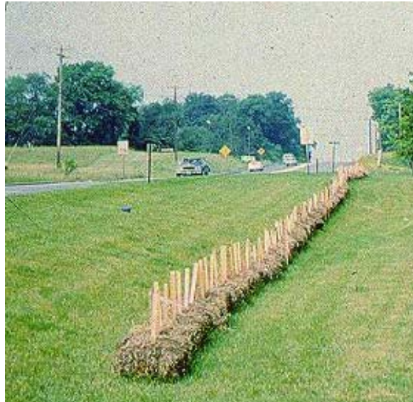
5-04 Proper bale installation prior to start of a major construction project. (Note: Bale barriers not recommended by EPA.)
