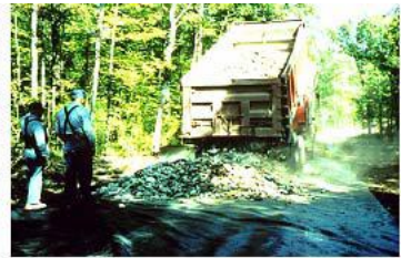
↑ Backdumping the ↑ aggregate
