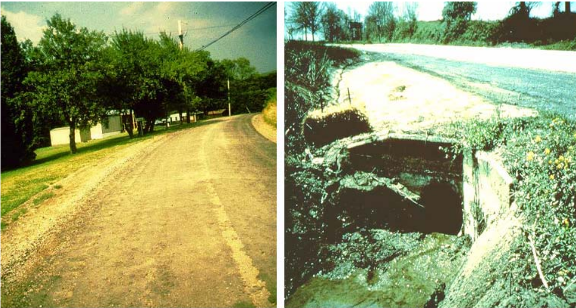
7-09 With the use of asphalt “oils,” tracking and/or run-off can become problems.
