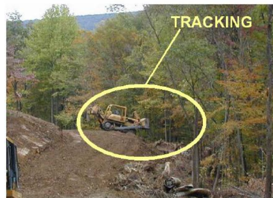
6-30 Tracking the newly constructed banks.
