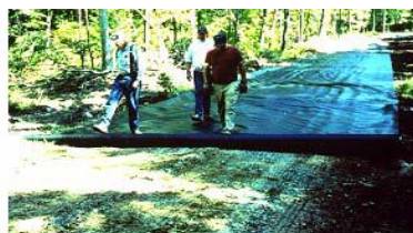
↑ Rolling out the fabric ↑
