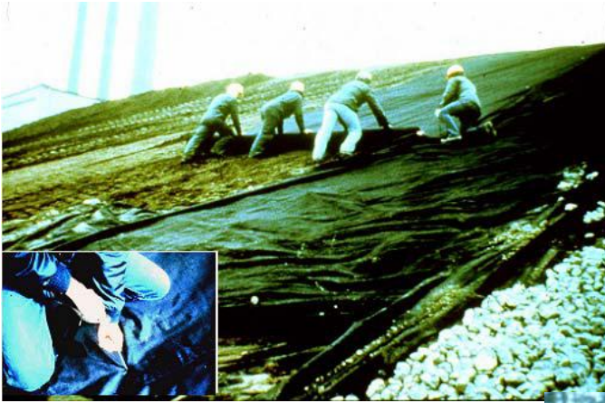
7-24 Installation of an erosion control fabric.
