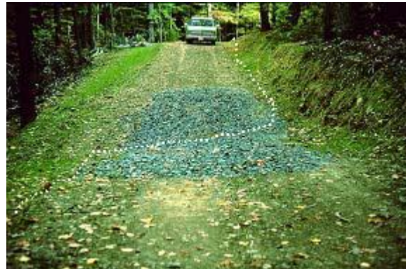
5-23 Broad based dip reinforced with large aggregate.
