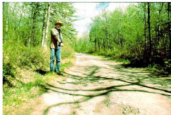
5-01 Typical entrenched eroded road.
