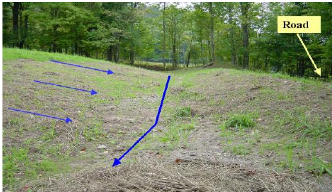
ESMP#13-02 Diversion Swale: Wider swales and gradual slopes result in more infiltration and less water volume to handle.
