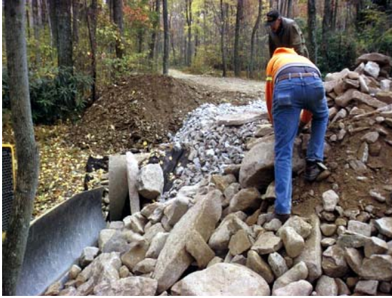
A7-08 Placing large size riprap at ends of pipe.
