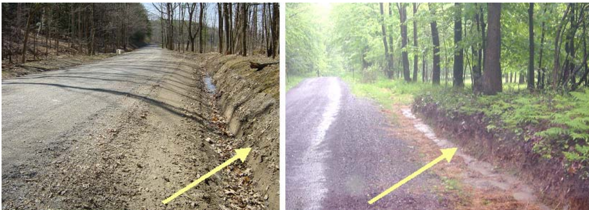
6-25 Unstable vertical bank will collapse.
