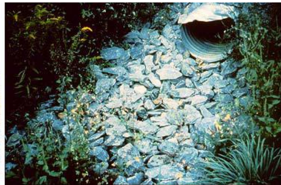
5-37 Rock rip-rap at pipe outlets spreads flow and dissipates energy.
