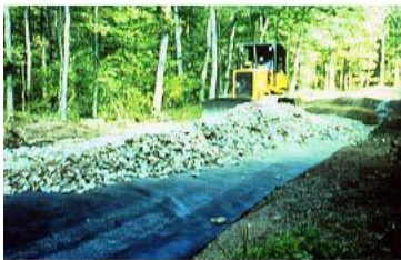
↑ Spreading the aggregate ↑
