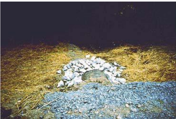
5-37 Rock rip-rap at pipe outlets spreads flow and dissipates energy.
