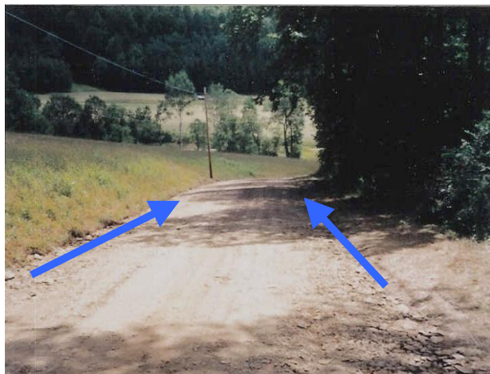
Before: The entrenched road trapped road drainage resulting in fast-moving concentrated ditchflow. This water eroded road material and deposited it directly into Pine Creek.
