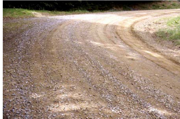
3-09 Banked (superelevated) curve.
