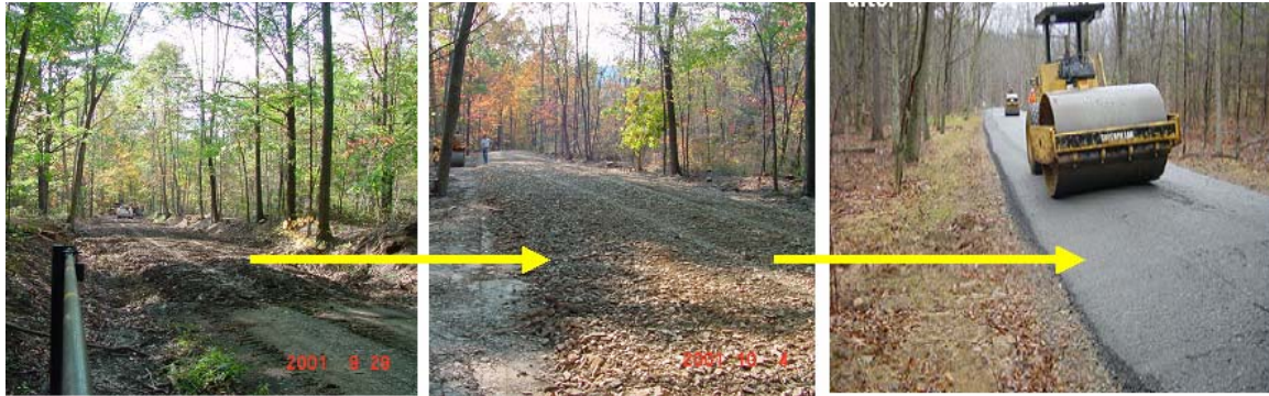
ESMP12-02 Raising the entrenched road—step-by-step.
