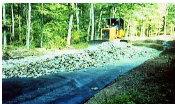
↑ Spreading the aggregate ↑
