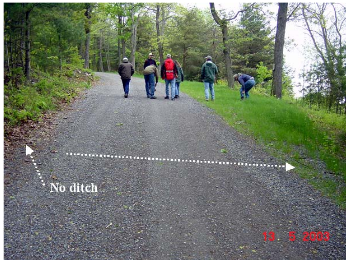
ESMP#2-01 Outsloped road showing no ditches and vegetative filtering areas for overland sheet flows.
