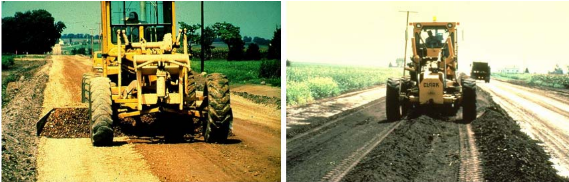
7-11 Stabilization can be accomplished with a road grader – scarifying the road, mixing in a stabilizing agent, regrading and shaping.
