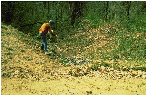
5-13 Seeding and mulching may be sufficient to revegetate the ditch.
