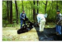
↑ Placing geocell ↑
