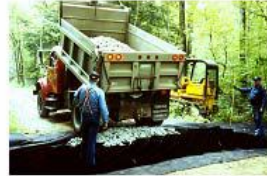
↑ Dumping aggregate fill ↑
