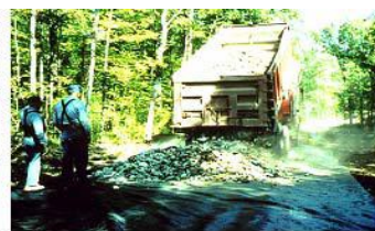
↑ Backdumping the aggregate ↑
