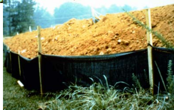
7-25 Geotextile silt fence barrier.
