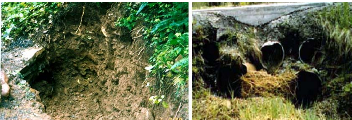
ESMP#7-01 Typical process of gouging out the roadside bank to install a cross pipe for ditch flow with no end structure leads to continual erosion and maintenance.
