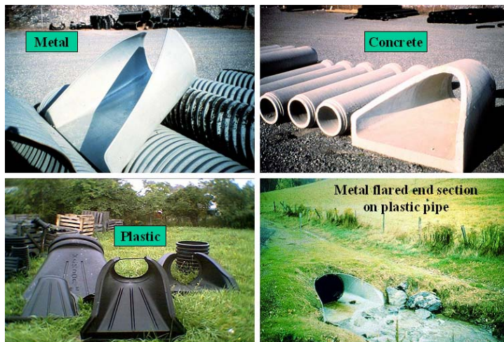
ESMP#8-03 Typical Flared End Sections.
