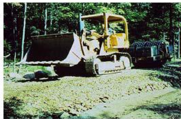
↑ Compacting the aggregate ↑
