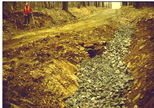
5-18 Riprap placed during construction—looking at the sediment potential, was this a good idea?
