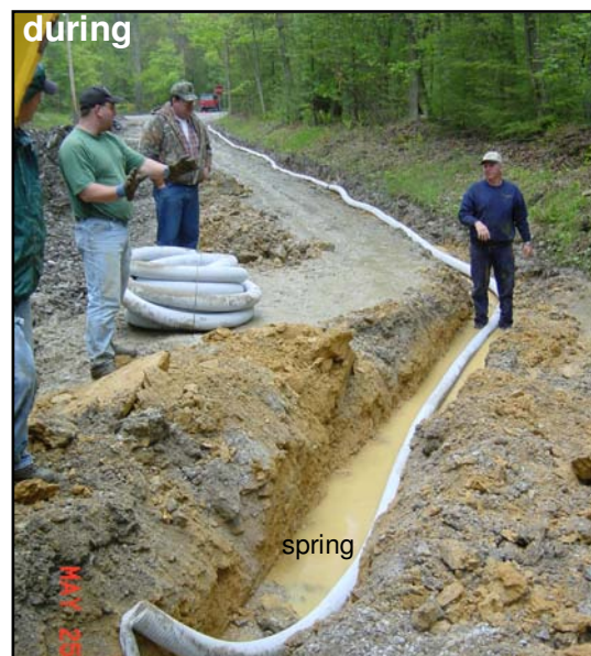
Photo 2. Pre-fabricated underdrain was used to collect subsurface water from under the road and both ditches.
