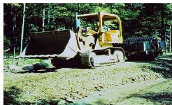
↑ Compacting the aggregate ↑
