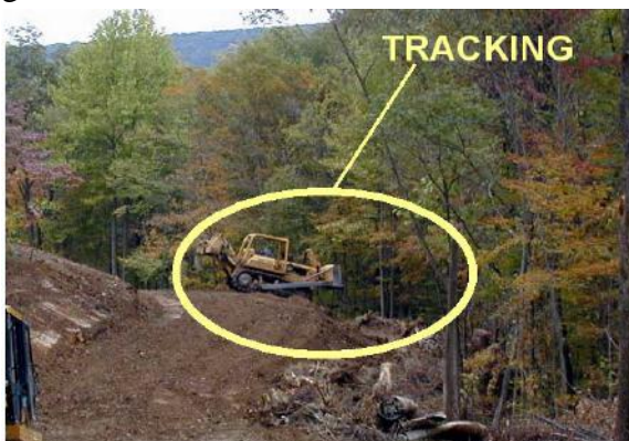
ESMP#13-03 Tracking newly constructed banks.
