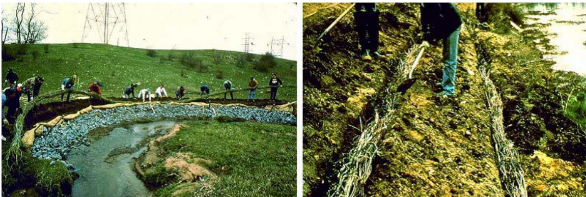
6.39 Placing the fascine and backfilling.
